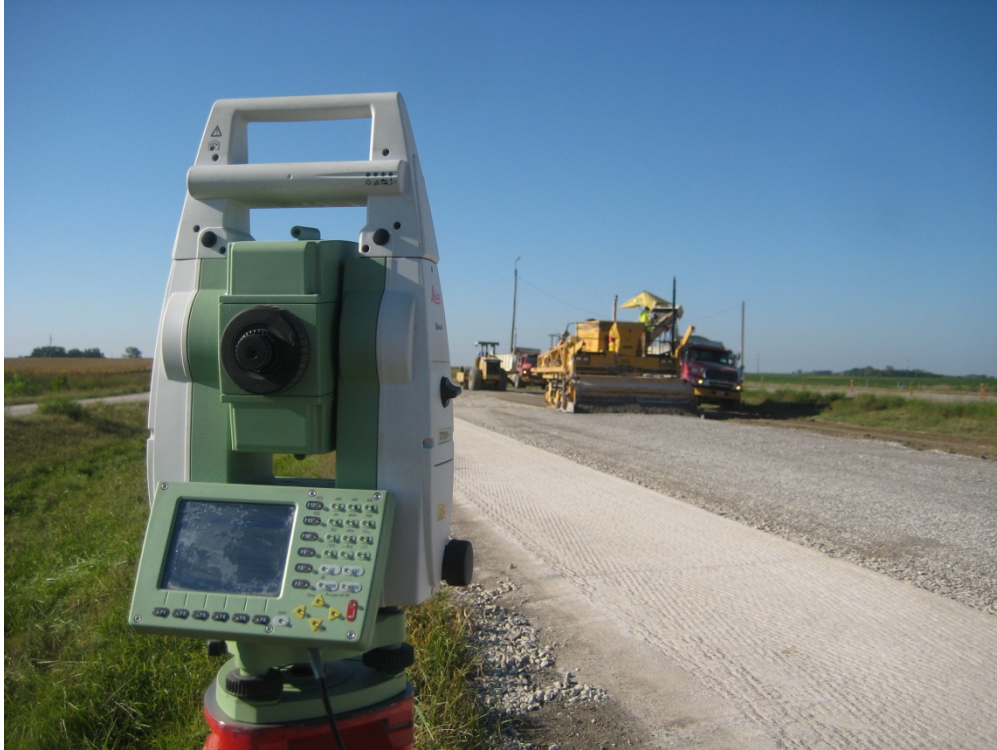
Figure 3. Total station for controlling leveling operations
