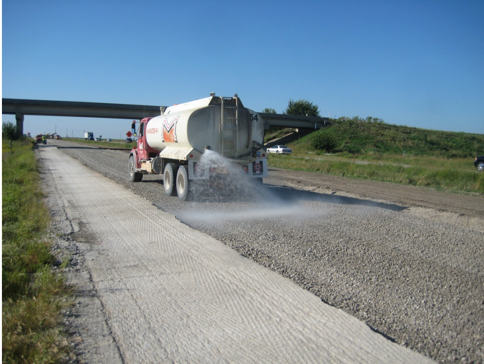
Figure 1. Moisture conditioning of aggregate after placement
