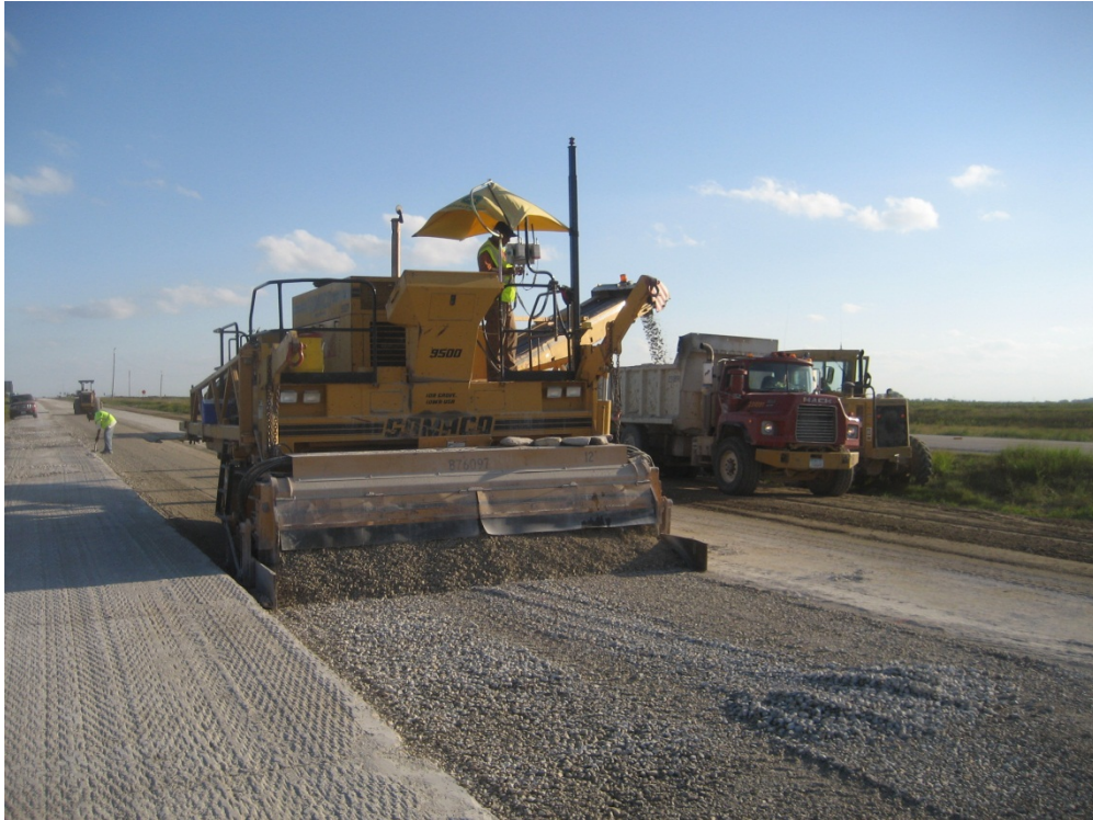
Figure 4. Open graded base layer trimming operations
