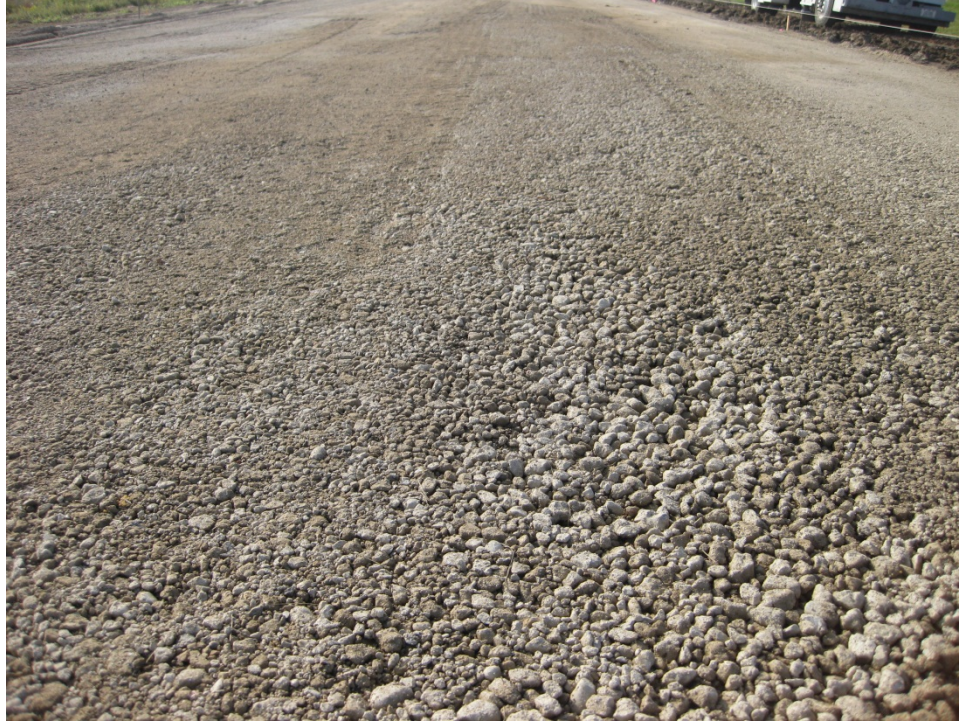
Figure 10. RPCC subbase layer after trimming
