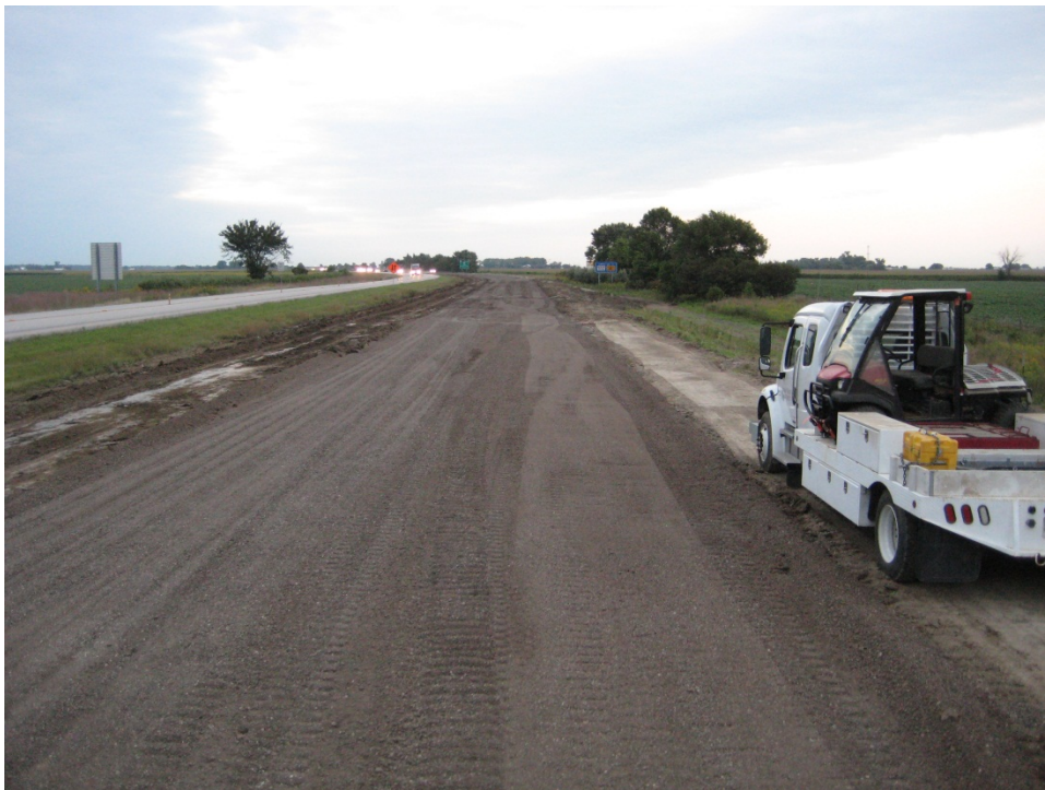
Figure 7. Compacted special backfill layer
