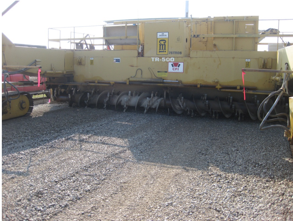
Figure 8. RPCC subbase layer trimming process
