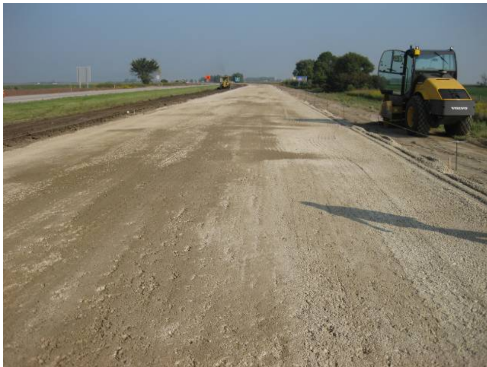
Figure 9. RPCC subbase layer before trimming
