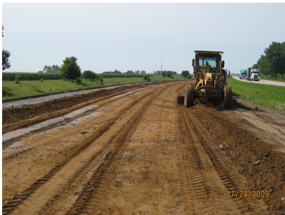
Figure 5. Blading existing subbase material down to subgrade
