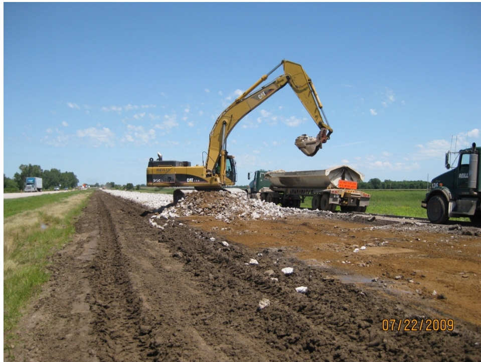
Figure 4. Removing existing CRCP
