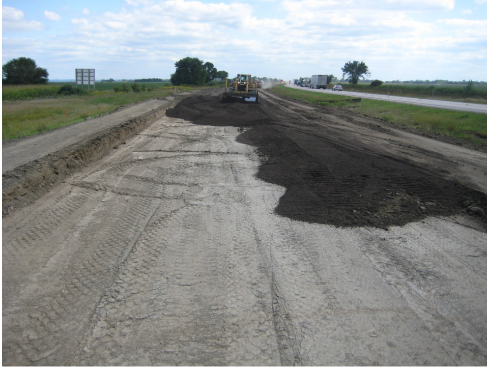
Figure 6. Spreading special backfill material over compacted subgrade
