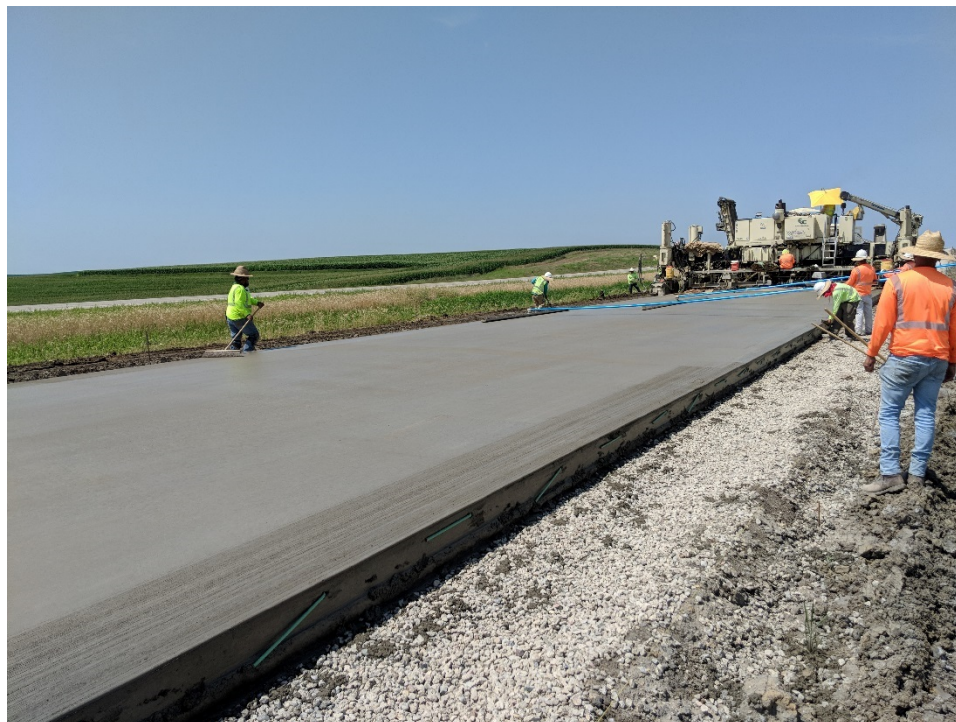
Figure 4: Cedar Valley Paving on US 20
