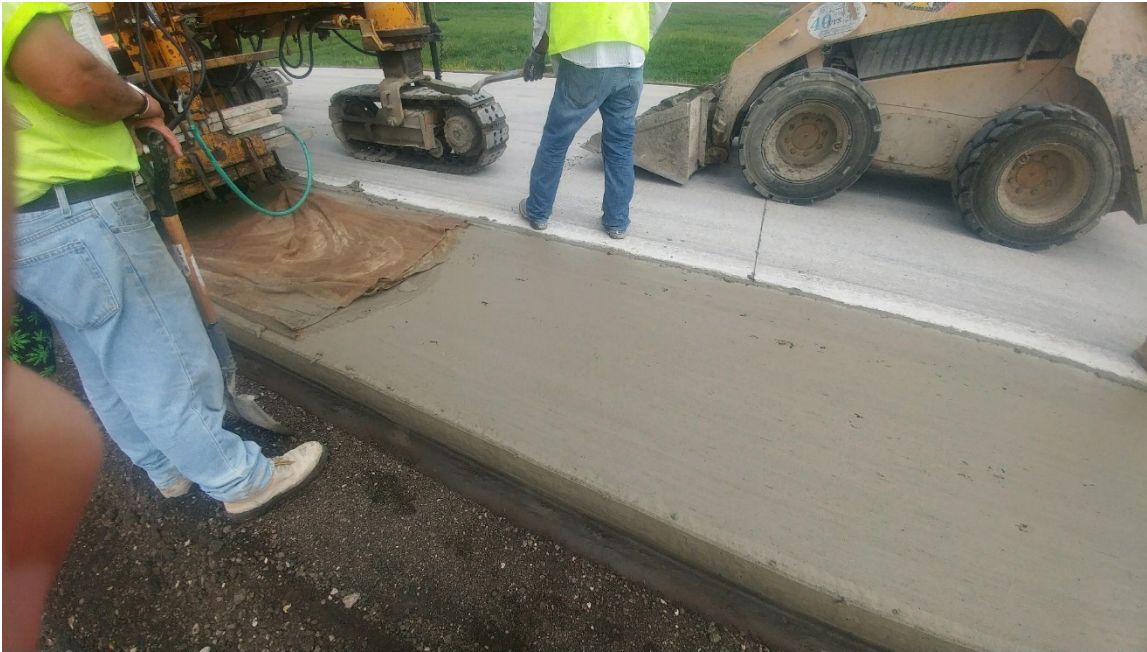
Figure 6: Paving with PEM Shoulder Mix
