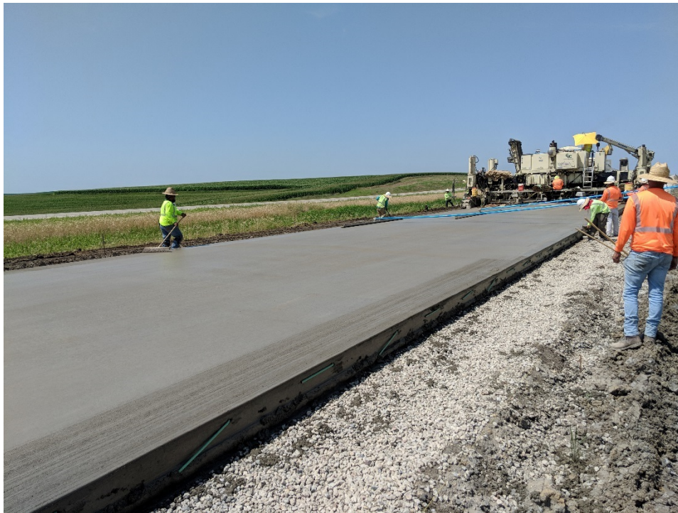
Figure 4: Cedar Valley Paving on US 20
