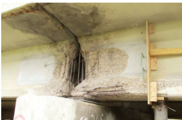
Severely deteriorated prestressed concrete beam ends in Minnesota
