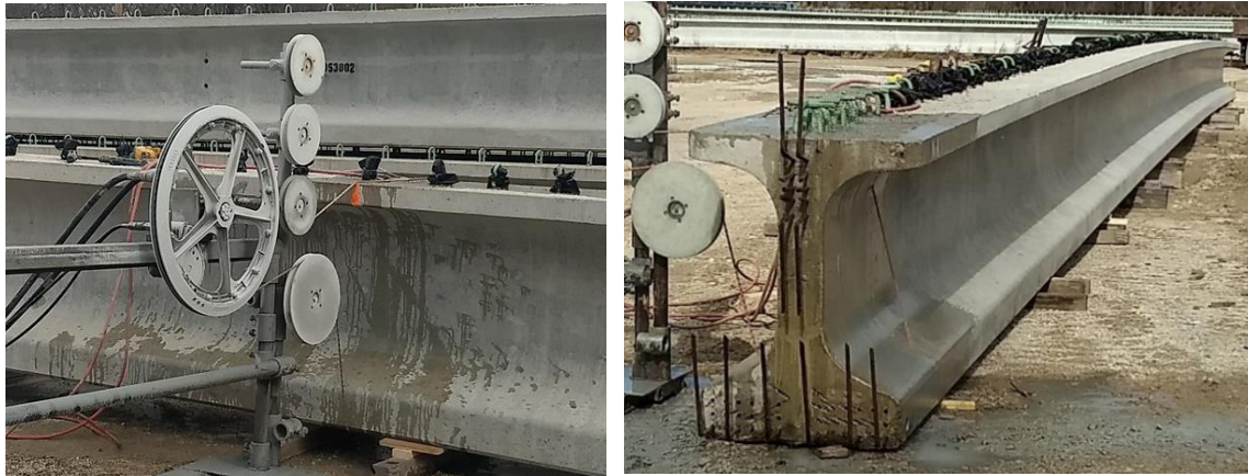
Figure 4.2. Wire saw cutting in progress
