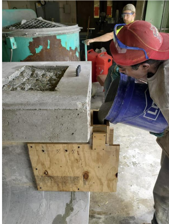
Figure 4.8. Patch mix being poured into formwork
