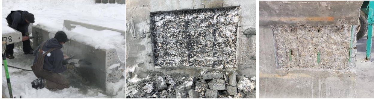
Figure 4.5. Cutting and chiseling (left), damaged bottom flange (center), and damaged web (right)
