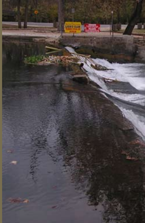
Recreational Makeover. Recreational chutes, pools, and boulders replaced a low-head dam, as hazard for innertubers in San Marcos, Texas. The area remains popular for innertubing, with added swimming and kayaking opportunities.
