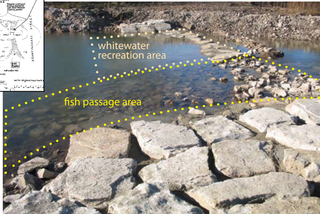
Figure 4-j. Iowa Code 481A.14 requires new in-channel structures to provide fish passage. Fish passage is a key for both muskels and fish to access various portions of streams. The roughened, gently sloping portion of the channel at the Charles City whiteater park is designed to maintain velocities and flow patterns fish can use to work up the rapids.
