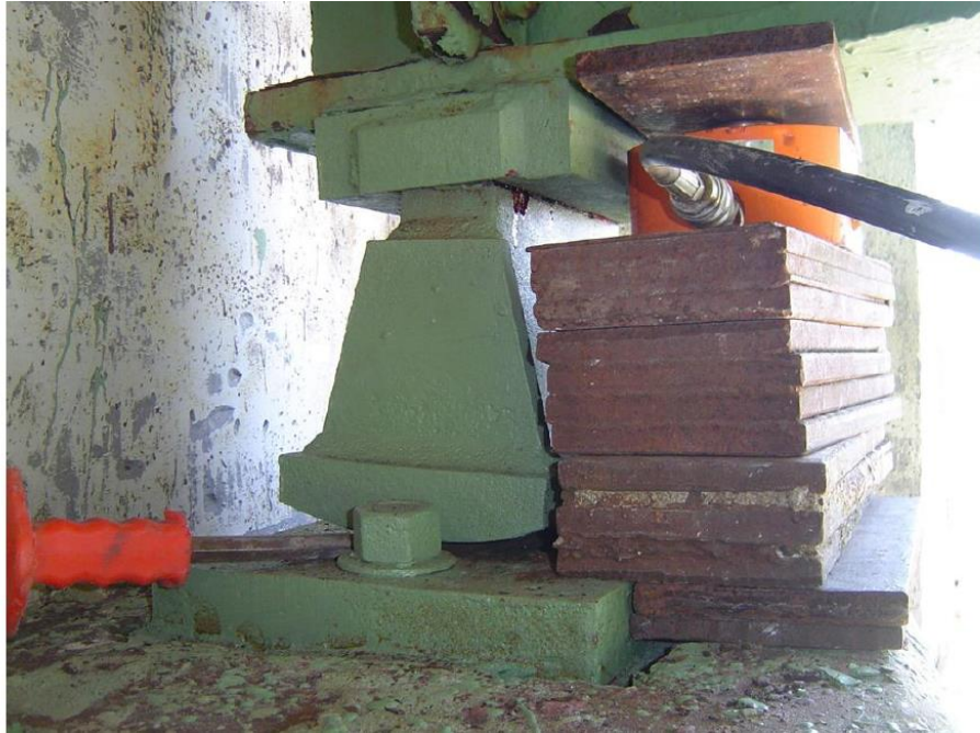
Figure 2.10. Typical bridge jacking to grease bearings
