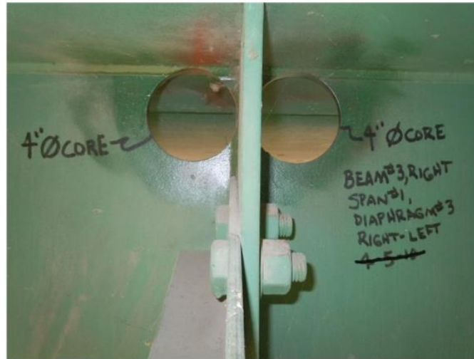
Figure 2.5. Arrest holes drilled in diaphragm stiffener
