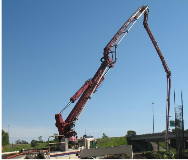
Figure 5.10. Pouring concrete using pump (left) and compaction using vibrator (right)
