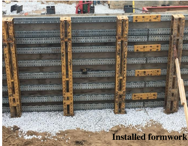
Figure 5.6. Formwork used in Pier 4 footing
