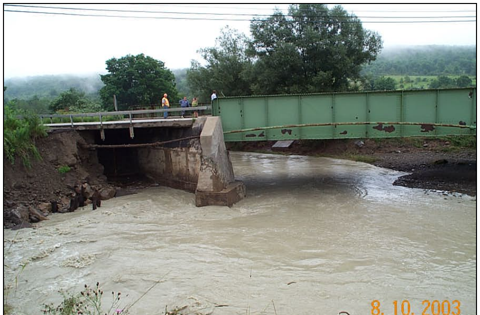
Waterway scour threatens bridge abutment and embankment.
