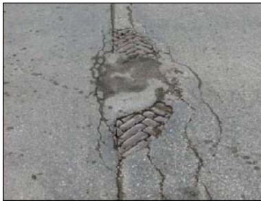
Asphalt Surface with Exposed Brick
