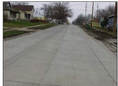
Completed Jointing Pattern
