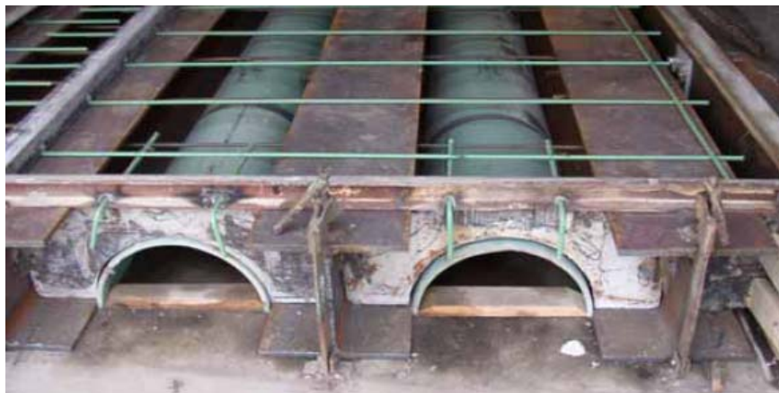
Transverse arches between the steel beams.
