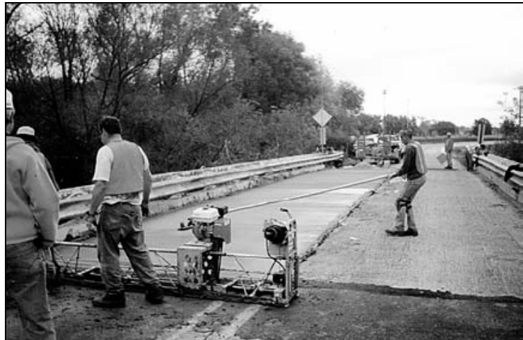
PCC Placement on the Independence Bridge
