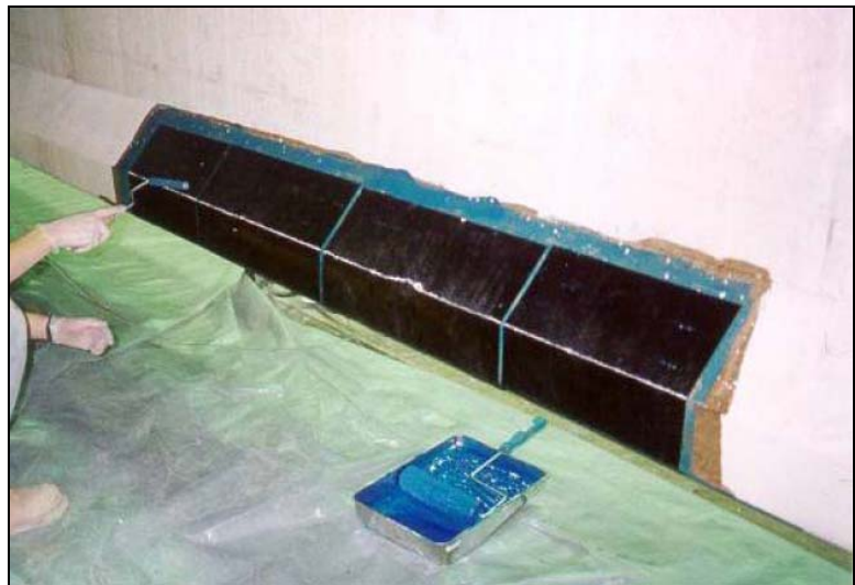
Installation of transverse CFRP jacket on Beam
