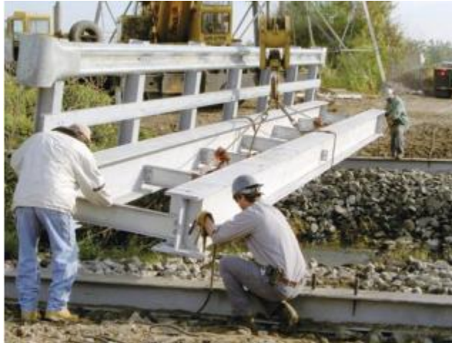
Figure 6. Construction of a one-lane bridge built with helical piles as the abutment foundation
