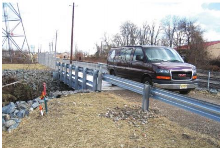
Figure 7. The completed one-lane bridge built with helical piles as the abutment foundation
