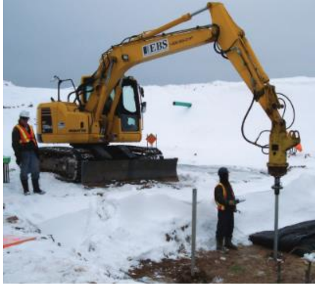
Figure 5. Installation of a helical pile
