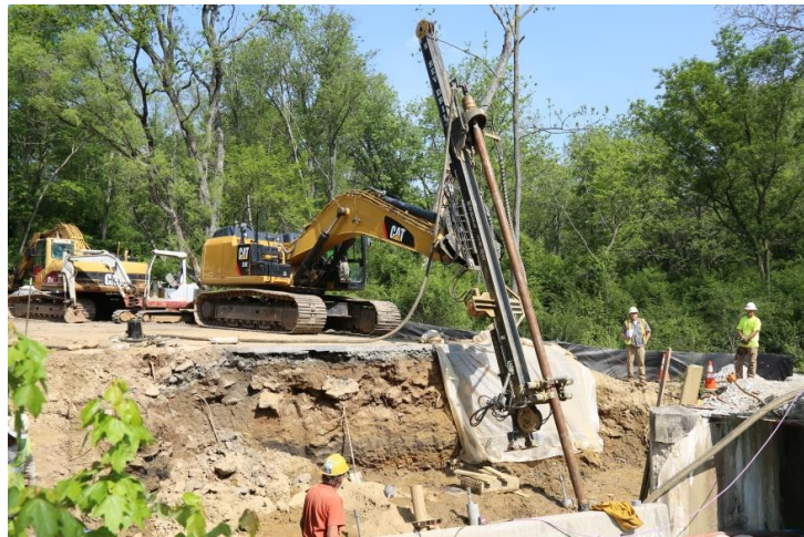
Figure 2. Setup for installing micropiles on Ensor Road bridge over Third Mine Branch
