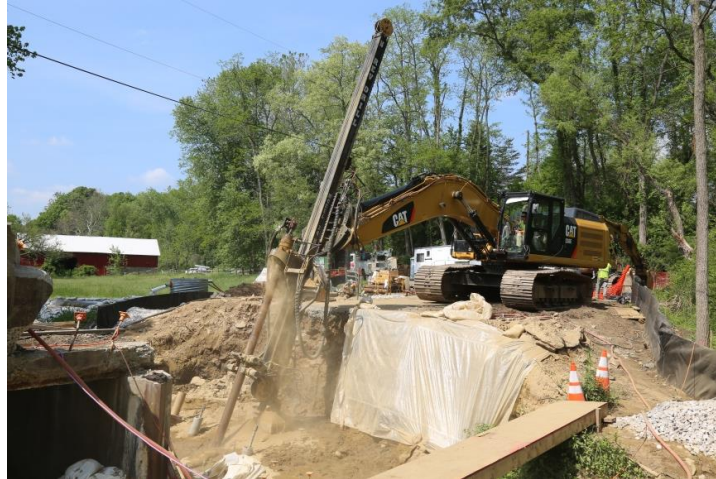
Figure 3. Micropiles being installed on Ensor Road bridge over Third Mine Branch
