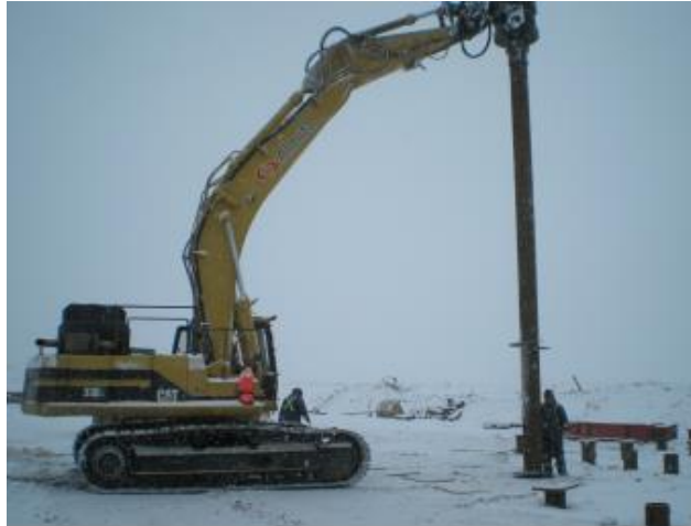
Figure 4. Large helical pile installation
