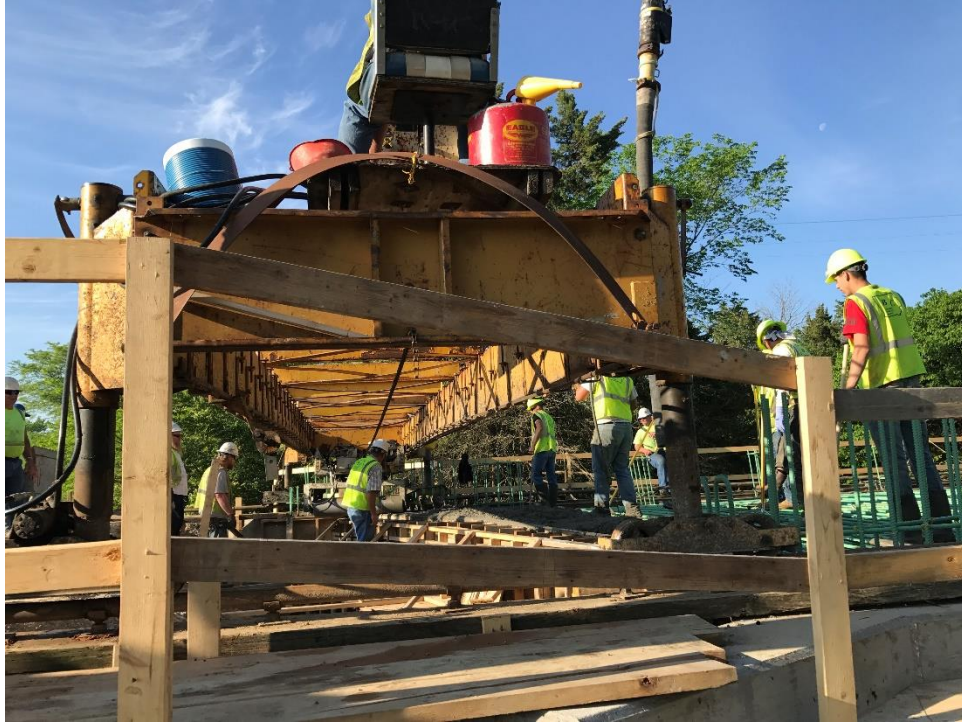
Figure 13. Cedar Fork Bridge screed orientation relative to deck skew
