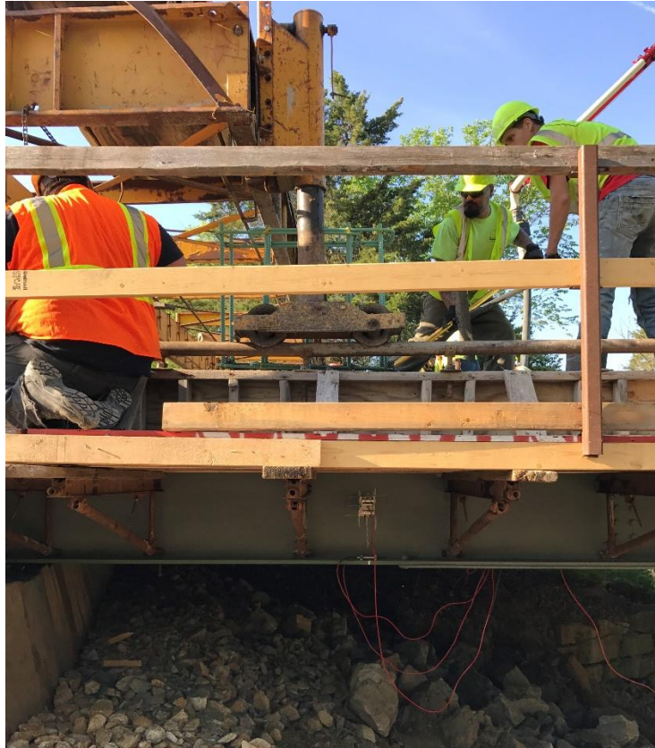
Figure 14. Screed traveling over an instrumented cross-sectional location of the Cedar Fork Bridge
