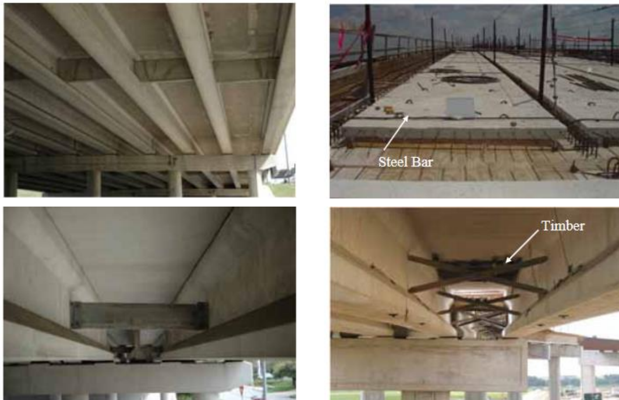
Figure 8. Bracing examples: concrete diaphragms (top left), top bracing bars (top right), steel diaphragms (bottom left), and timber blocking (bottom right)
