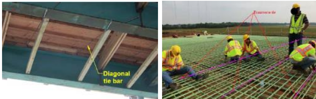
Figure 9. Diagonal tie bar connected from exterior girder to first interior girder (left) and transverse tie bars connected from exterior girder to exterior girder (right)
