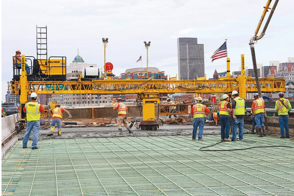
Figure 2. Finishing screed for deck construction
