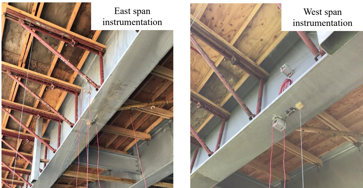
Figure 26. Maple Bridge instrumentation for the east (left) and west (right) spans during the braced deck pour
