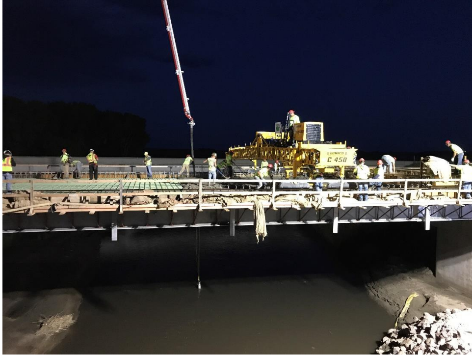
Figure 20. Screed orientation for the Maple Bridge
