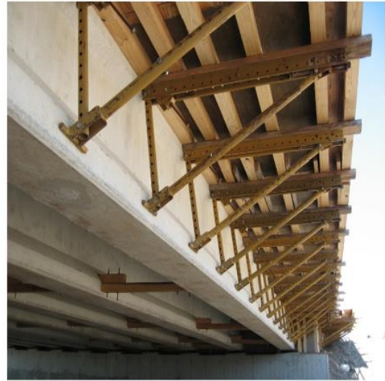
Figure 1. Typical overhang formwork schematic (left) and in-field example (right)
