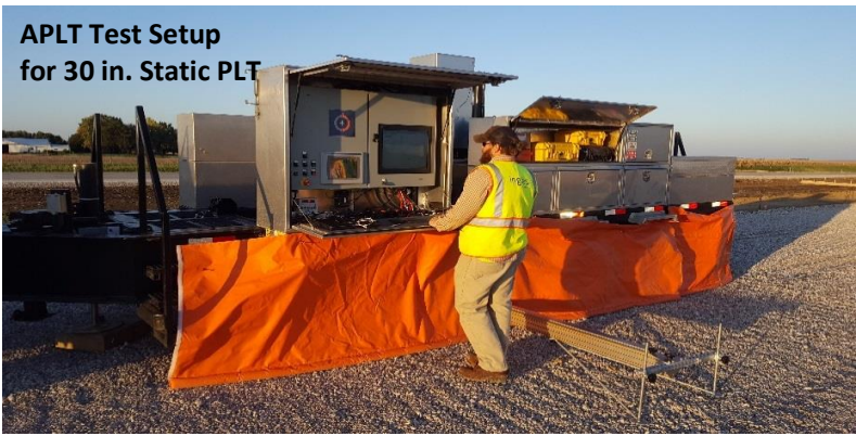
30 in. Static Plate Load Testing
