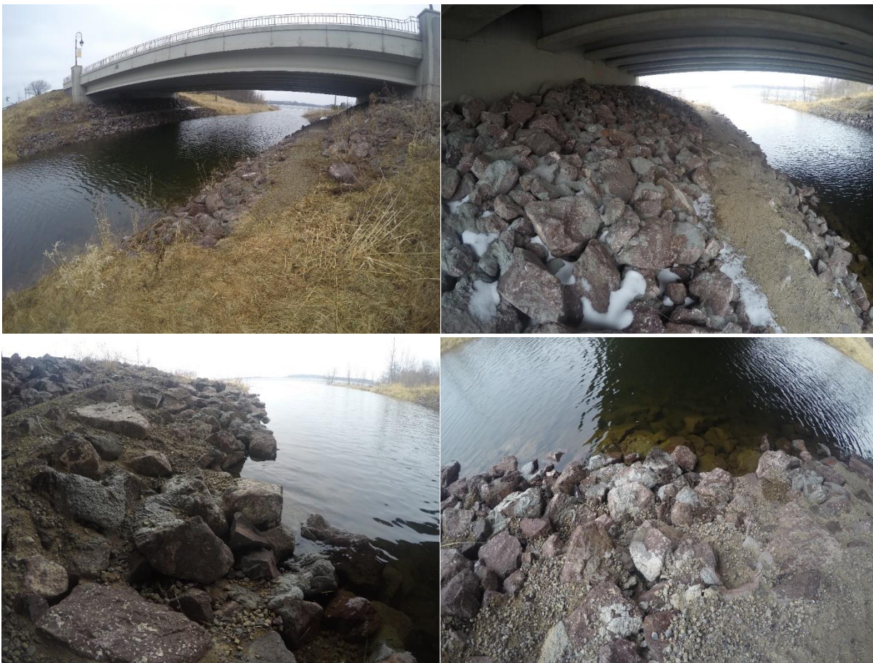
Figure 17. Minnesota Site 2: Partially grouted riprap
