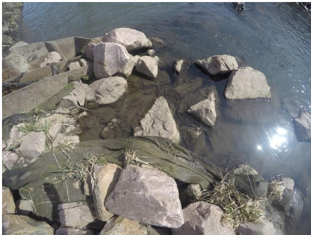
Figure 25. Failing stream grade control in Woodbury County, Iowa
