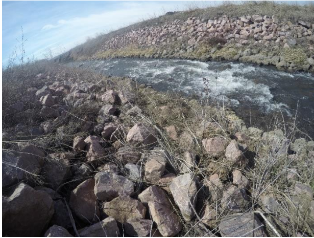
Figure 24. Partially grouted riprap in Woodbury County, Iowa
