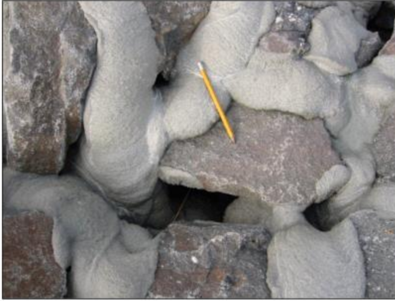
Figure 7. Partially grouted riprap
