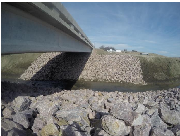
Figure 23. Recently completed, loose riprap in good condition in Woodbury County, Iowa
