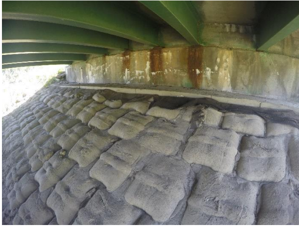
Figure 27. Grout-filled blankets in Buchanan County, Iowa
