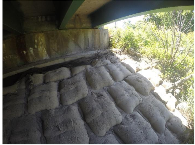
Figure 27. Grout-filled blankets in Buchanan County, Iowa
