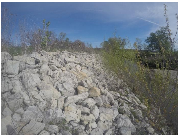
Figure 29. Loose riprap during low water levels in Madison County, Iowa
