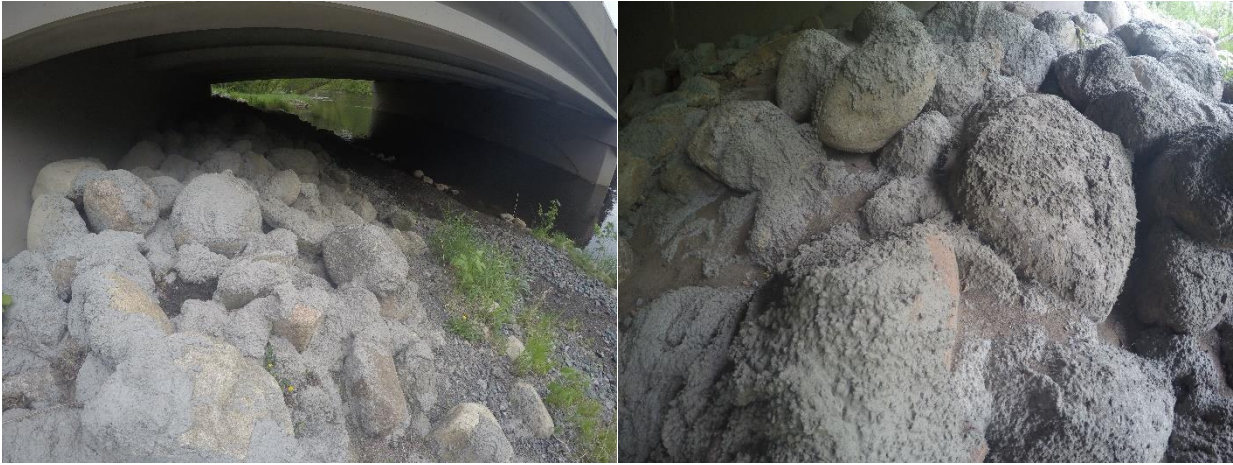
Figure 19. Minnesota Site 4: Partially grouted riprap-splash of grout
