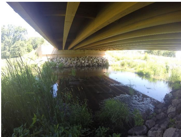
Figure 26. Loose riprap in Buchanan County, Iowa
