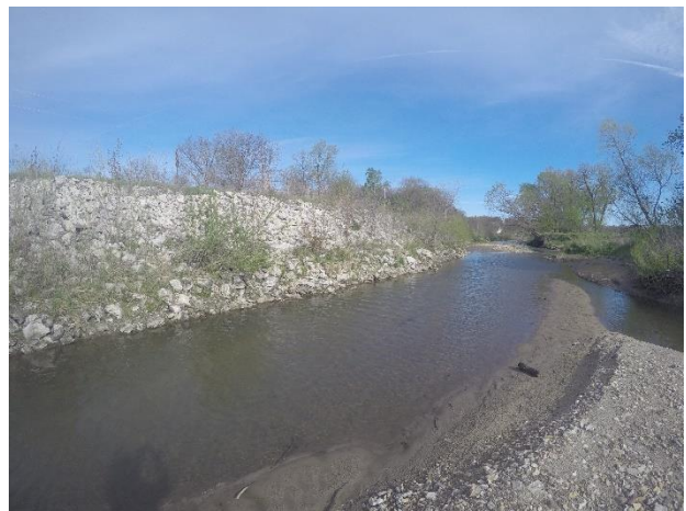
Figure 29. Loose riprap during low water levels in Madison County, Iowa
