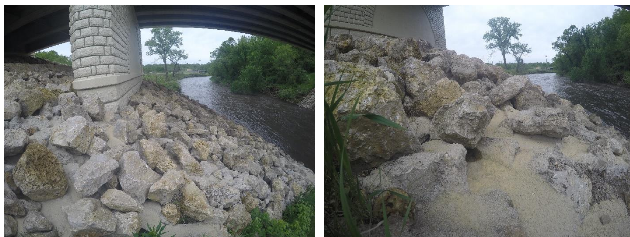
Figure 18. Minnesota Site 3: Partially grouted riprap-thin grout
