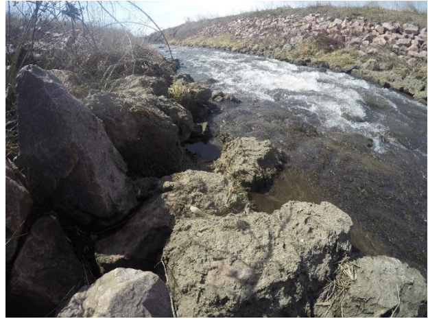
Figure 24. Partially grouted riprap in Woodbury County, Iowa
