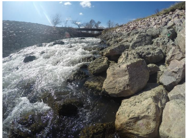
Figure 22. Grouted and loose riprap in Woodbury County, Iowa
