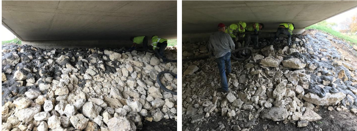
Figure 33. Grouting of Class E revetment (left) and shotrock (right) used for Bridge 1 in Buchanan County
