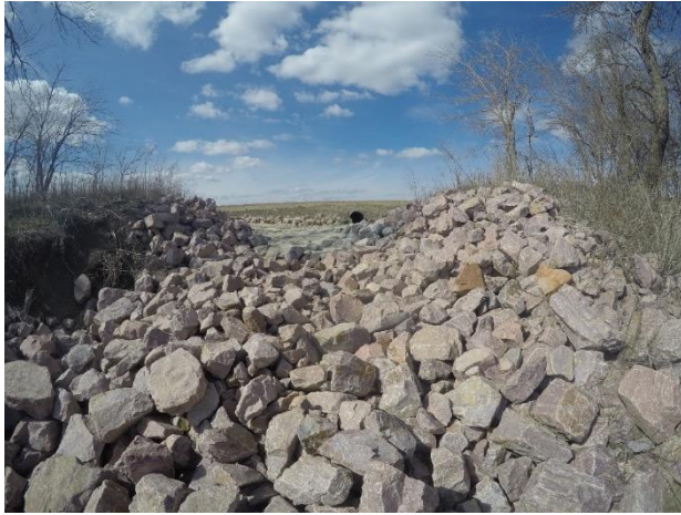
Figure 21. Loose riprap with some grouting in Woodbury County, Iowa
