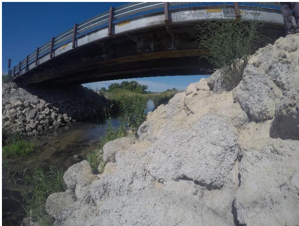
Figure 28. Grouted riprap in Buchanan County, Iowa
