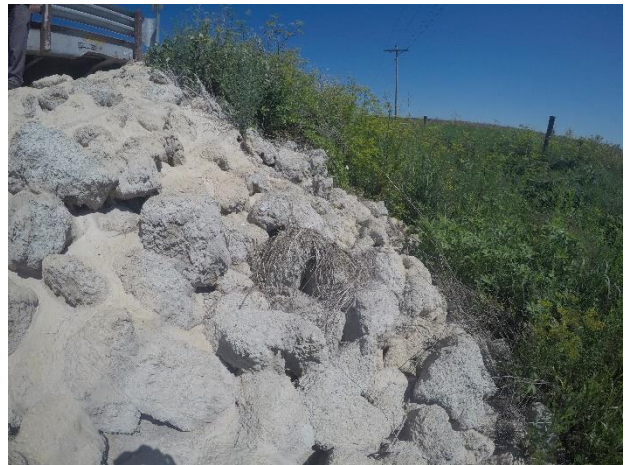
Figure 28. Grouted riprap in Buchanan County, Iowa
