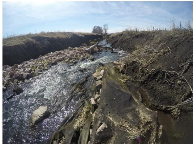
Figure 25. Failing stream grade control in Woodbury County, Iowa
