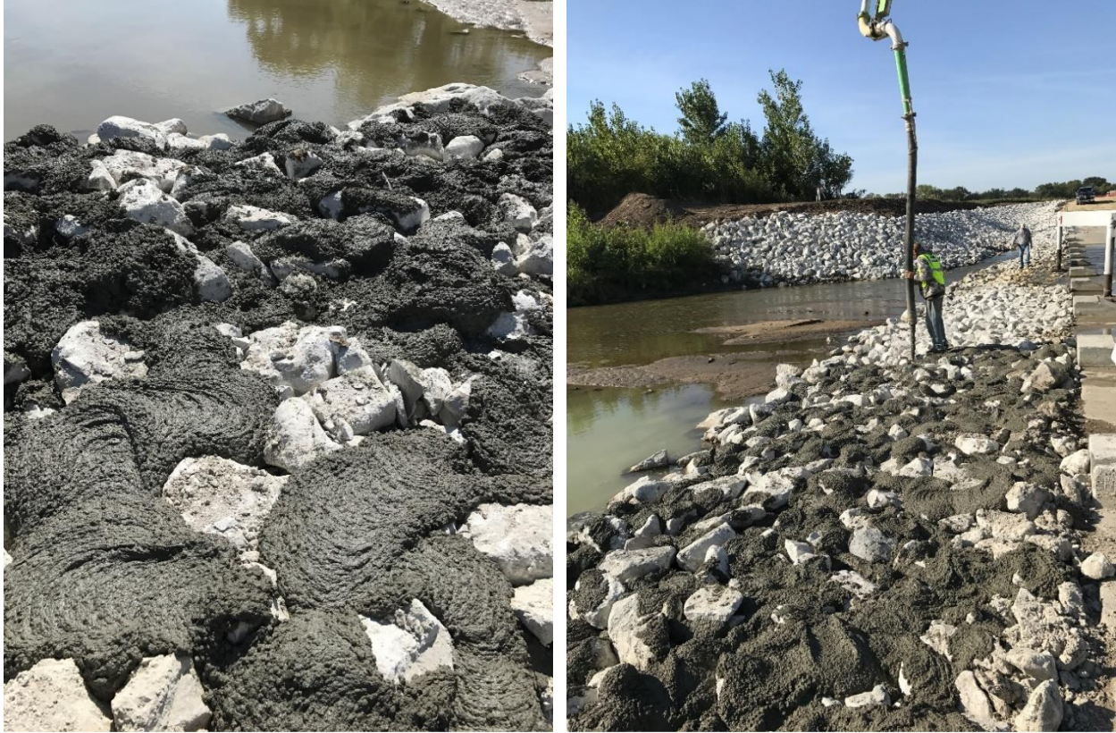
Figure 38. Madison County pilot installation grouting
