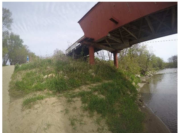
Figure 32. Loose riprap, many washed away stones in Madison County, Iowa
