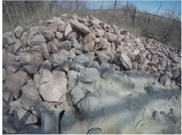
Figure 21. Loose riprap with some grouting in Woodbury County, Iowa
