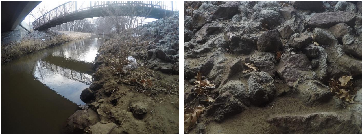
Figure 16. Minnesota Site 1: Partially grouted riprap
