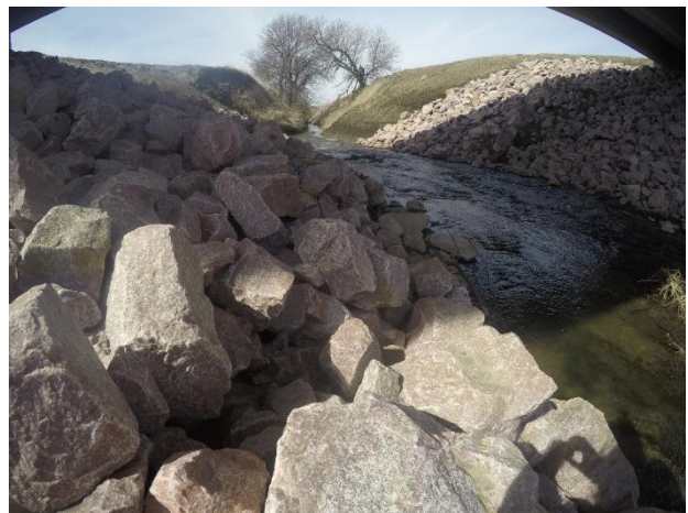
Figure 23. Recently completed, loose riprap in good condition in Woodbury County, Iowa
