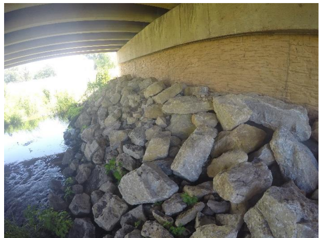
Figure 26. Loose riprap in Buchanan County, Iowa
