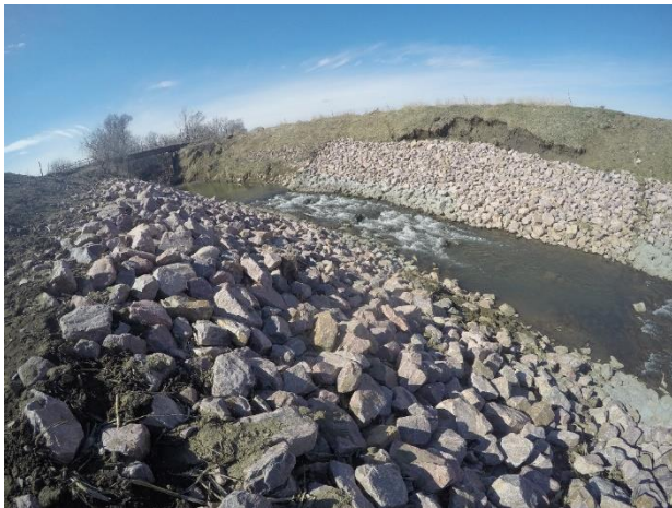
Figure 22. Grouted and loose riprap in Woodbury County, Iowa
