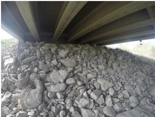
Figure 31. Loose riprap, undersized in Madison County, Iowa
