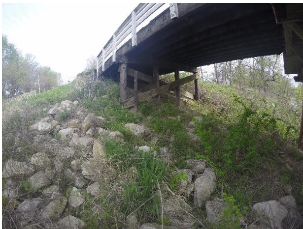
Figure 32. Loose riprap, many washed away stones in Madison County, Iowa
