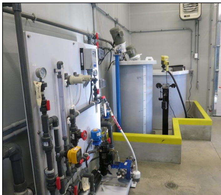
Chemical feed and feedstocks with containment
