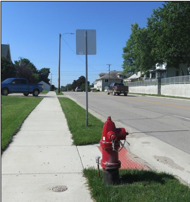
New hydrant as part of a water main replacement project
