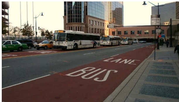
Figure 10. Red pavement treatment for bus lanes at Penn Station in Newark, New Jersey
