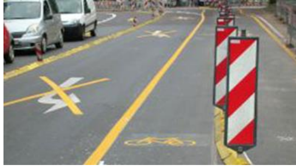
Figure 55. Special-color overriding existing urban street marking (Germany 2010)
