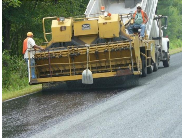
Figure 5. Chip seal application
