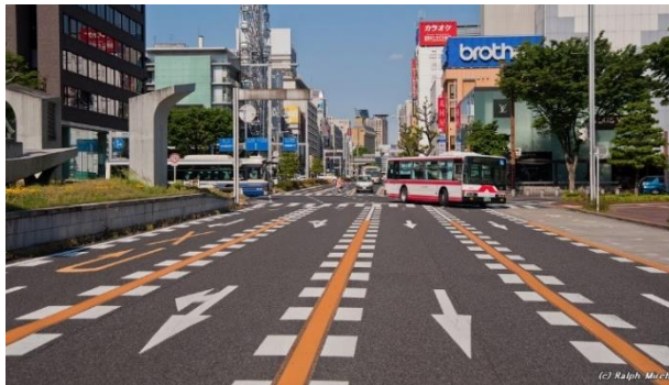
Figure 26. Permanent pavement markings on an urban arterial in Nagoya, Japan (2012)
