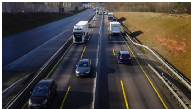
a. Yellow PM override the usual white markings at this highway work zone on the A9 Autobahn near Schnaittach, Germany (2003)
