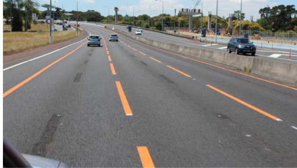
Figure 24. Orange marking trial and ghost markings on SH 16 Causeway Upgrade in Auckland, New Zealand
