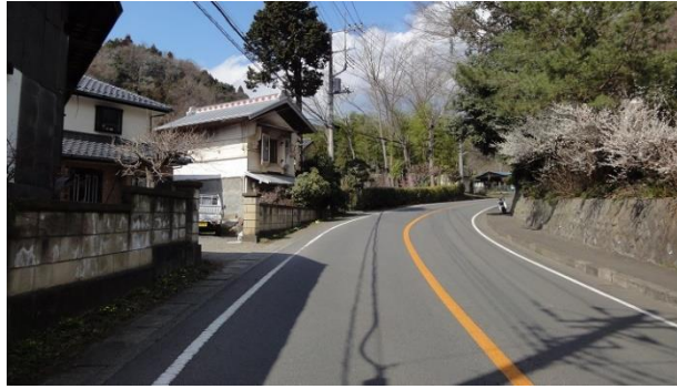
Figure 27. Comparison of yellow and orange no-passing zone markings in Japan
