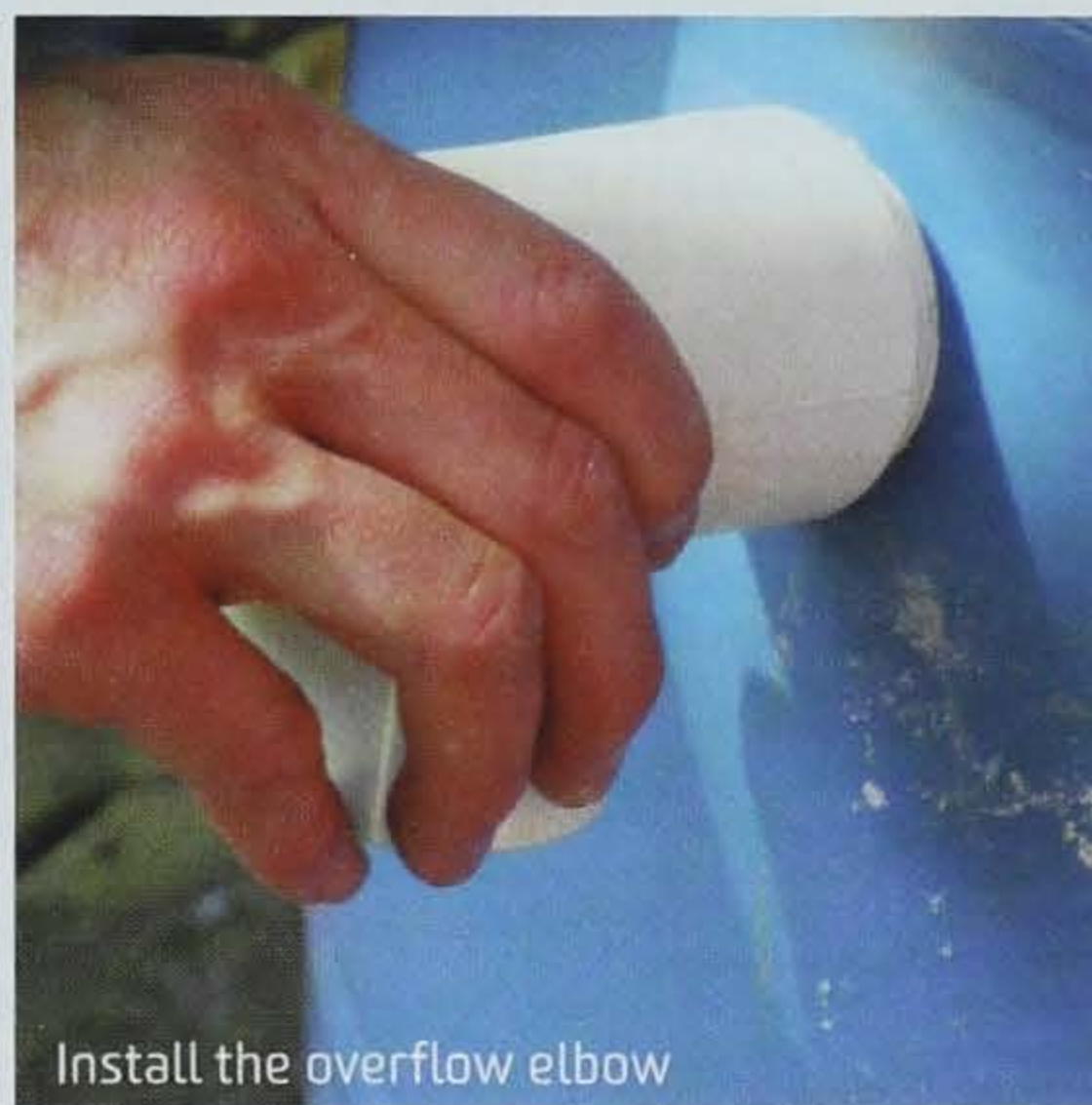
The PVC overflow pipe carries water away from foundations.
