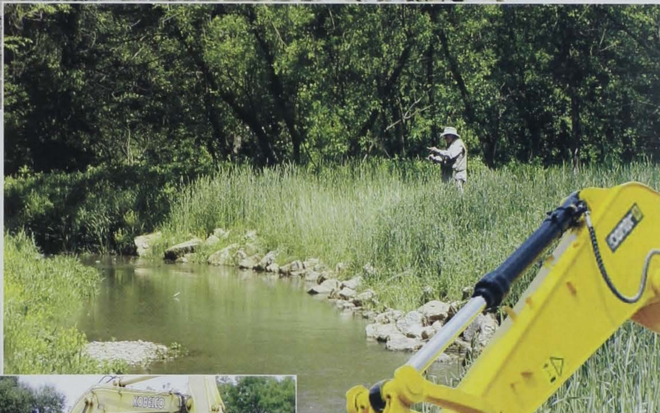
Roughly 4,700 feet of Catfish Creek's streambank were stabilized with rock riprap and 750 feet of bankhides were added, making the coldwater stream one of the more popular trout destinations in the state.
