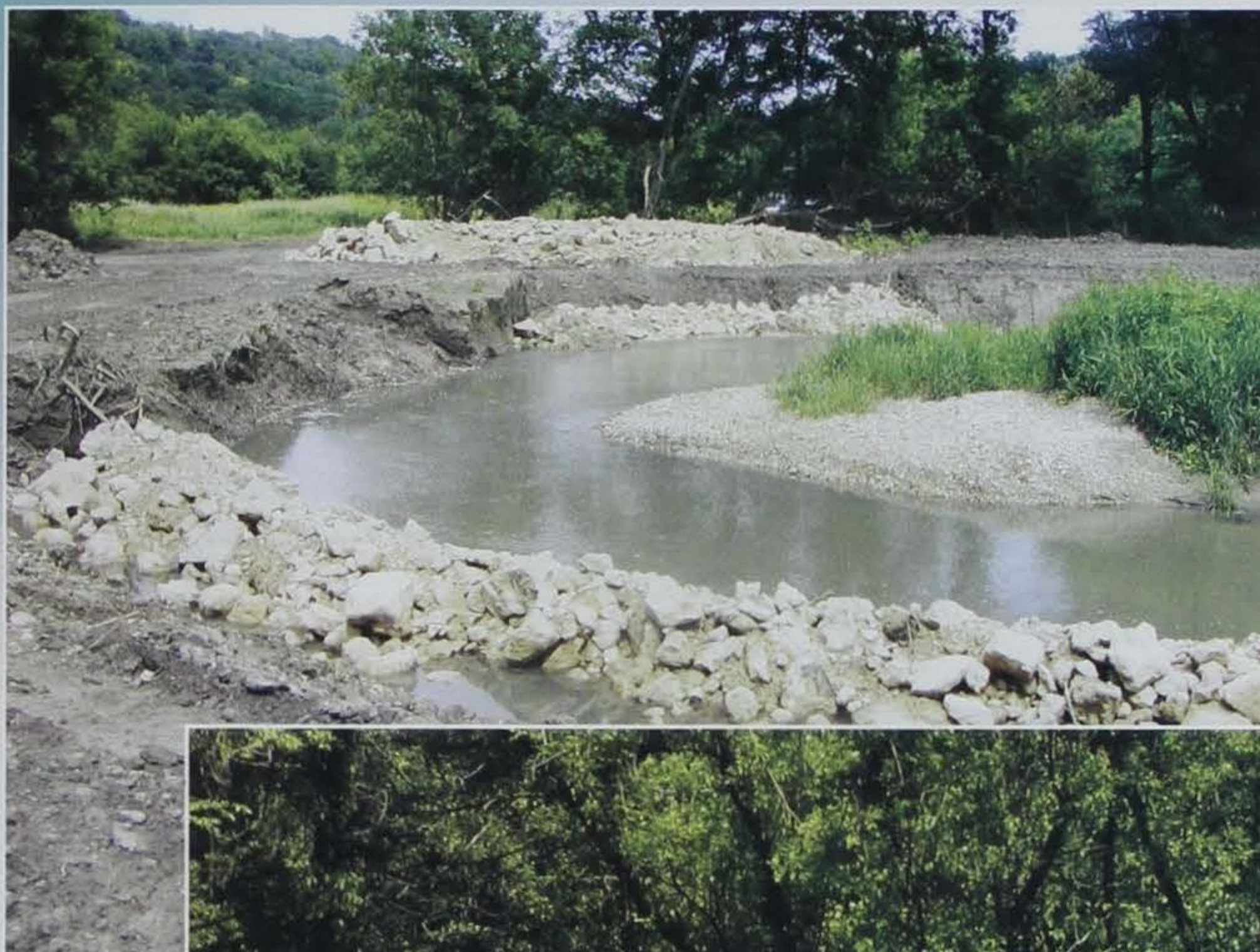
Roughly 4,700 feet of Catfish Creek's streambank were stabilized with rock riprap and 750 feet of bankhides were added, making the coldwater stream one of the more popular trout destinations in the state.
