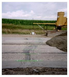
Figure 8. Tied Transverse Crack
