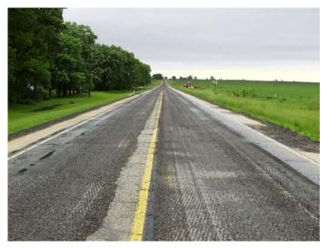
Figure 5. Scarified Pavement Surface
