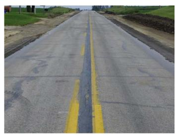
Figure 6. Completed Milling Operation
