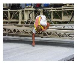
Figure A.2. Iowa Maturity Device Installation
