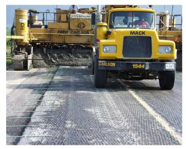
Figure 10. Stapled #4 Bar that Ties the Widening Unit to the Thin Overlay
