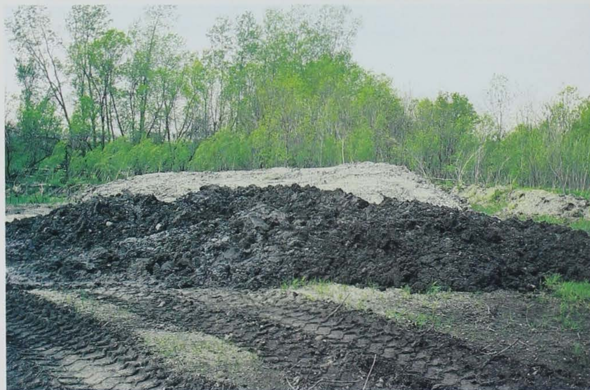
The contaminated soil was stacked nearby to dry before going to the landfill.
