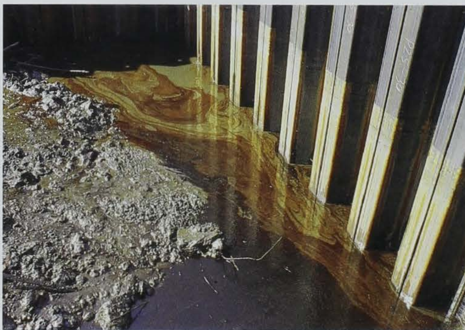
The product swirls around on top of the water after the backhoe digs into the riverbank. There is a strong smell of diesel fuel.
