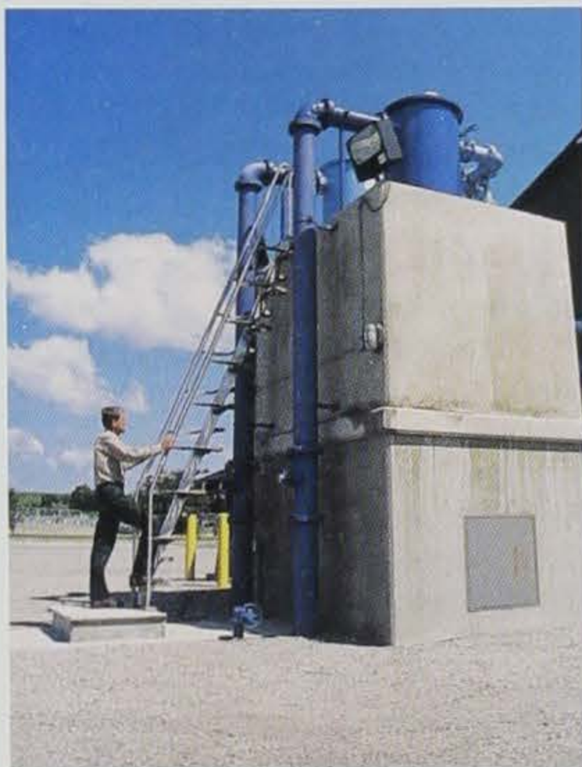
The aeration/degassing head tank is used to add oxygen to water flowing to the outside raceways and tanks located inside the building.
