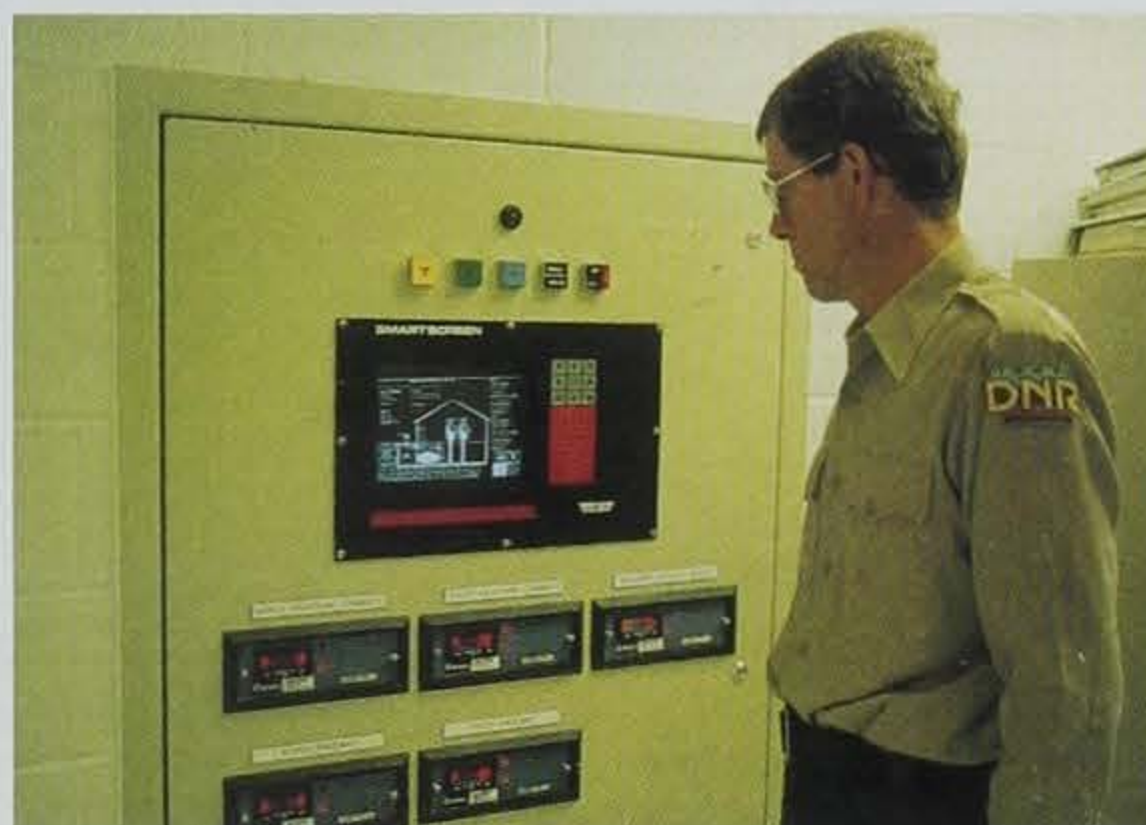
Disease diagnosis is routinely performed in the combination laboratory/office located inside the research building (left). The computerized "smartscreen" located inside the laboratory/office, monitors the condition of the equipment and water quality and alerts personnel to alarm situations.
