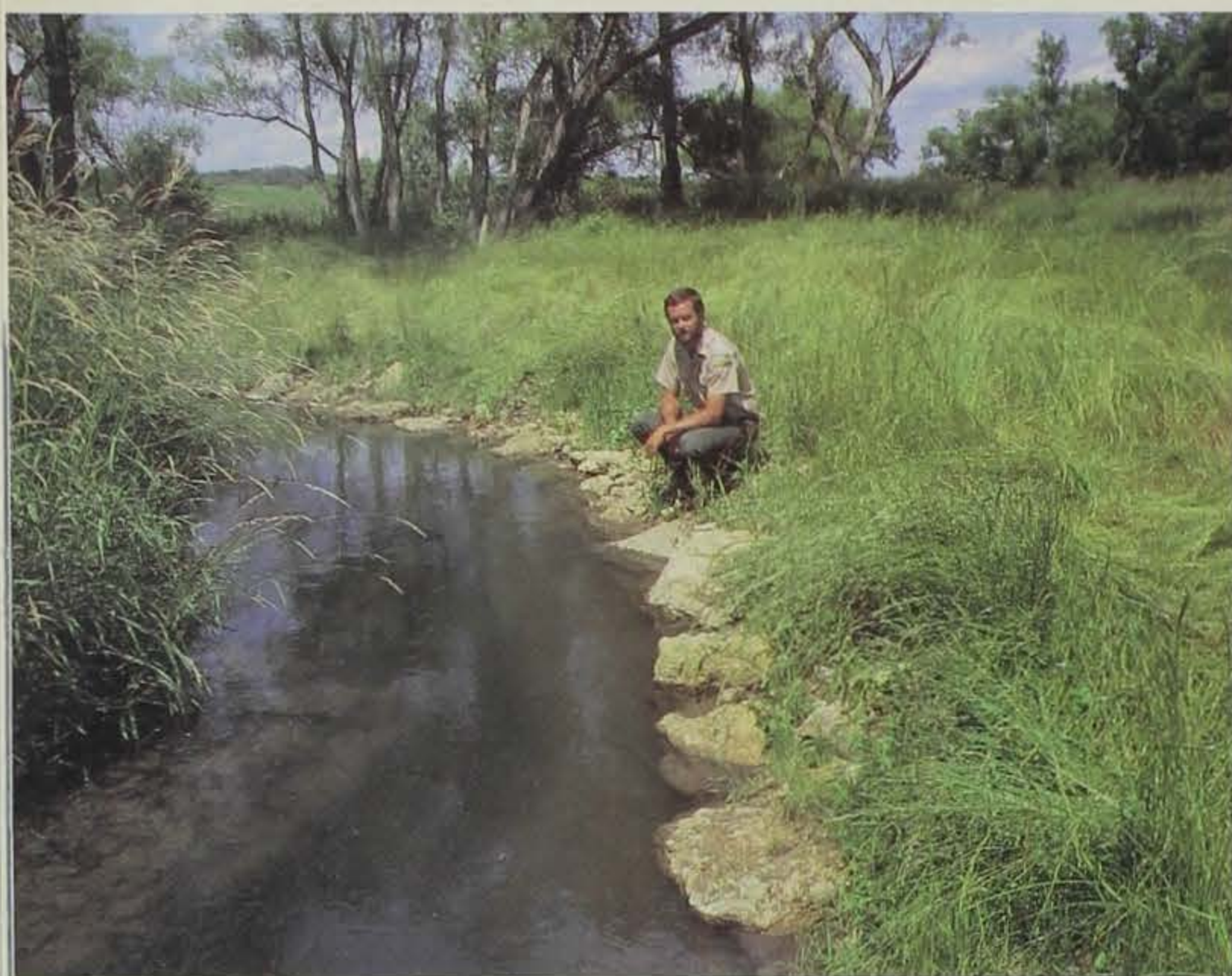
▲ Bill Kalishek on top of a bank hide at the Ensign Hollow project in Clayton County. Riprap and long-stemmed native prairie grasses were used to shelter the stream.
