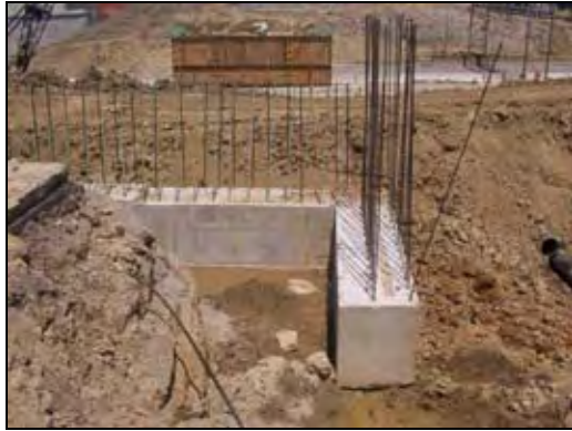
(a) Backwall construction
