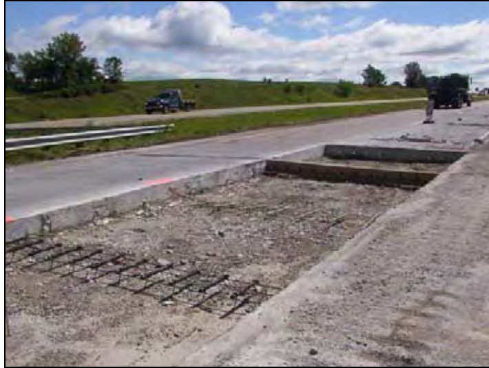
Figure 133. Replacing the bridge approach slab section
