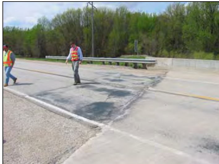
Figure 84. Cracking of asphalt overlay (East end)
