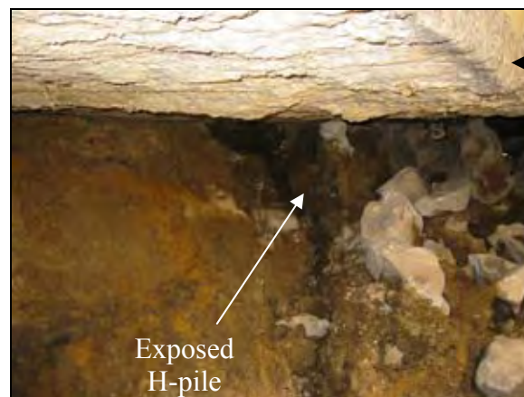
Figure 122. Exposed H-pile (side view)
