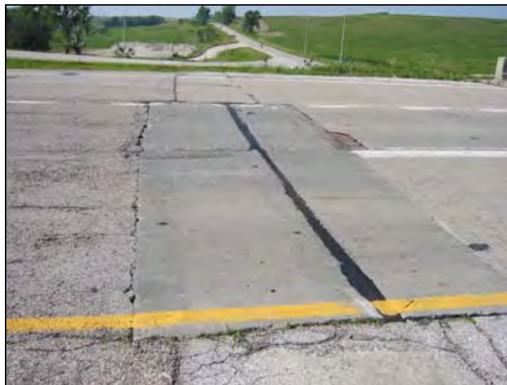
Figure 119. Various cracking at the bridge approach (EBL)
