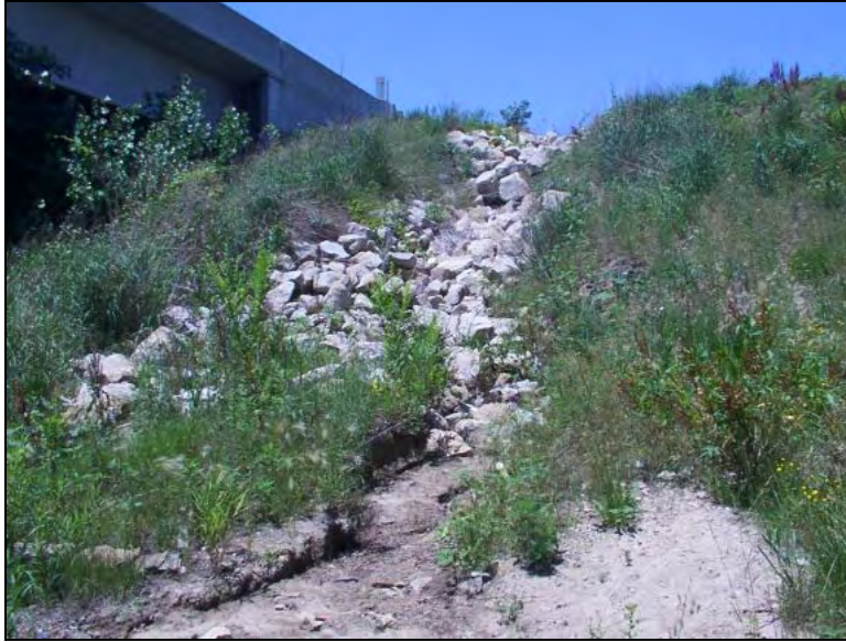
Figure 250. Rocks placed at the abutment side to prevent erosion (North end of NBL)
