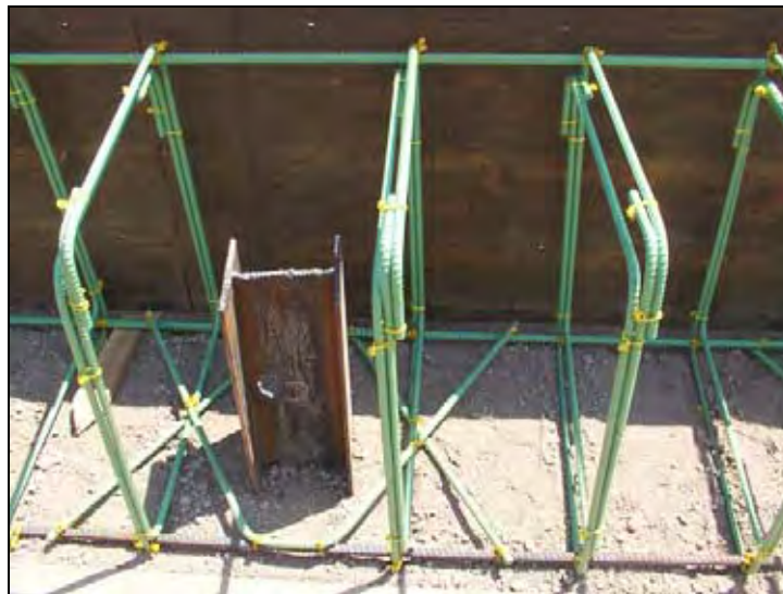
Figure 225. H-pile embedded in the bridge backwall
