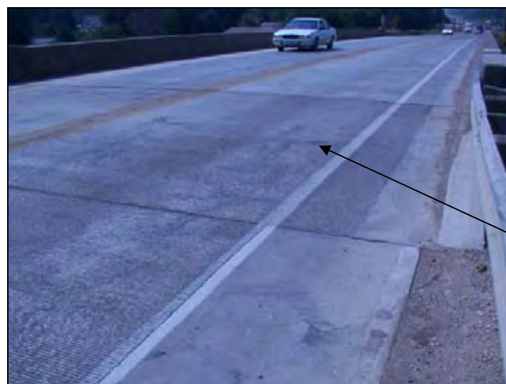
Figure 145. Differential settlement at recently replaced bridge approach
