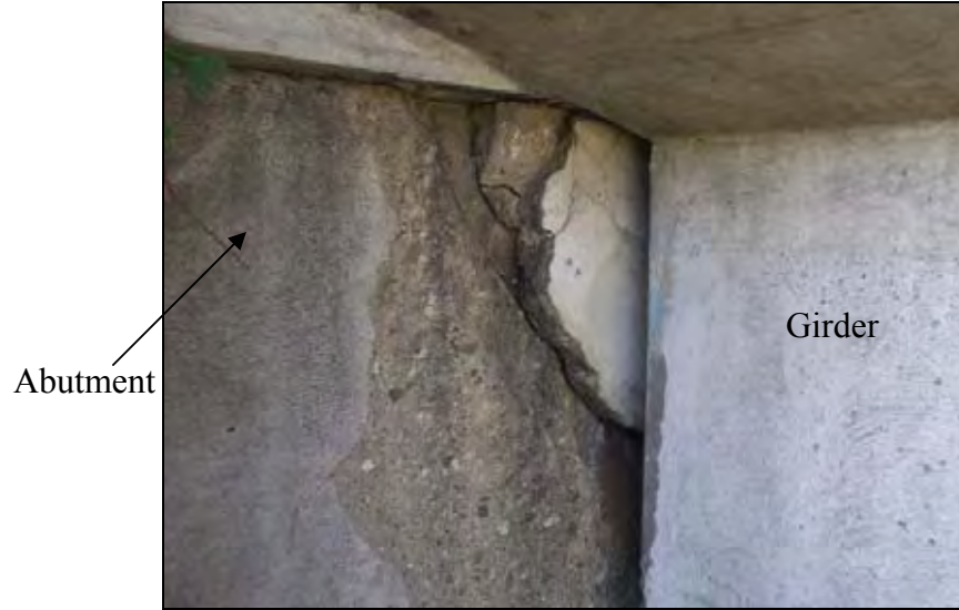
Figure 194. Concrete spalling at the abutment (SBL)
