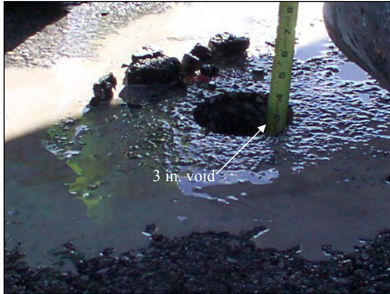
Figure 283. A 3-inch-void under the approach slab estimated by measuring the distance the core dropped (North end of SBL, edge line)
