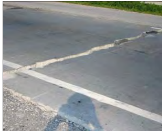
(b) Closer image of faulted approach slab
