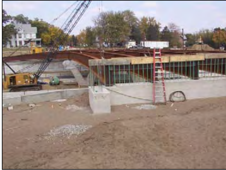
Figure 209. Construction of steel girders and backwall
