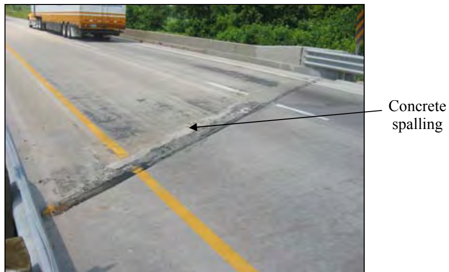
Figure 128. Concrete spalling at the expansion joint
