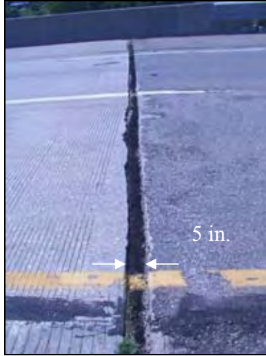
Figure 302. Recycled tires used as joint filler
