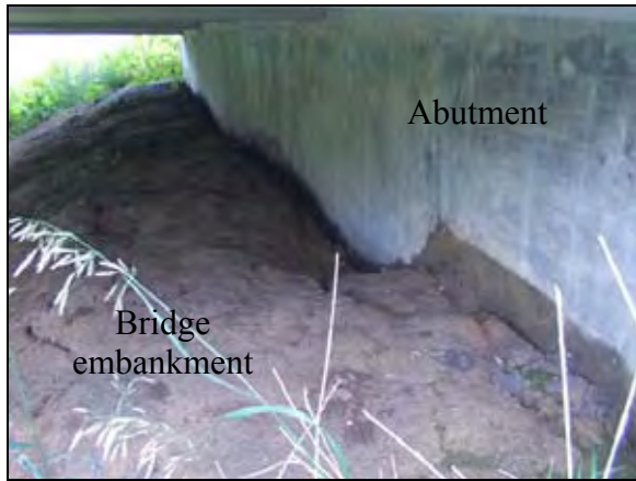
(a) Erosion at the abutment
