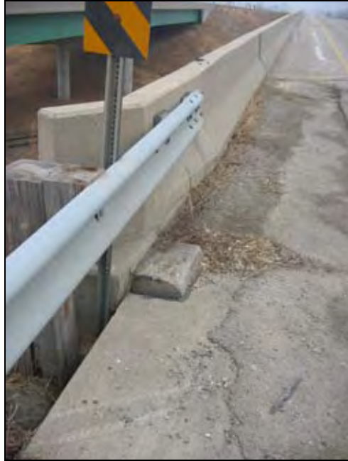
Figure A3. Differential settlement
