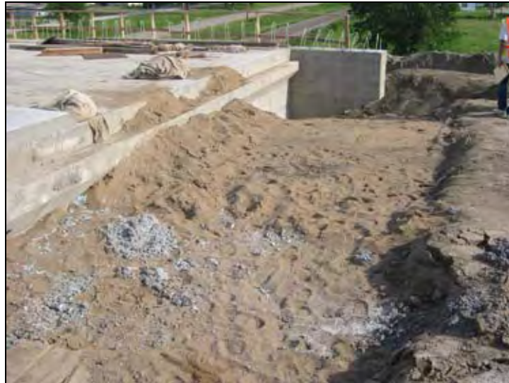
Figure 230. Poorly placed granular backfill
