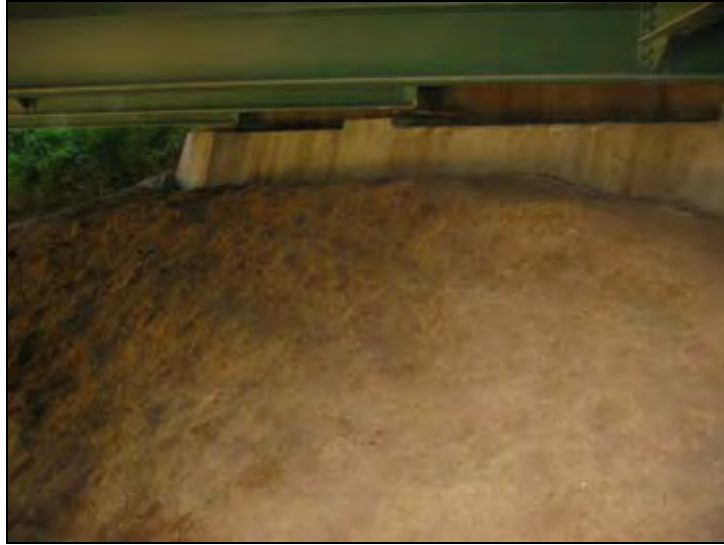
Figure 114. Loess soil used for the embankment
