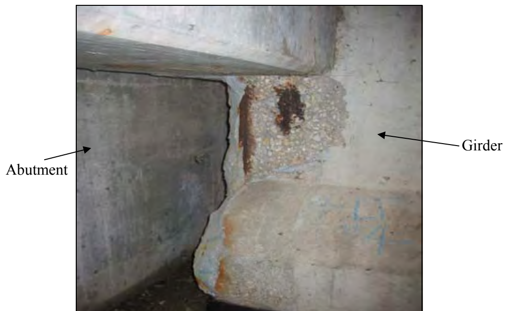
Figure 18. Deterioration of concrete with visible steel of the girders (South end NBL)
