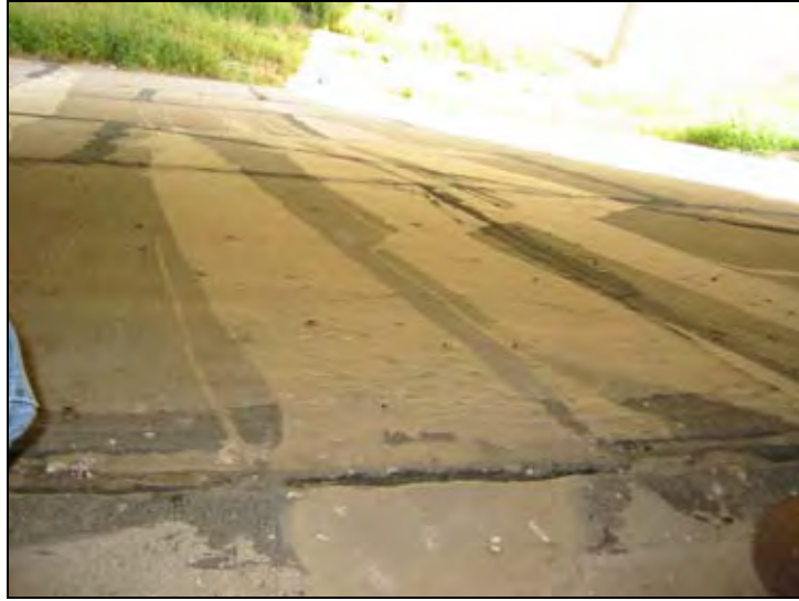
Figure 162. Grout seeping from under the concrete cover
