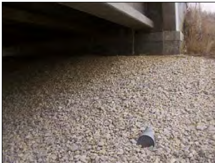
Figure 46. Aggregate used as a slope protection at the embankment under the bridge
