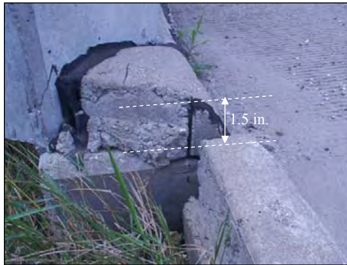
Figure 287. Differential settlement between the bridge slab and the bridge approach (North end of NBL)
