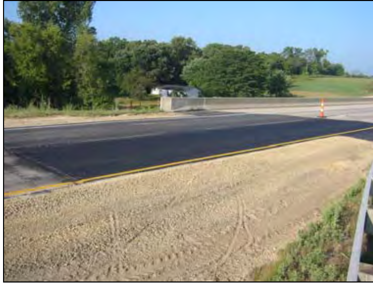
Figure 161. Approach slab asphalt overlay
