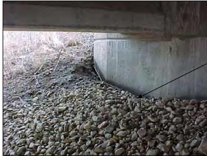
Figure 32. Aggregate used as slope protection at the embankment under the bridge
