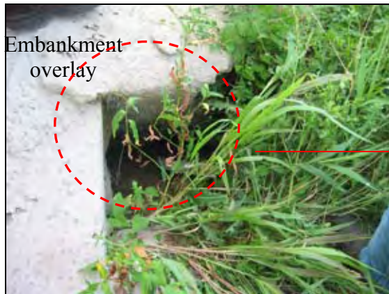
(a) Void under slope protection
