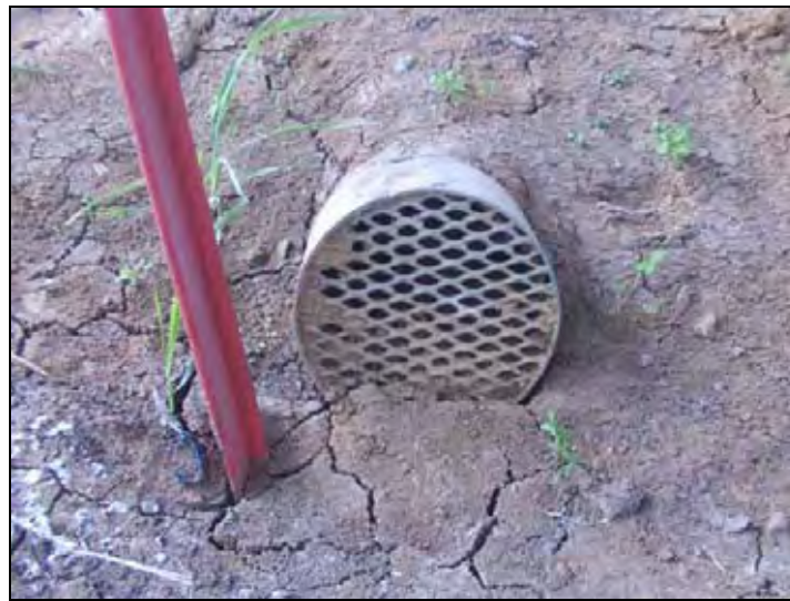
Figure 149. Perforated drain tile filled with soil (South end of SBL)
