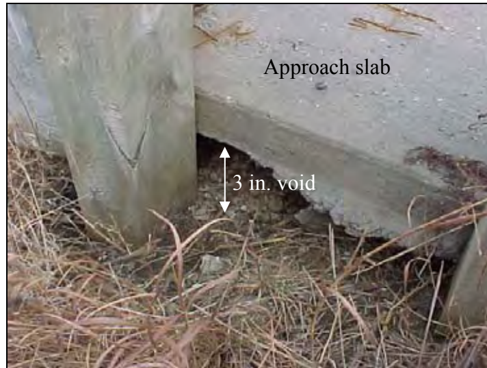
Figure 33. Void developed under the approach slab (South end of North bound bridge)
