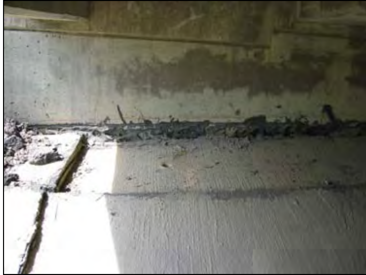
Figure 92. Uneven settlement of concrete slope protection
