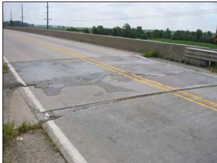
Figure 177. Deterioration of asphalt overlay at bridge approach
