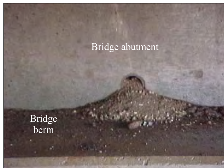
Figure 37. Weep holes filled with backfill material
