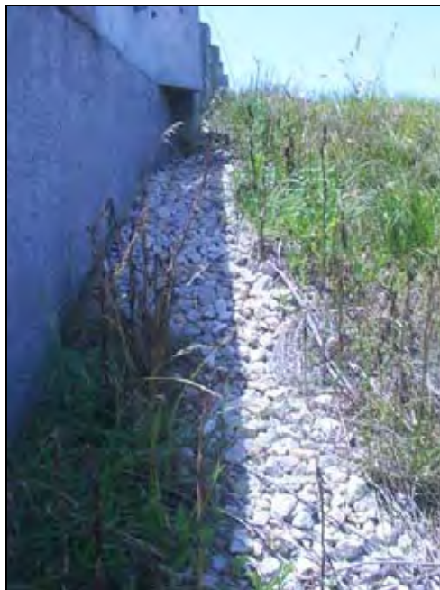
Figure 241. Aggregate placed at the sides of the abutment to control erosion (South end of SBL)
