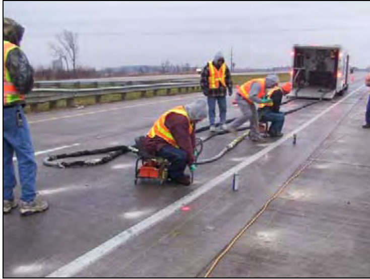
Figure 259. Injecting high-density polyurethane under the approach slab
