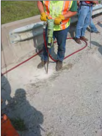
(a) Drilling at the approach slab
