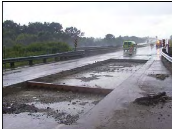
Figure 130. Bridge approach panel removed for replacement
