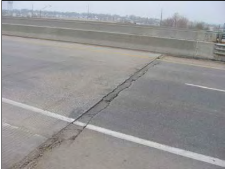
Figure A5. Cracks near the expansion joint
