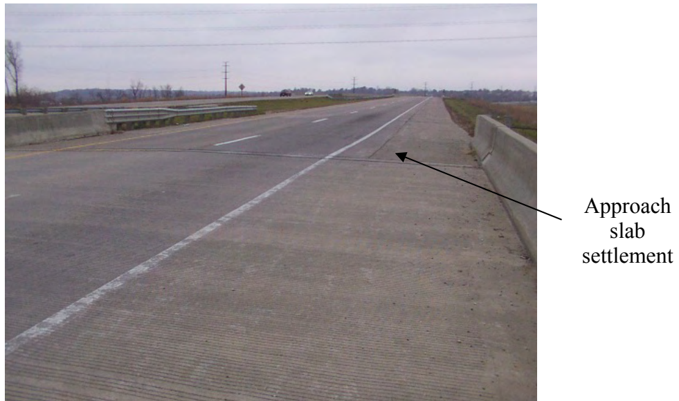
Figure 252. Settlement of approach slab (North end NBL)
