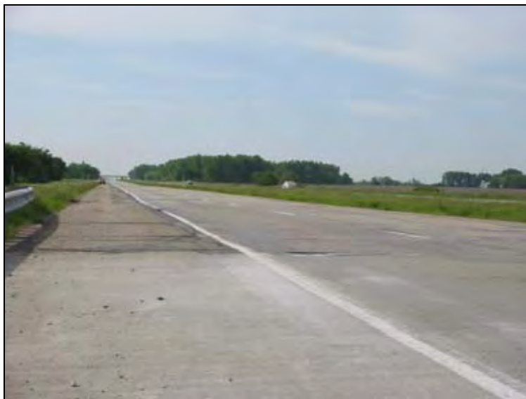
Figure 87. Wavy approach slab (NBL)
