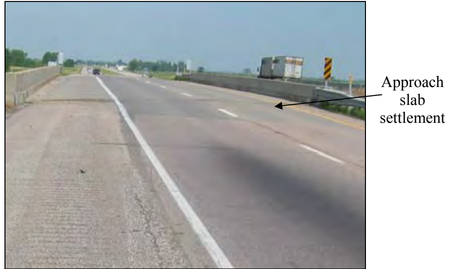
Figure 127. Settlement of bridge approach
