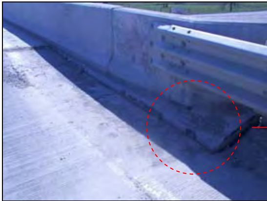
(a) Settlement of approach slab
