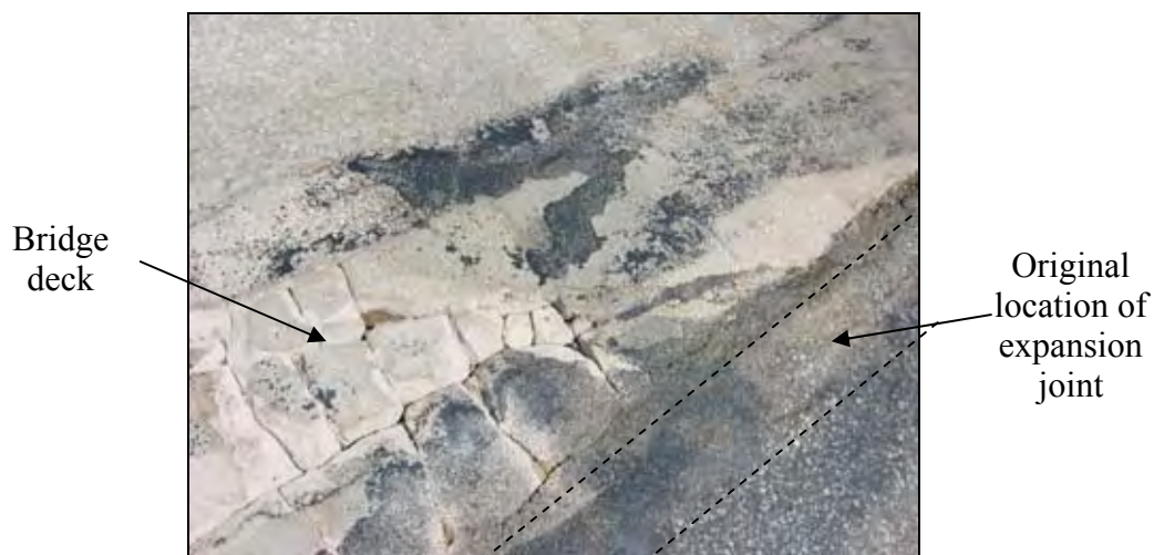
Figure 79. Breakage of bridge deck concrete
