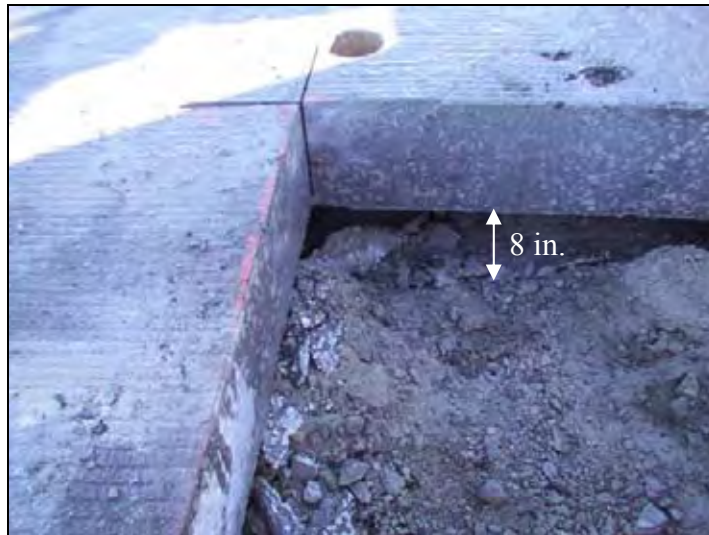
Figure 56. Eight-inch void observed under the approach slab
