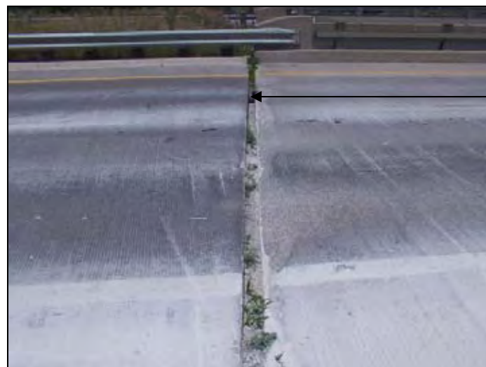
Figure 134. Expansion joint poorly sealed and filled with fines (West end of EBL)
