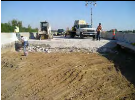
(a) Replaced approach slab
