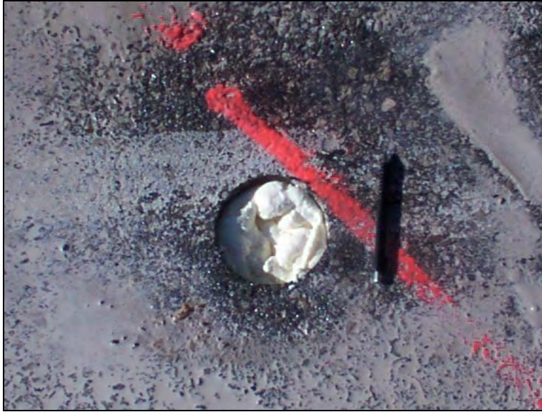
Figure 315. Expanding foam placed in the core hole of the approach slab (NBL)
