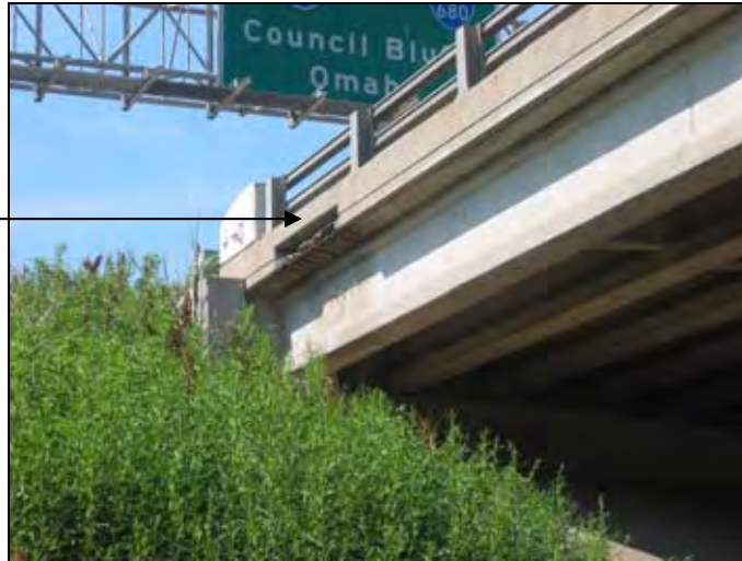
Figure 120. Surface drain of the bridge deck allowing water to fall on the embankment
