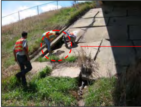
(a) Damaged slope protection
