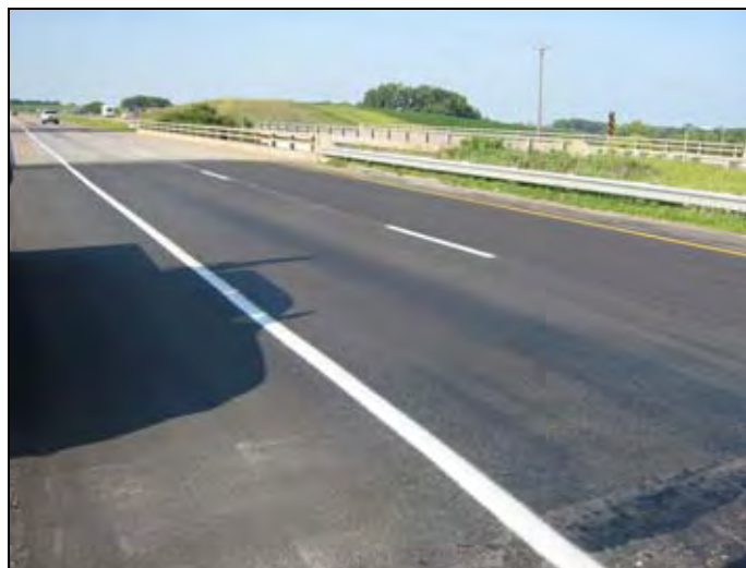
Figure 115. New asphalt-resurfaced approach
