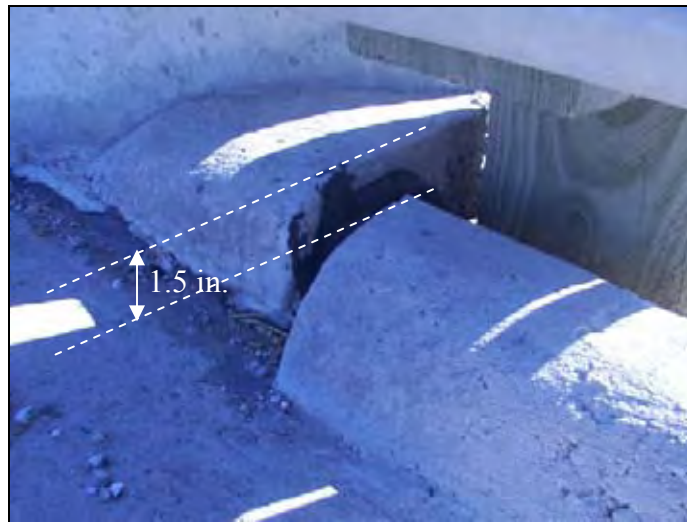
Figure 330. Differential settlement between the bridge approach and the approach slab (West end of EBL)
