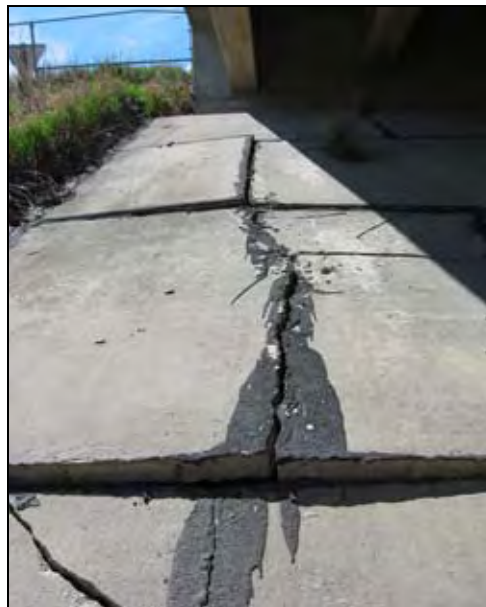
Figure 77. Fractured concrete slope protection
