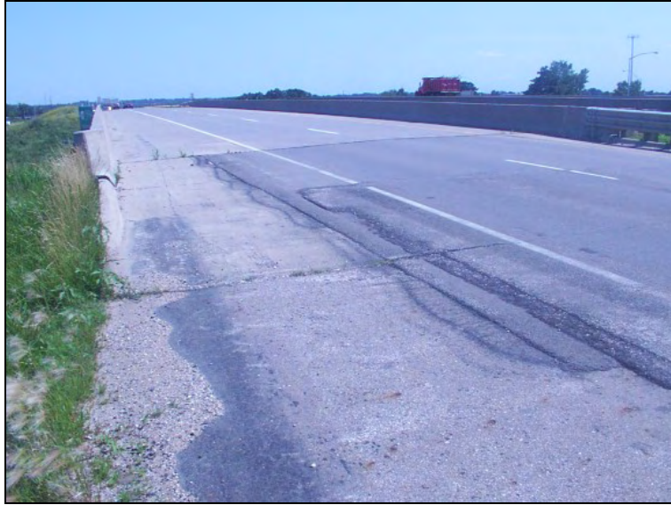
Figure 323. Asphalt overlay placed to compensate for the differential settlement (North of end NBL)
