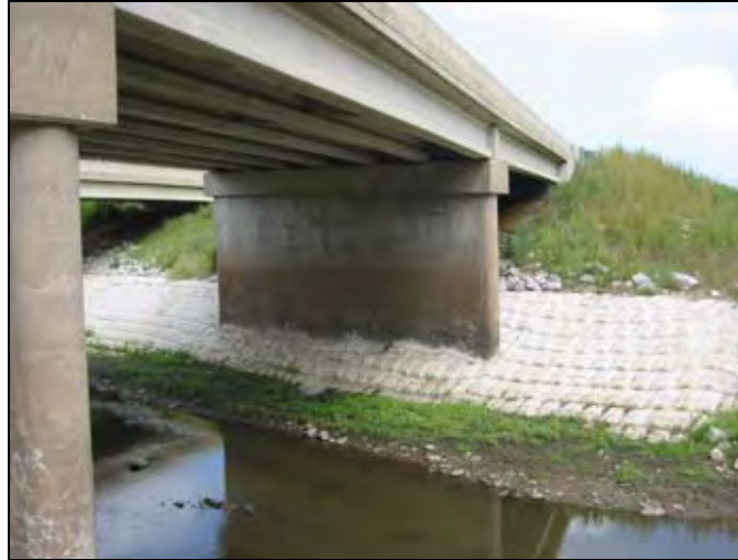
Figure 174. Rocks and pillows used for embankment stabilization
