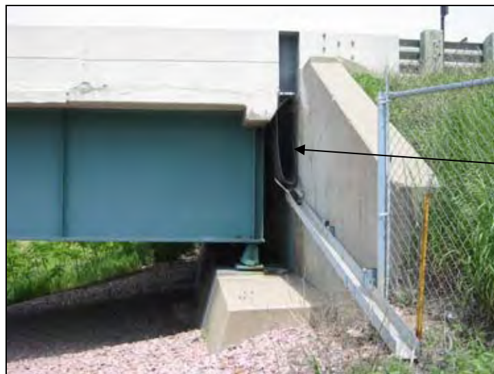
Figure 104. Drainage design at the end of the bridge in South Dakota
