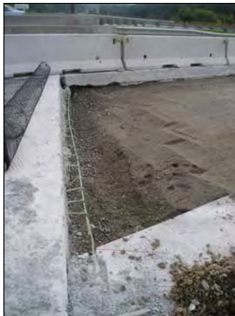
Figure 277. Compacted special backfill (South end of SBL)
