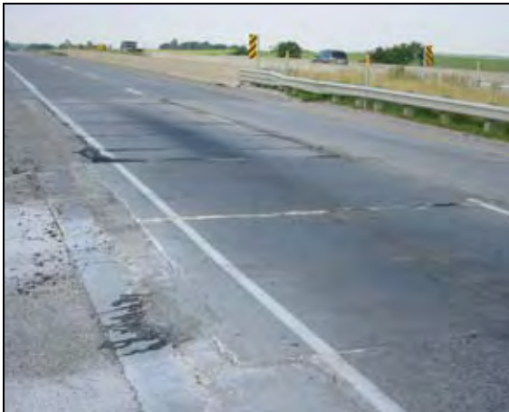
(a) Cracked approach slab panels
