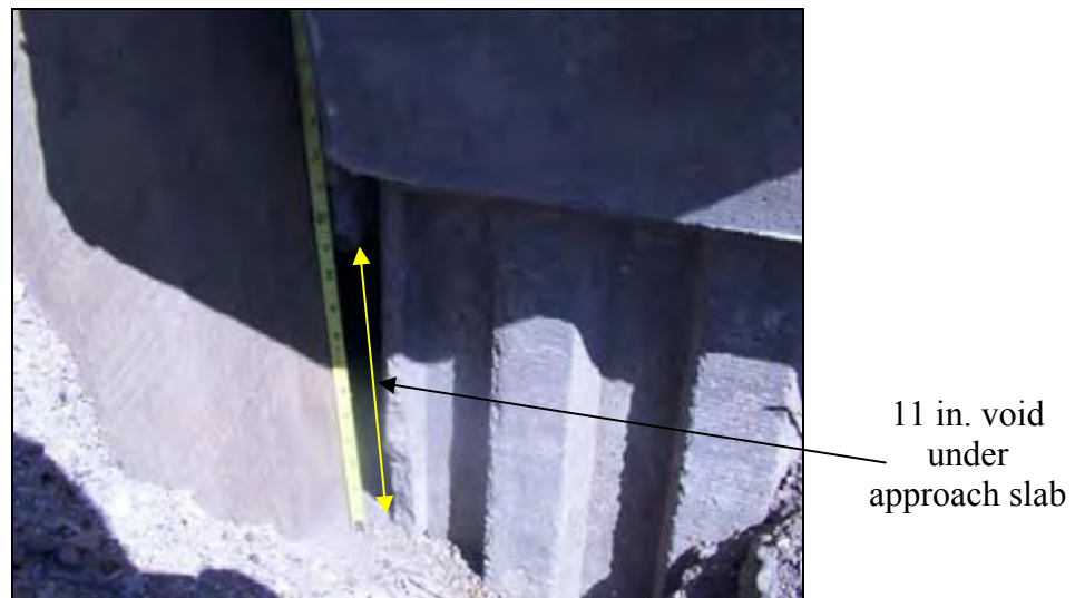
Figure 140. Void developed under the approach slab
