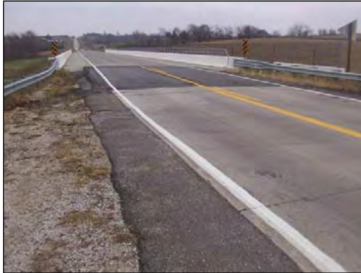
Figure 43. A view of the bridge showing recently placed asphalt overlay at the bridge approach (East end)
