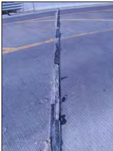
Figure 139. Deteriorated expansion joint filler
