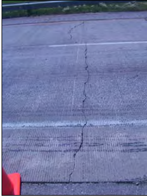
Figure 307. Transverse cracks at the bridge approach
