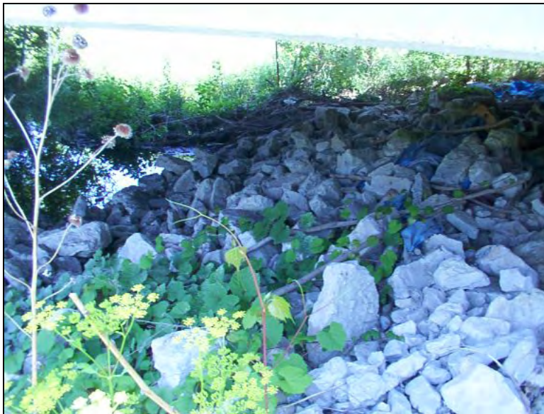
Figure 251. Rocks placed at the embankment under the bridge to prevent further erosion (South end of NBL)
