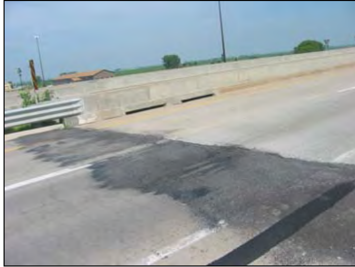
Figure 125. Asphalt patch placed at the approach slab
