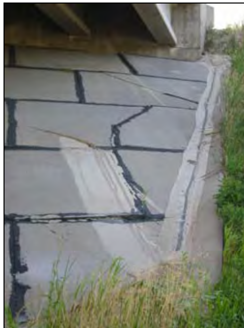
Figure 169. Cracking of the concrete slope protection overlay
