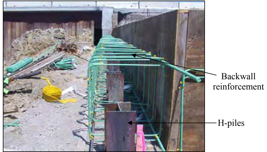
Figure 224. Reinforcement for the bridge backwall
