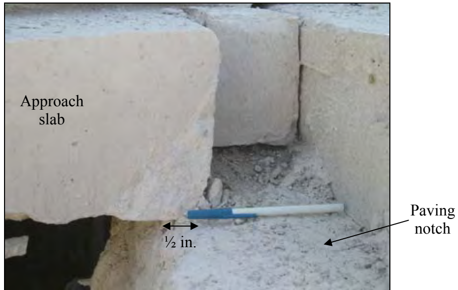
Figure 274. The approach slab resting on 0.5 in. of the paving notch (north end of SBL)
