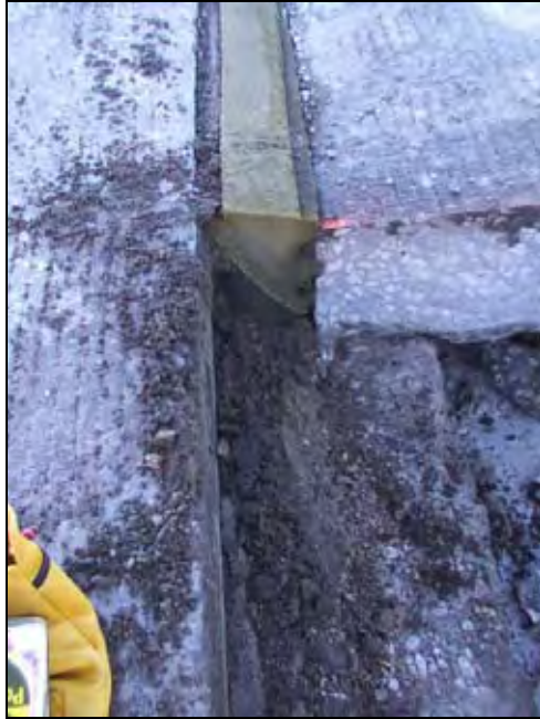
Figure 59. Contaminated expansion joint
