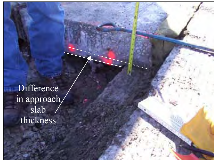
Figure 58. Non-uniform approach slab thickness with 1.5 in. increase over the backfill compared with the thickness over the paving notch
