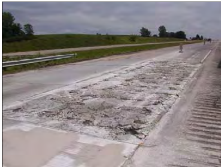
Figure 132. Approach pavement broken before replacement
