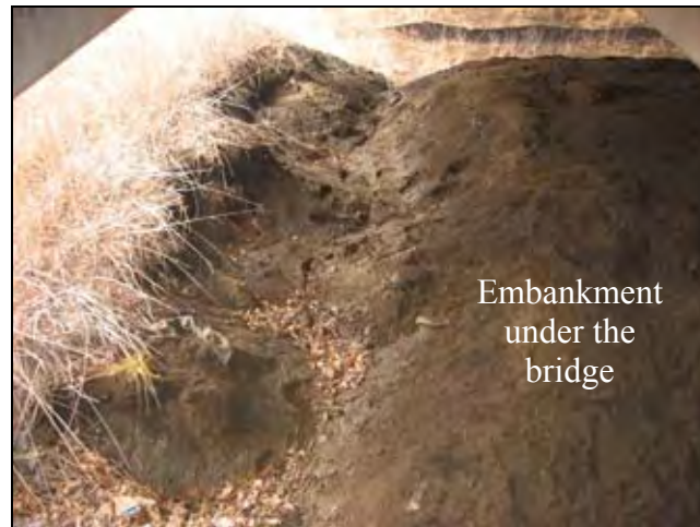
Figure 17. Soil erosion of the embankment under the bridge (South end of North bound)
