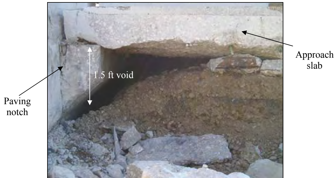
Figure 294. A void developed under the left lane approach slab which was 1.5-feet-deep at the bridge abutment (South end of SBL)
