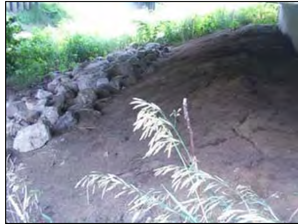
(b) Rip-rap used to control erosion
