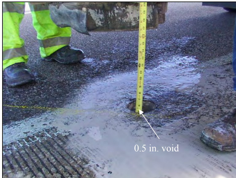
Figure 314. Measuring the void under the approach slab (North end of SBL)
