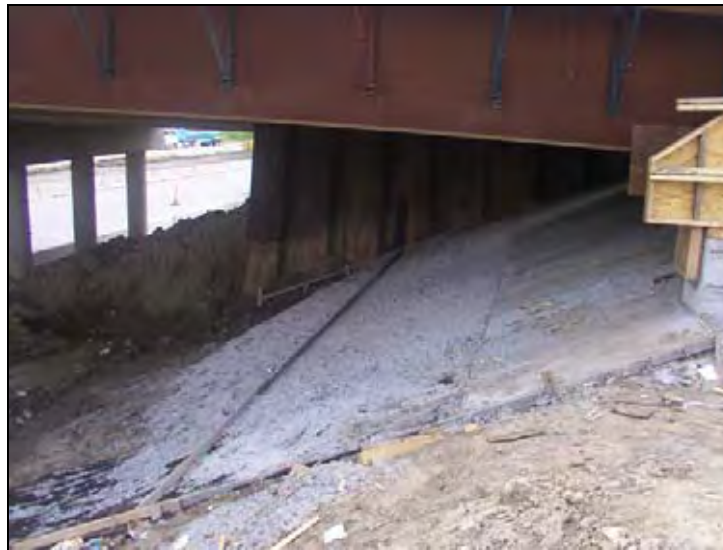
Figure 221. Construction of slope protection at the embankment
