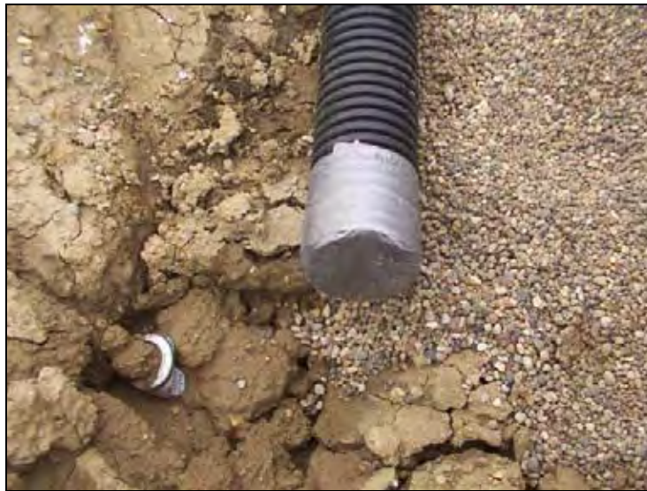
Figure 185. Porous fill placed around the drainage pipe
