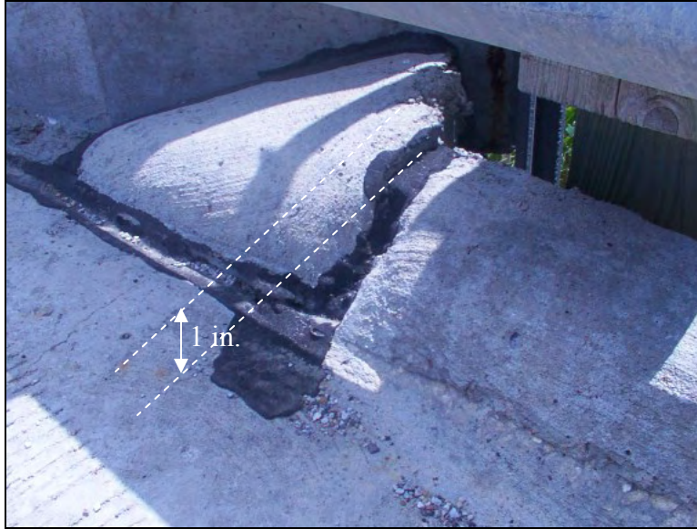
Figure 240. Differential settlement of 1 inch between the bridge slab and the bridge approach (South end of SBL)
