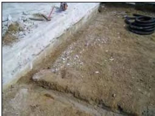
(a) Trench excavated to install subdrain
