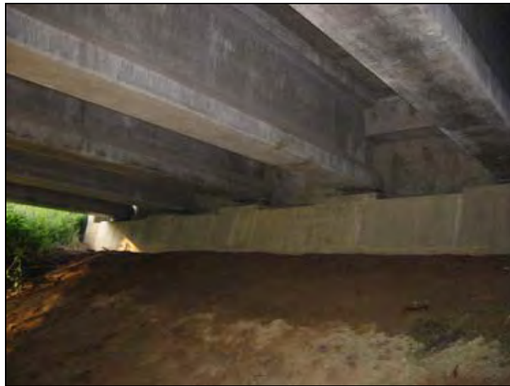
Figure 160. Wet loess soil observed at the embankment under the bridge
