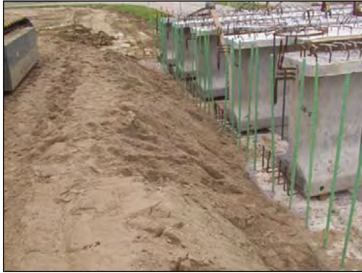
Figure 184. Granular Backfill used behind the abutment
