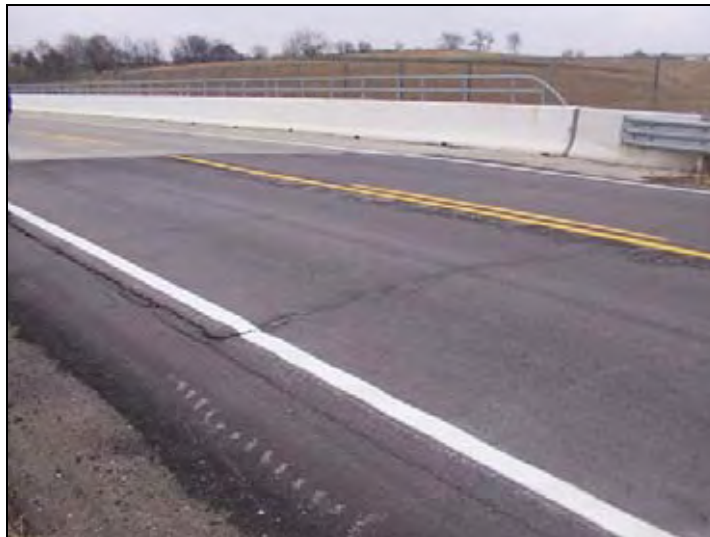
Figure 44. Cracking of the asphalt overlay (East end)
