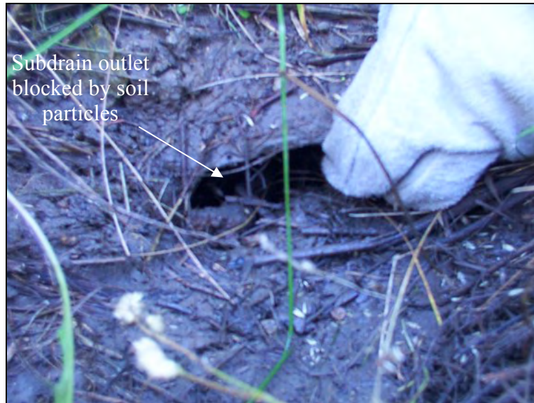
Figure 306. Subdrain outlet, located at the bottom of the embankment, blocked by soil debris
