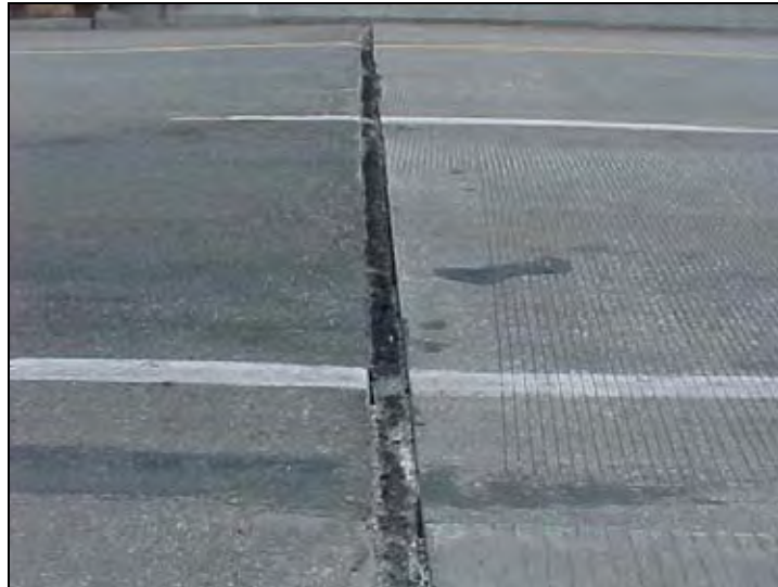
Figure 31. Poorly filled expansion joint with recycled tires used as a joint filler (North end SBL)
