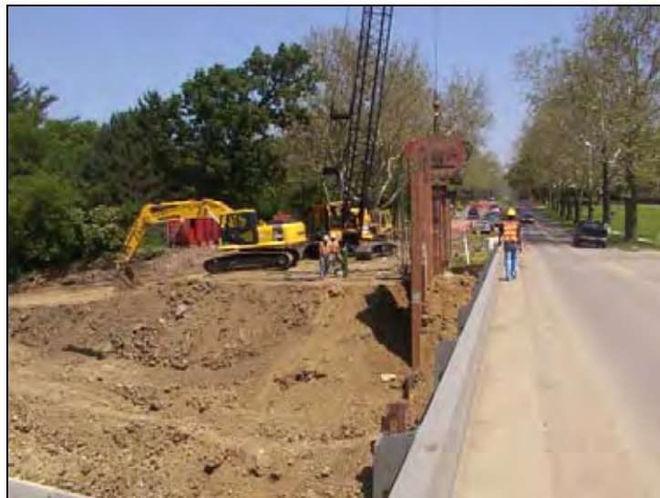
Figure 193. Installation of the sheet piles (NBL)
