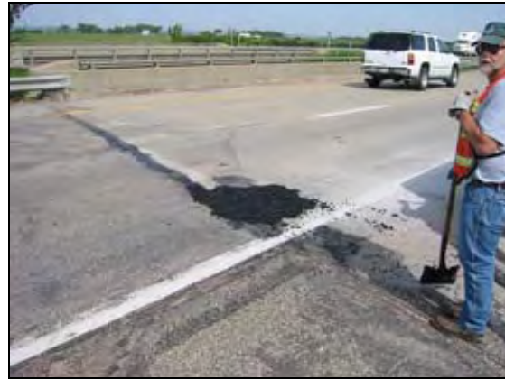
(b) Asphalt patch covering the cracks
