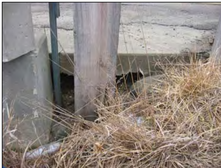
Figure A2. Void developed under approach slab
