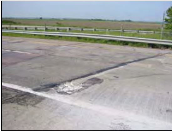
(a) Cracks on the bridge deck
