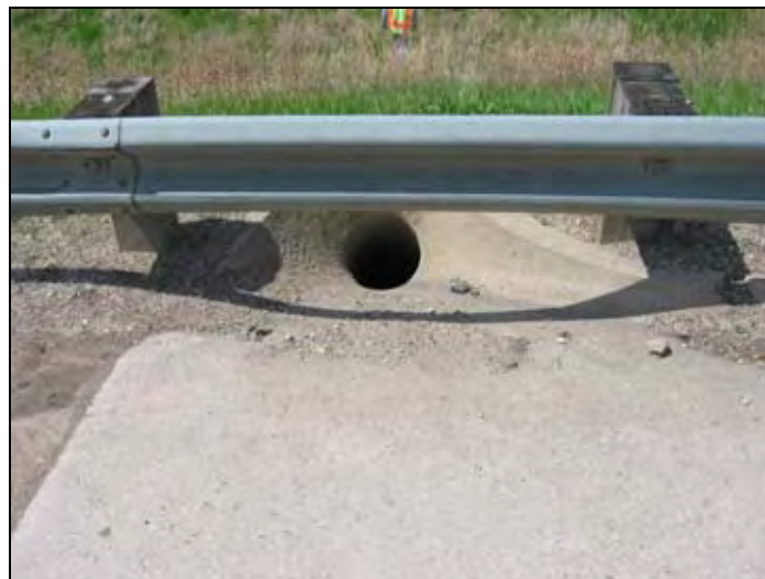
Figure 81. Surface drainage inlet at the bridge approach
