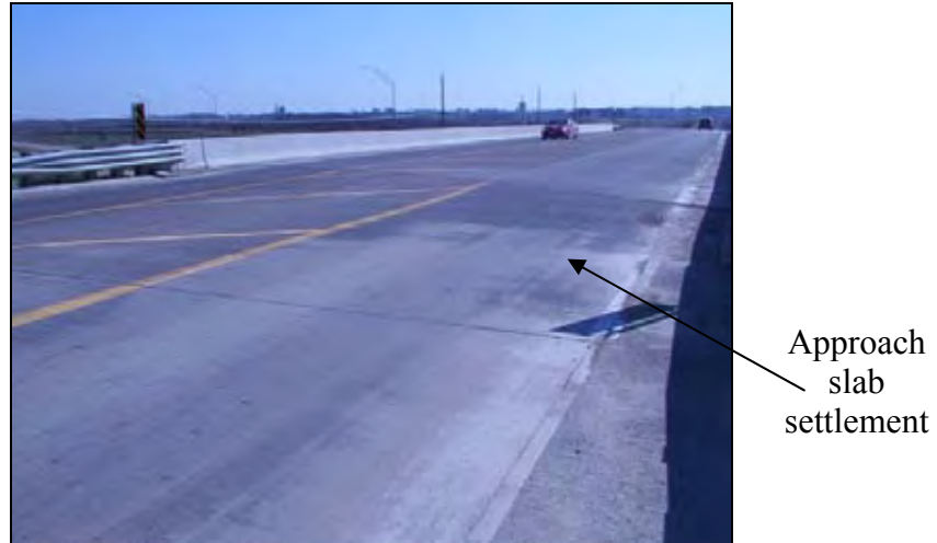
Figure 137. Settlement of approach slab
