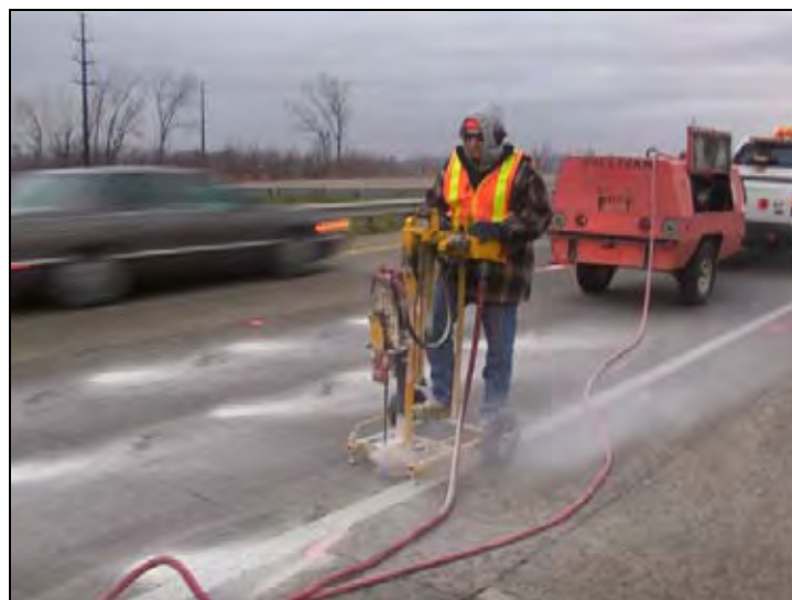
Figure 256. Holes drilled on the approach slab
