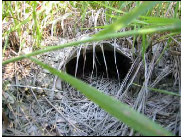
Figure 108. End drain plugged with soil
