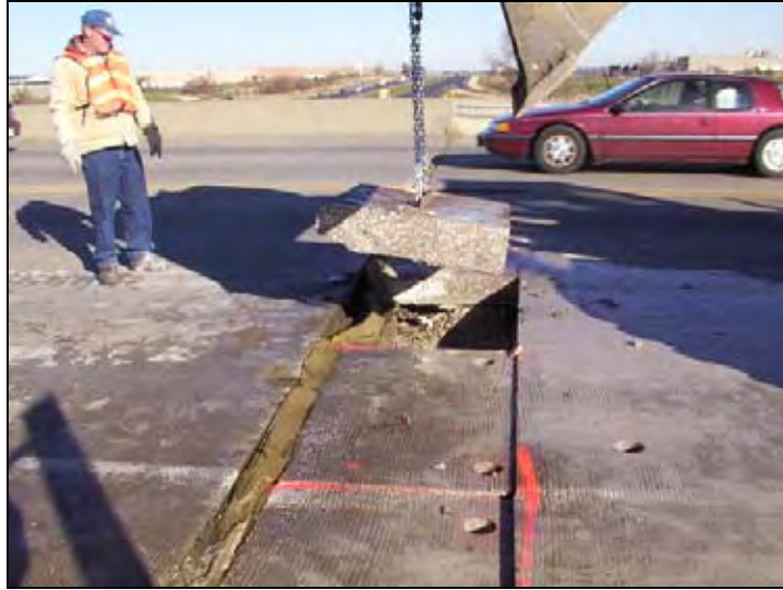
Figure 55. Removing a segment of the bridge approach
