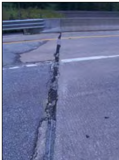
Figure 153. Poor performing resurfaced bridge approach (West end of WBL)
