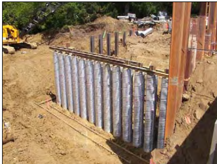
Figure 195. Installation of H-Piles (North end of NBL)
