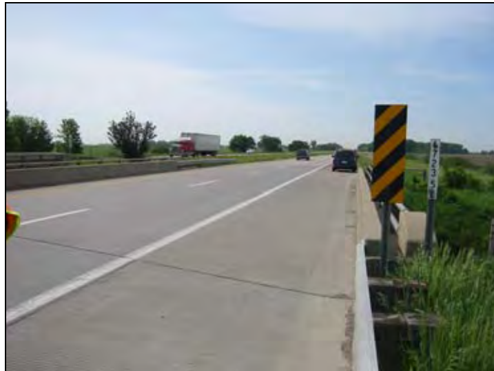
Figure 85. Recently replaced bridge approach slab (SBL)
