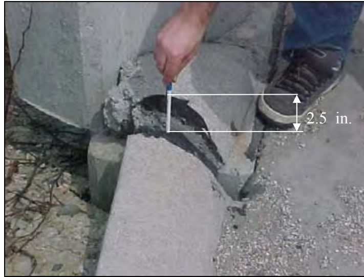
Figure 19. Differential settlement of 2.5 inches at the end of the abutment wingwall (South end SBL)
