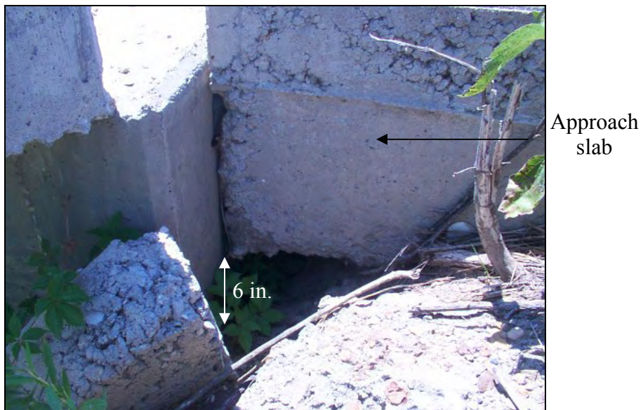
Figure 263. A 6 in. void developed under the approach slab (North end of NBL)
