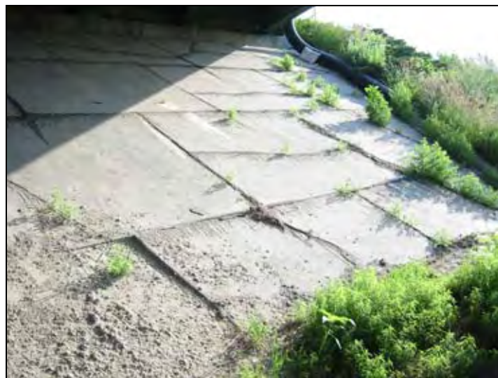
Figure 111. Cracking of concrete slope protection
