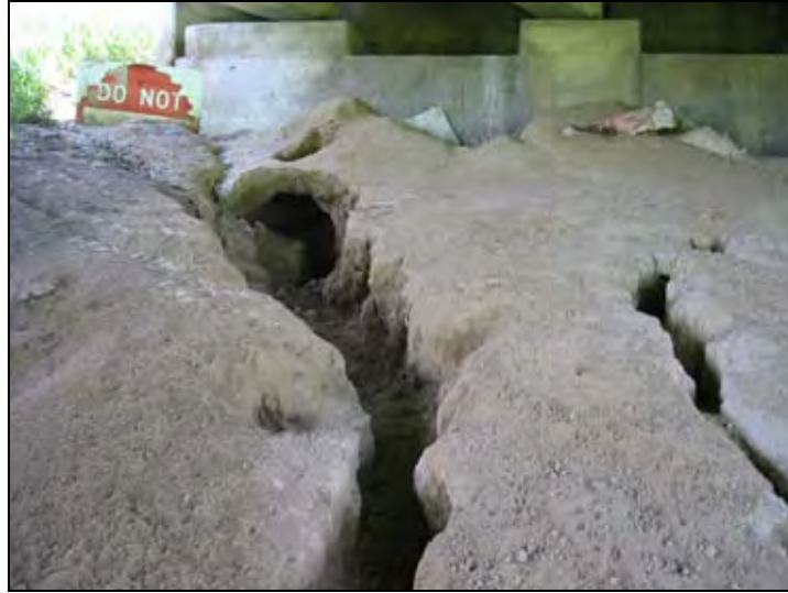
Figure 96. Severe erosion under the bridge
