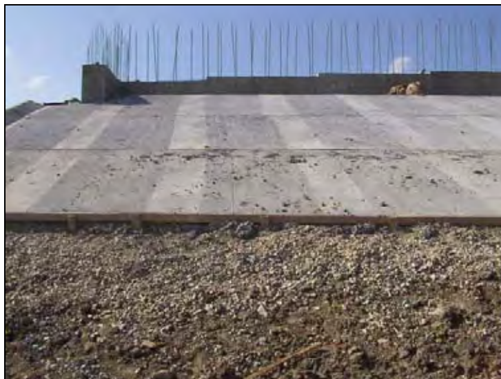
Figure 229. Construction of embankment slope protection
