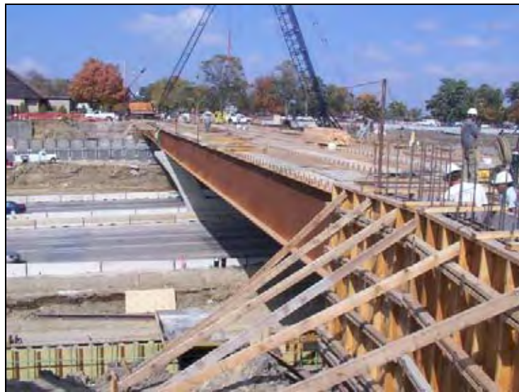
Figure 216. Construction of bridge slab (NBL)
