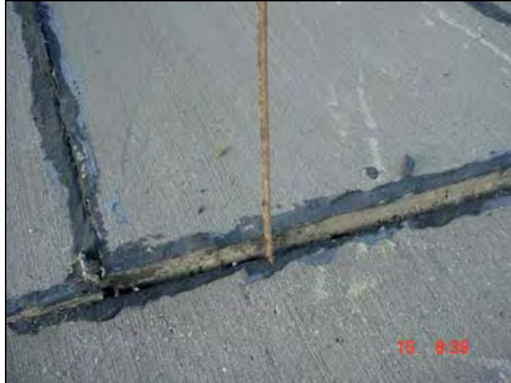
Figure 178. Uneven concrete slope protection
