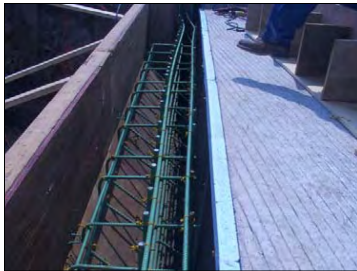
Figure 238. Abutment reinforcement (North end of NBL)
