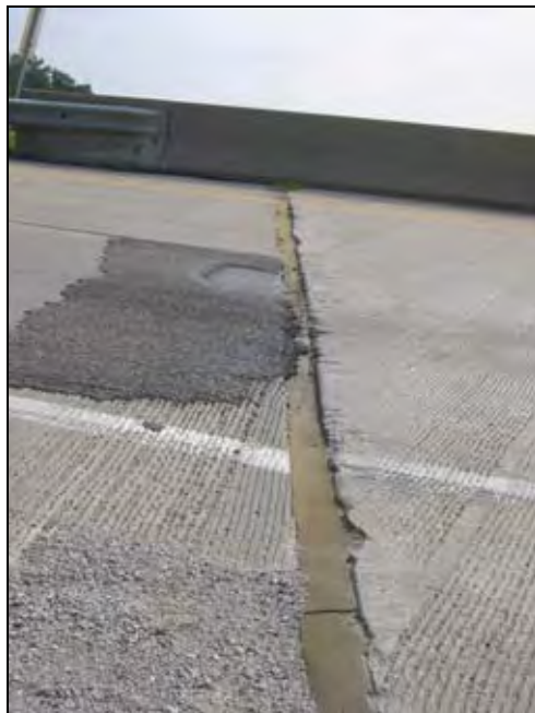
Figure 167. Flexible foam used as joint filler
