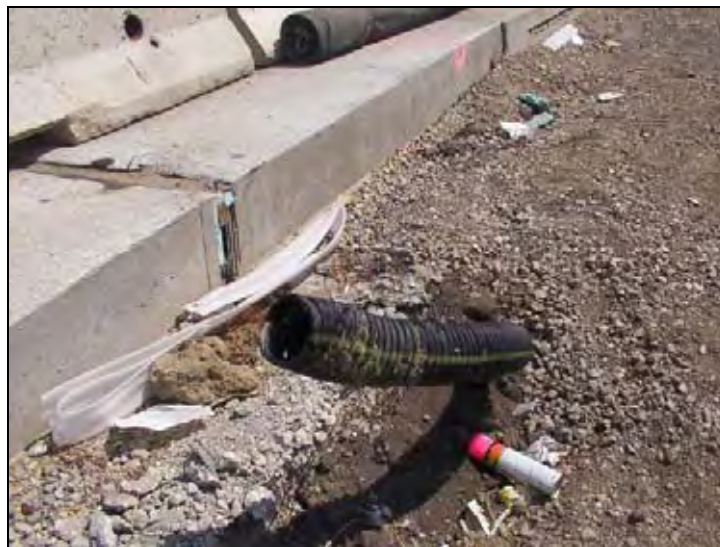
Figure 223. End drain outlet filled with soil
