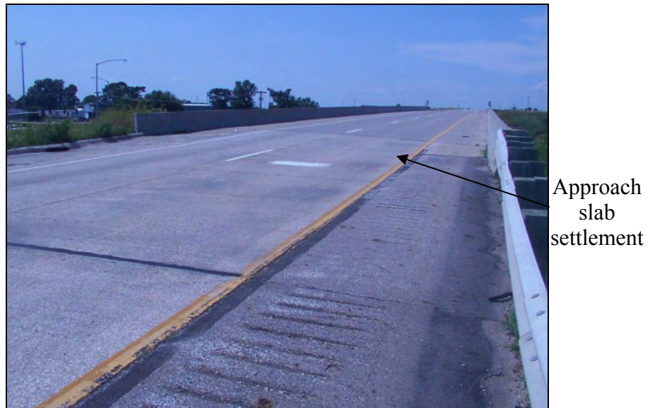
Figure 320. Bridge approach settlement (South end of SBL)
