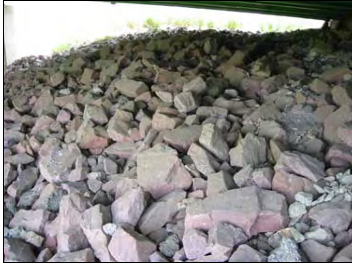
Figure 101. Aggregate used as embankment slope protection
