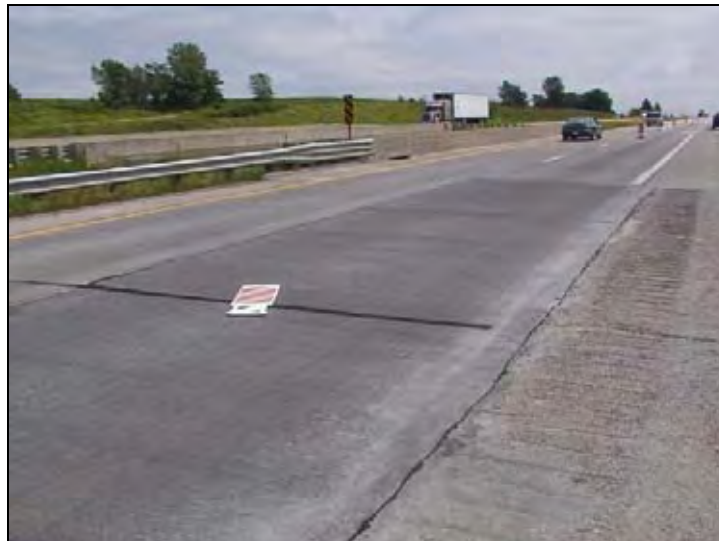
Figure 136. Replaced bridge approach slab
