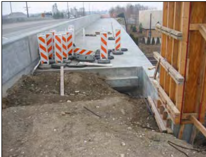
Figure 42. Non-compacted granular backfill behind the bridge abutment
