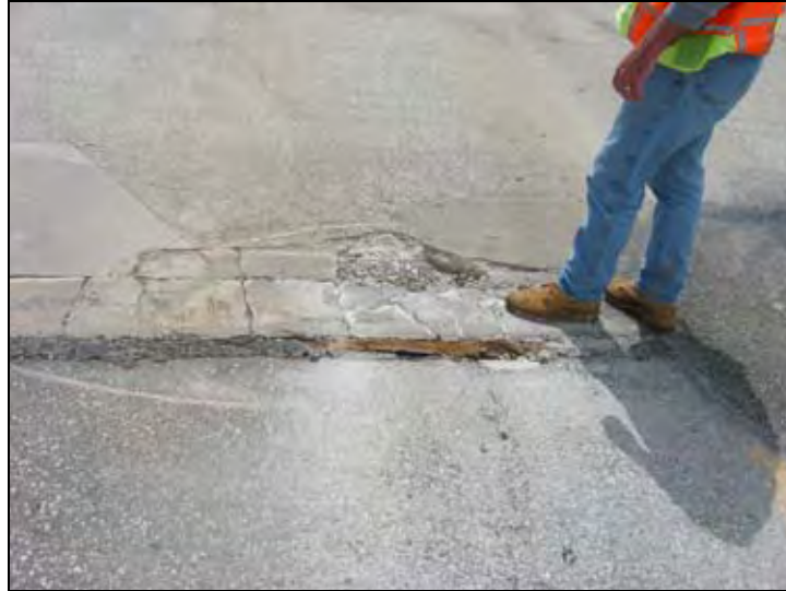
Figure 83. Cracks in the bridge deck concrete
