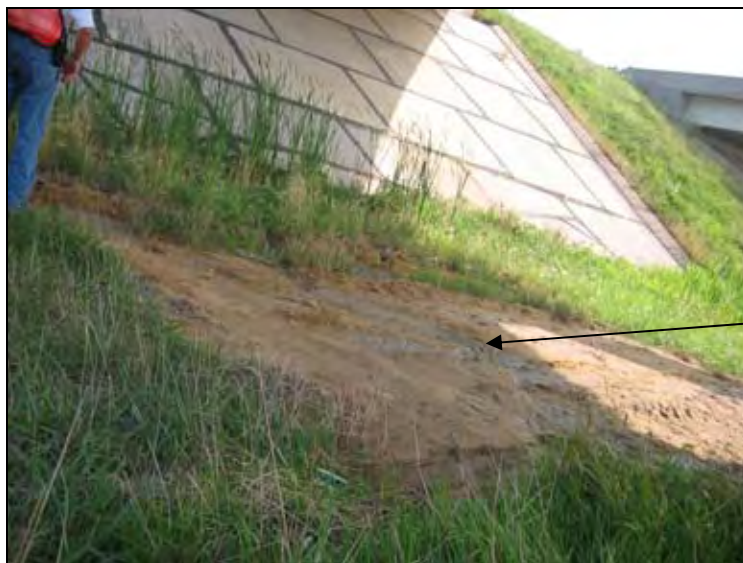
Figure 163. Grout seeping from the bottom of the embankment
