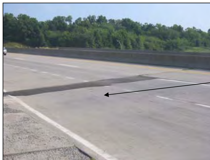
Figure 165. Differential settlement at approach slab
