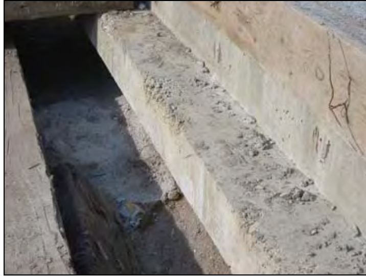
Figure 232. Poor construction of bridge paving notch
