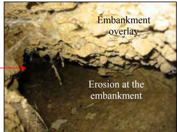
(b) Closer image of the developed void
