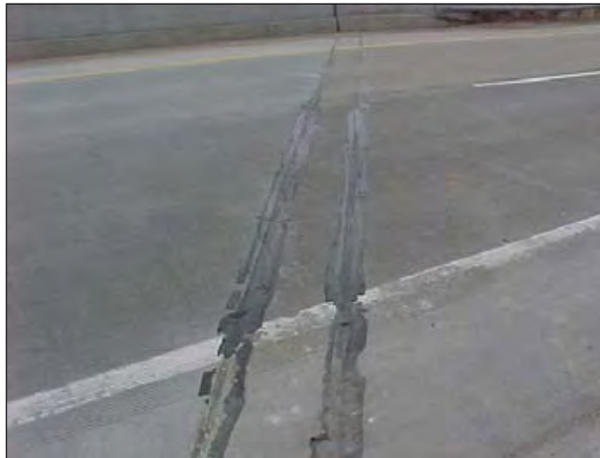
Figure 39. Deteriorated sealer at the expansion joint
