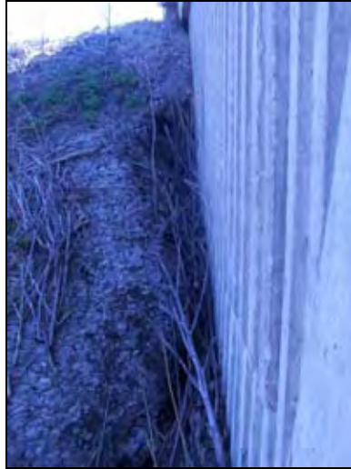
Figure 144. Erosion around the abutment (East end)
