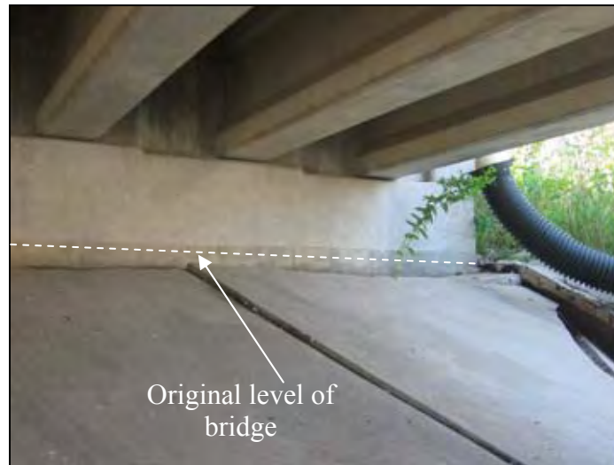
Figure 123. Concrete cover settlement of 10.5 in.
