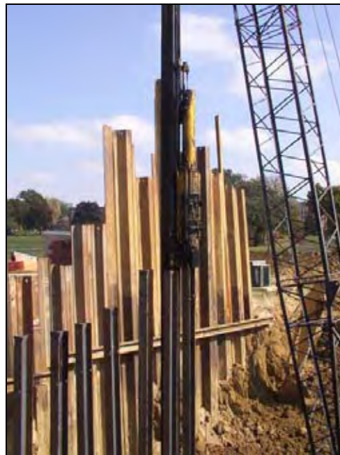
Figure 199. H-piles being driven
