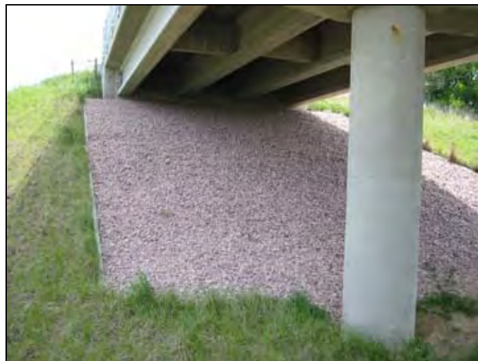
Figure 97. Aggregate slope protection of the embankment under the bridge
