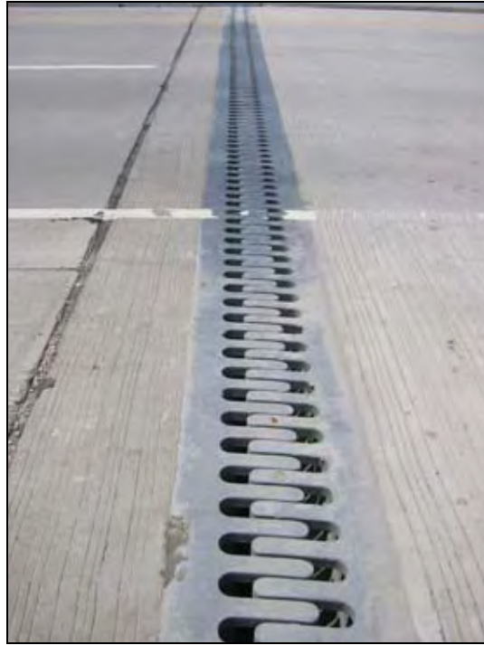
Figure 100. Finger type joint
