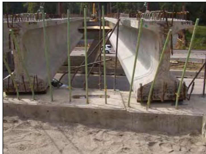
Figure 197. Sand used as granular backfill material
