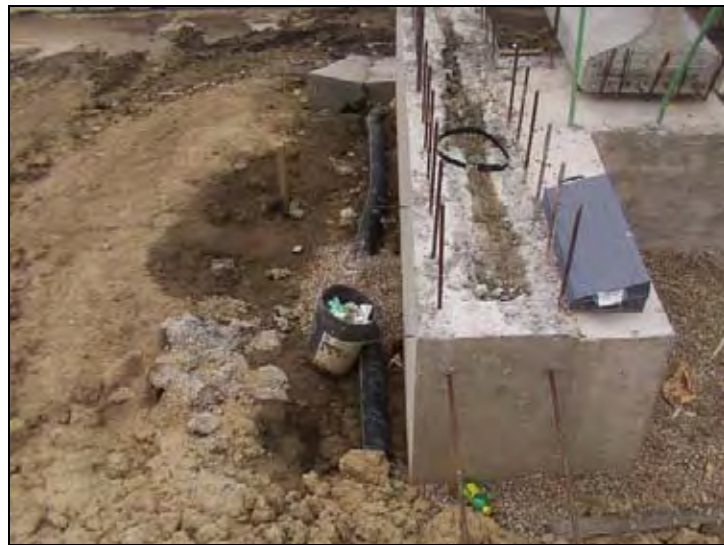
Figure 187. Subdrain along the side of the abutment
