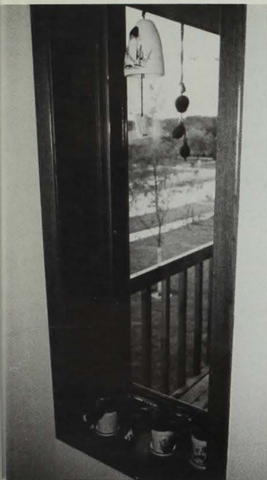
The only visible evidence of a superinsulated house is its deep-set windows.
