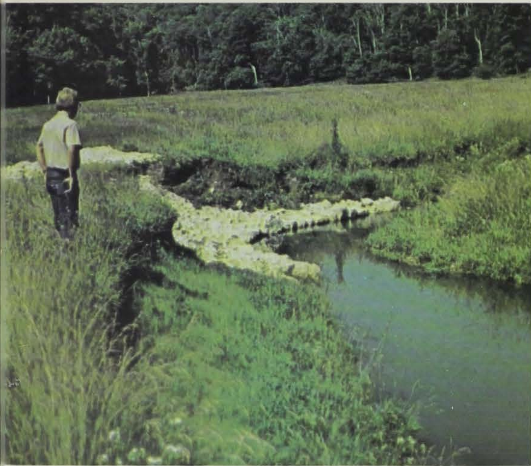
In-stream habitat enhanced by construction of bank hides on South Fork Big Mill.
