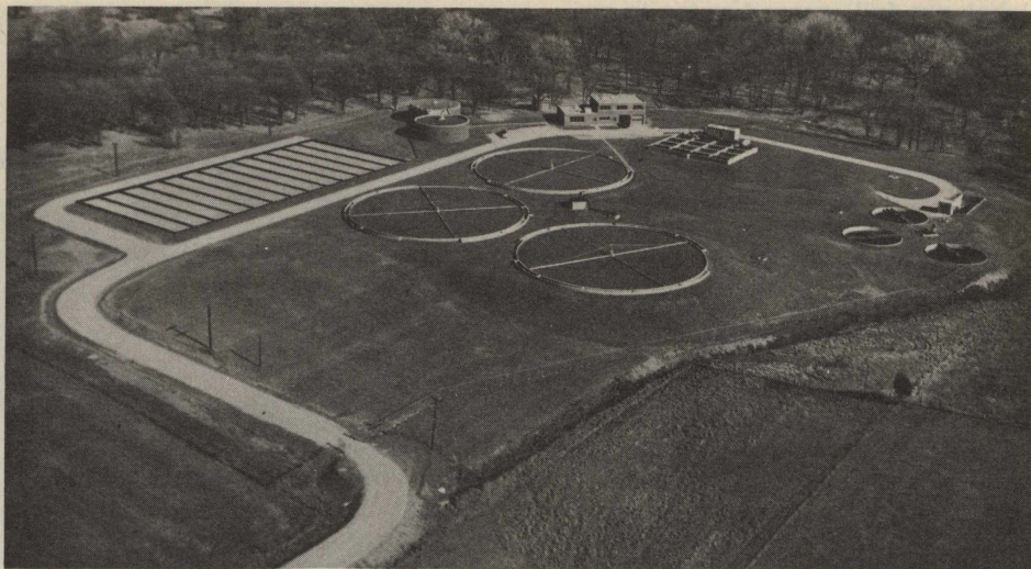
Fig. 2.7. Wastewater treatment plants help to prevent stream pollution. These plants remove solid materials from sewage and permit bacterial and chemical action to render most of the sewage harmless before it enters the stream.
