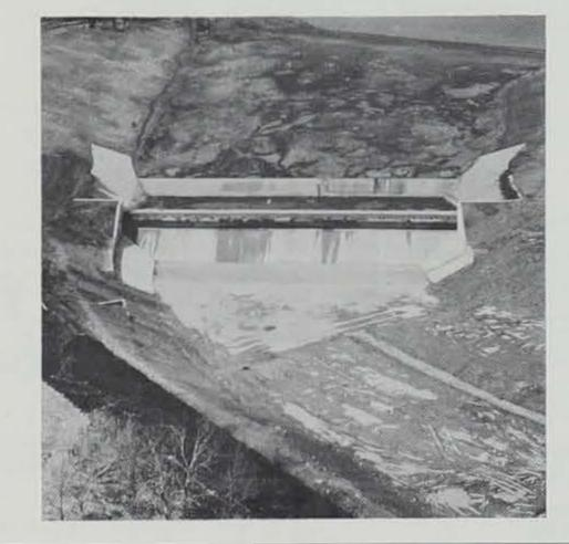
Above: Erosion and spillway damage before construction started, point out the need for maintenance work at Rock Creek.
