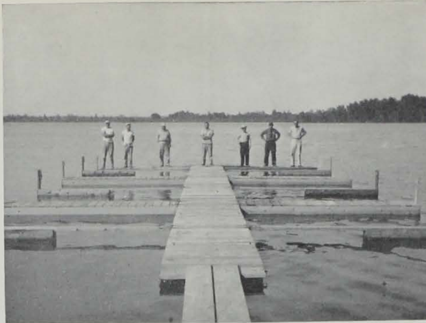
These seven men are standing on one of the new type plastic foam floating docks constructed at Lake Odessa. Notice that even with more than half a ton bearing on them, the docks are not noticeably depressed. They'll rent for $2 per week, $5 per month and $20 per season. Many are already taken.
