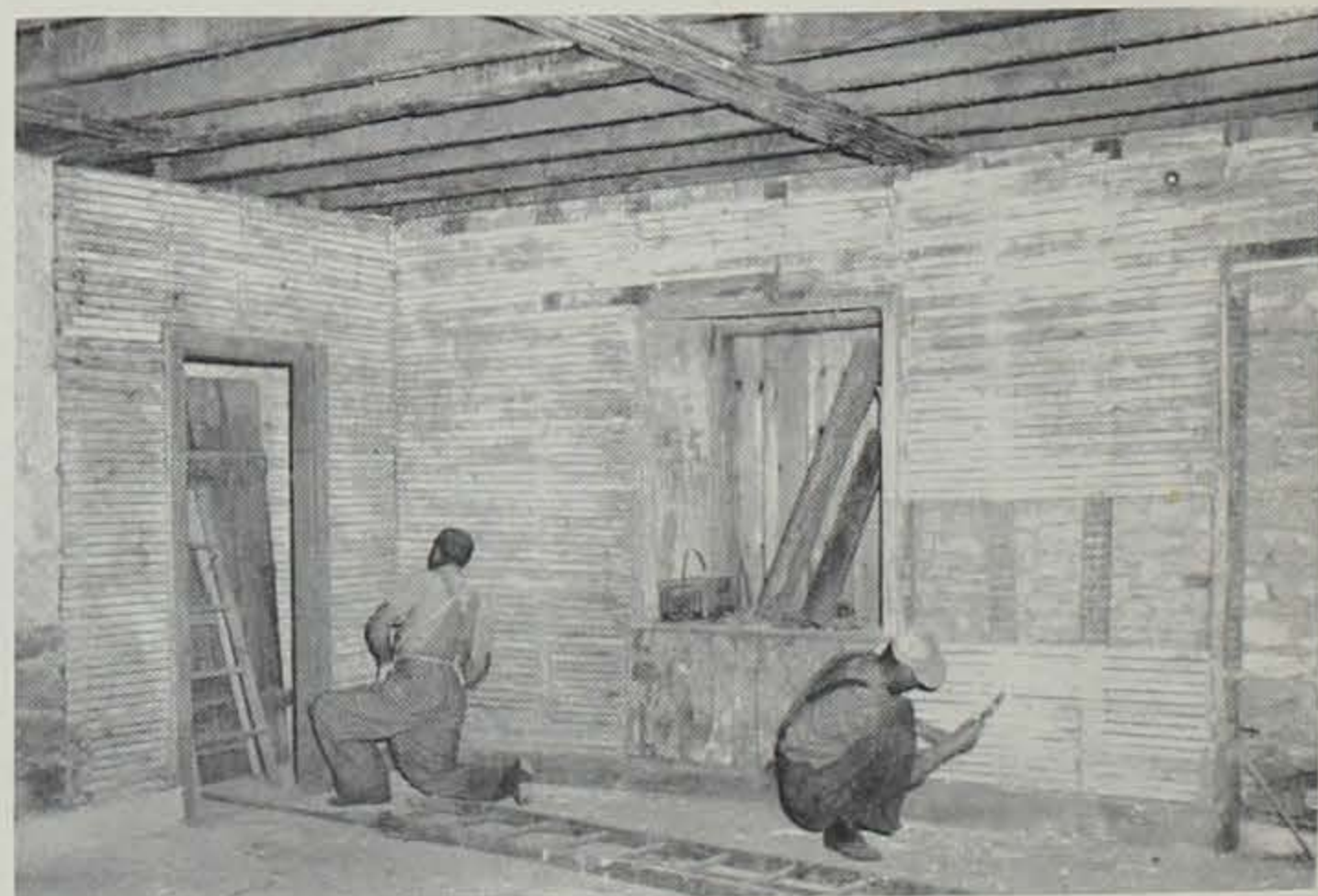
Workmen here are completing some lathing on the inside of the old barracks building at Fort Atkinson. Work at the fort is slow and tedious because of one important objective—to restore as nearly as possible the fort as it appeared in 1840.
