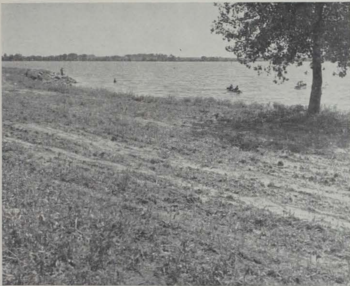
The park land at Storm Lake was made by dredging silt and sand from the bottom of the lake into a fill area enclosed by a dike. Jim Sherman Photo.
