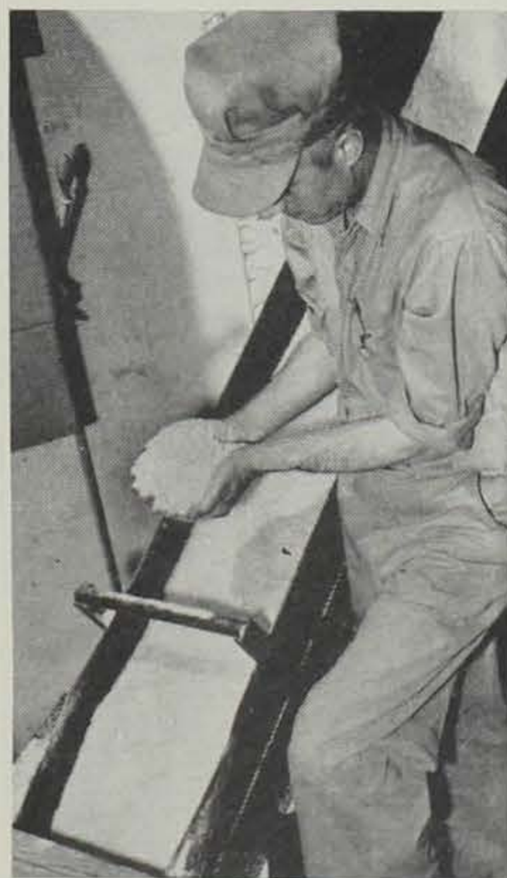
Sawdust gold, formerly waste in the lumber industry, climbs a conveyor on its way to becoming Prespine wood panels. Monsanto Chemical Company Photo.
