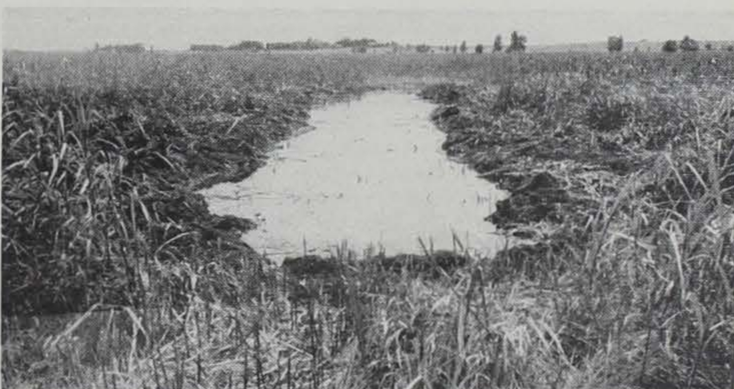
Blasting has created an open water area four feet deep and ten feet wide in this marsh. Tom Scott Photo.
