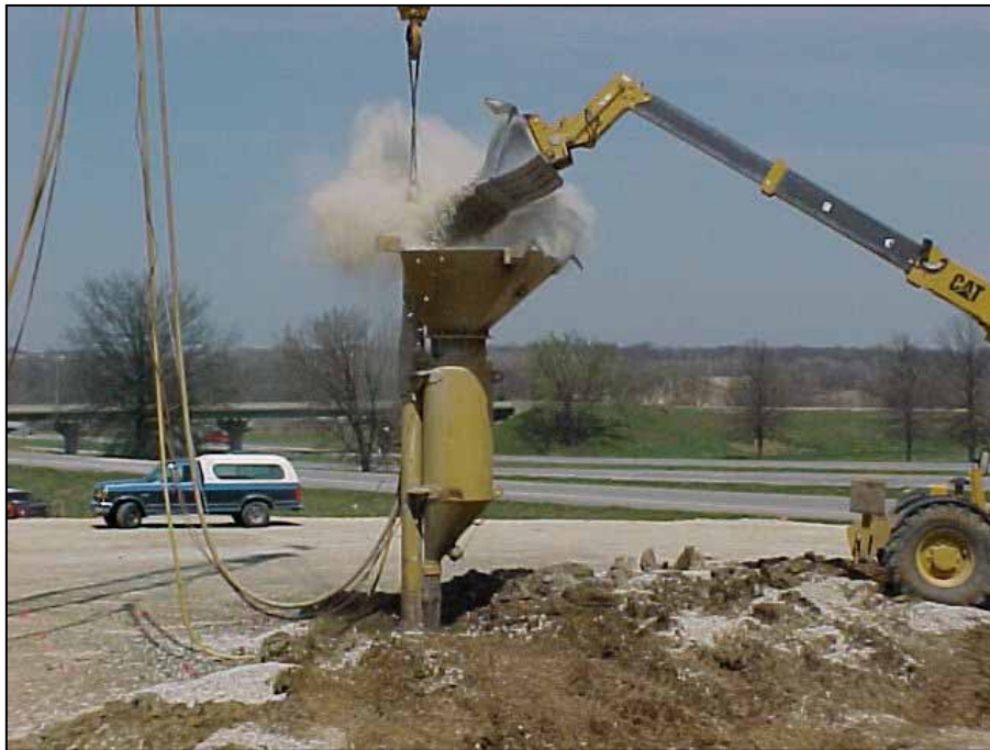
Figure 12. Stone column construction at I-35/Hwy 5 in West Des Moines, Iowa (Pitt et al. 2003)
