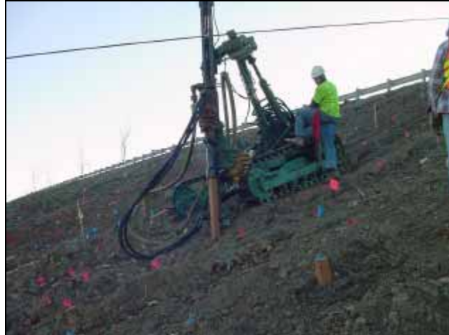
Figure 23. Installation of recycled plastic pins (from Loehr and Bowders 2003)
