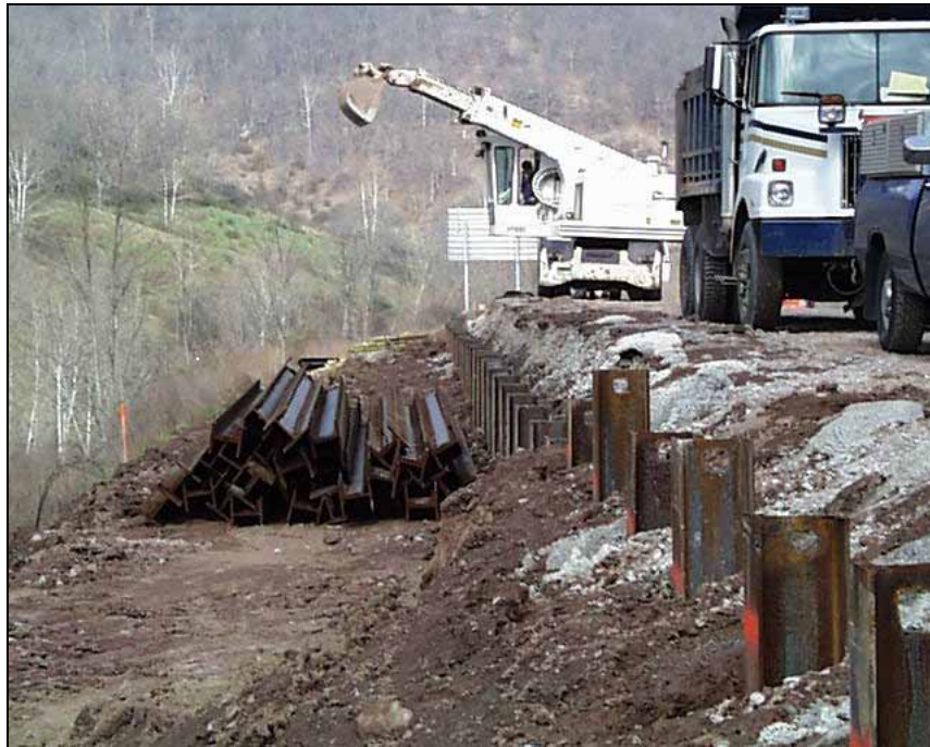
Figure 21. Pile wall construction in West Virginia (photo courtesy of Jim Fisher)
