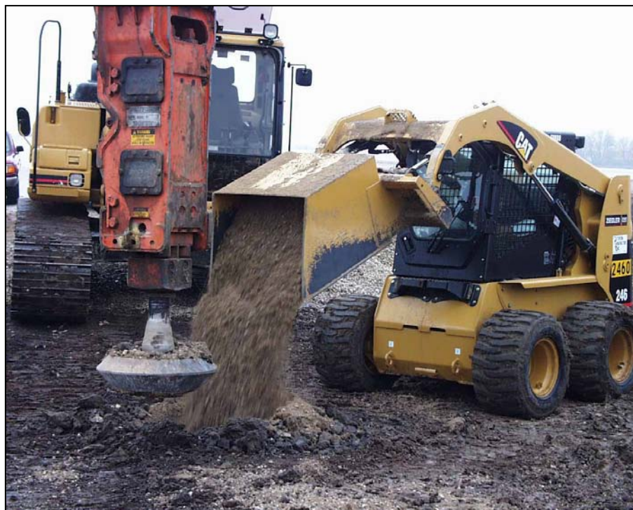
Figure 13. Rammed aggregate pier construction at I-35/Hwy 5 in West Des Moines, Iowa (Pitt et al. 2003)
