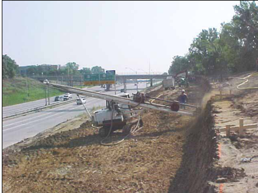
Figure 16. Installation of soil nails by drilling on I-235 in Iowa (from Makarla 2004)
