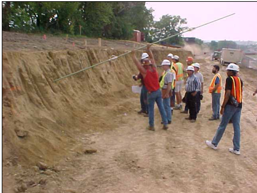
Figure 17. Placement of steel inclusion in drilled hole on I-235 in Iowa (from Makarla 2004)
