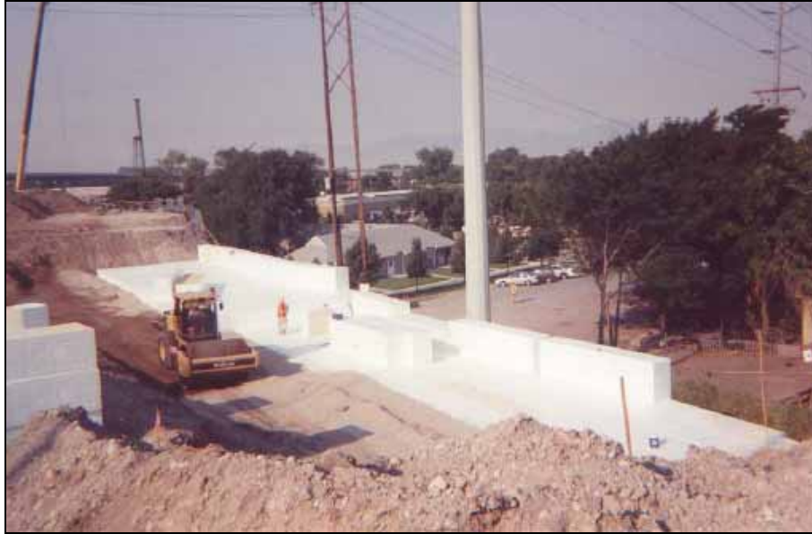
Figure 5. Soil compaction adjacent to geofabric fill (from Negussey and Stuedlein 2003)
