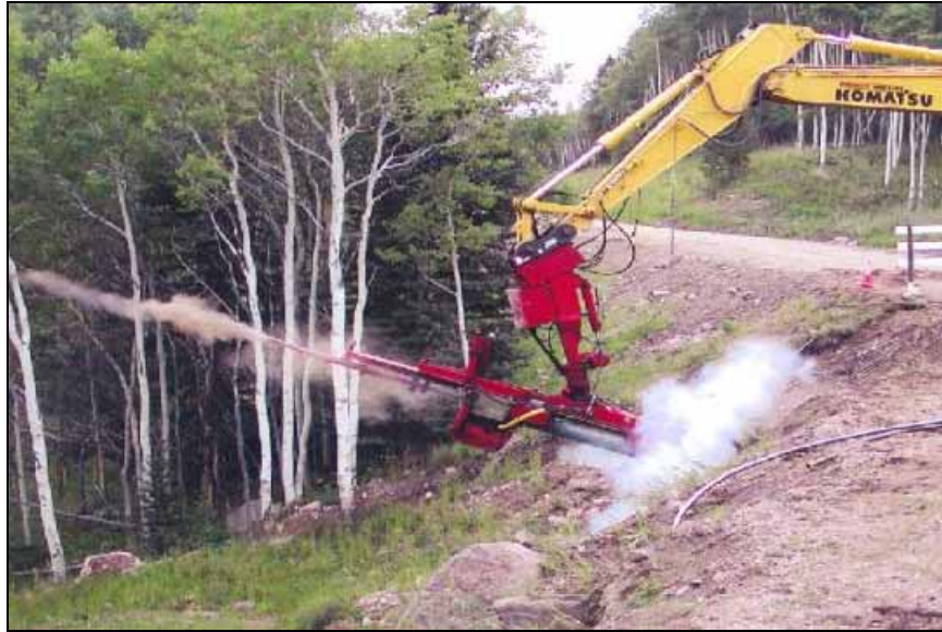
Figure 19. Installation of soil nails with launcher (from soilnaillauncher.com)
