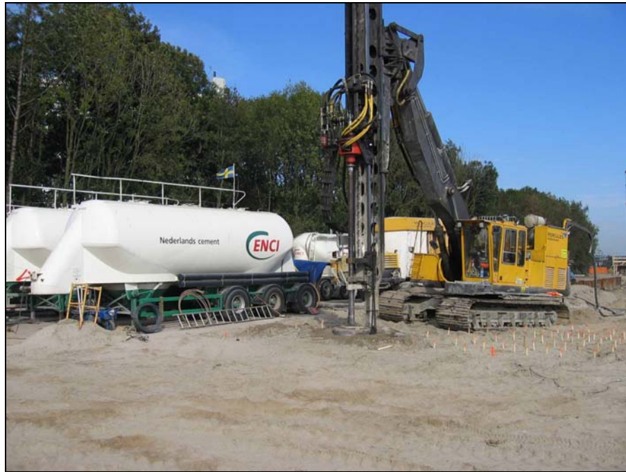
Figure 15. Lime/cement column installation
