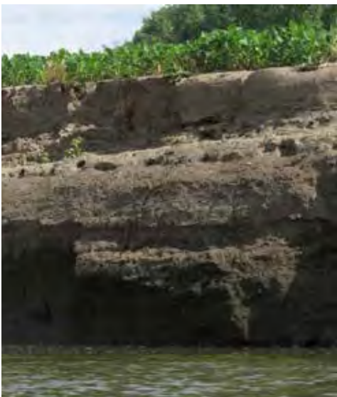
Severely eroded banks are visible along the South Raccoon riverbank in places. Shallow-rooted corn and soybeans are unable to hold ground against the eroding force of water. The farmland tears away, dumping soil into the river.
