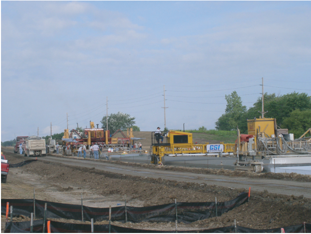
Measuring pavement profile during construction using the GOMACO Smoothness Indicator (GSI)
