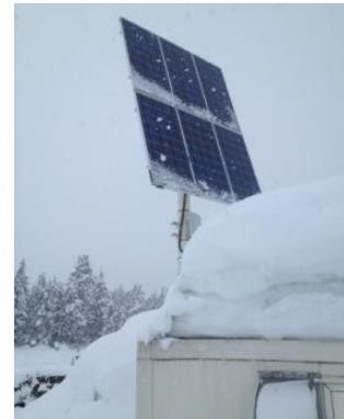
**Figure 1. Power supplies at a remote RWIS site in Alaska, from left to right: overall site, 8340K-WG972 propane DC generator, and six Kyocera 120 solar PV modules**
