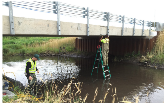
Instrumenting the bridge for live load tests
