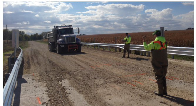
Load Case 5 live load testing
