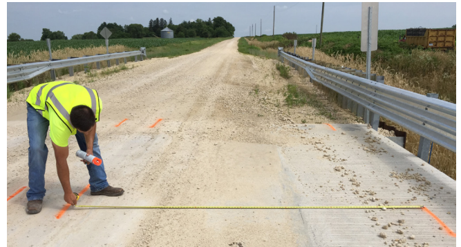
Measuring and marking wheelpath bounds for load tests
