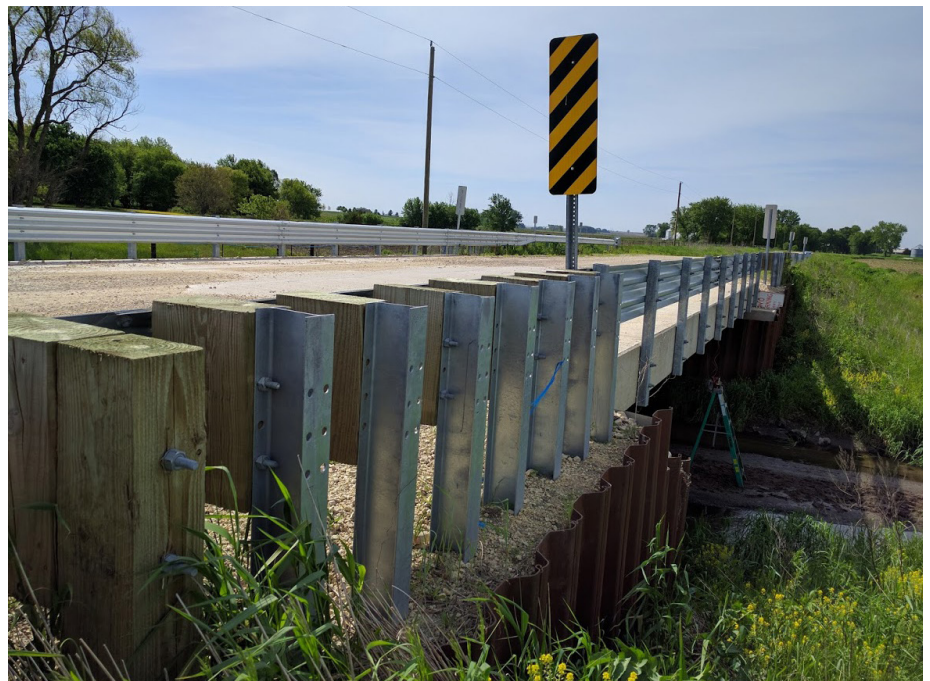
Buchanan County cast-on-site adjacent box beam bridge on Victor Avenue over Prairie Creek
