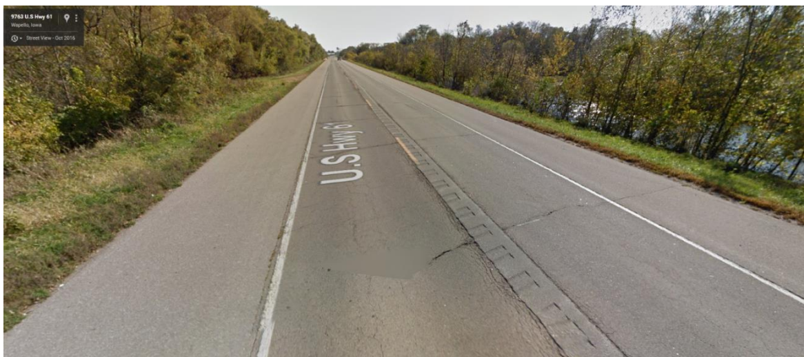
Figure 7. Centerline-only installation example
