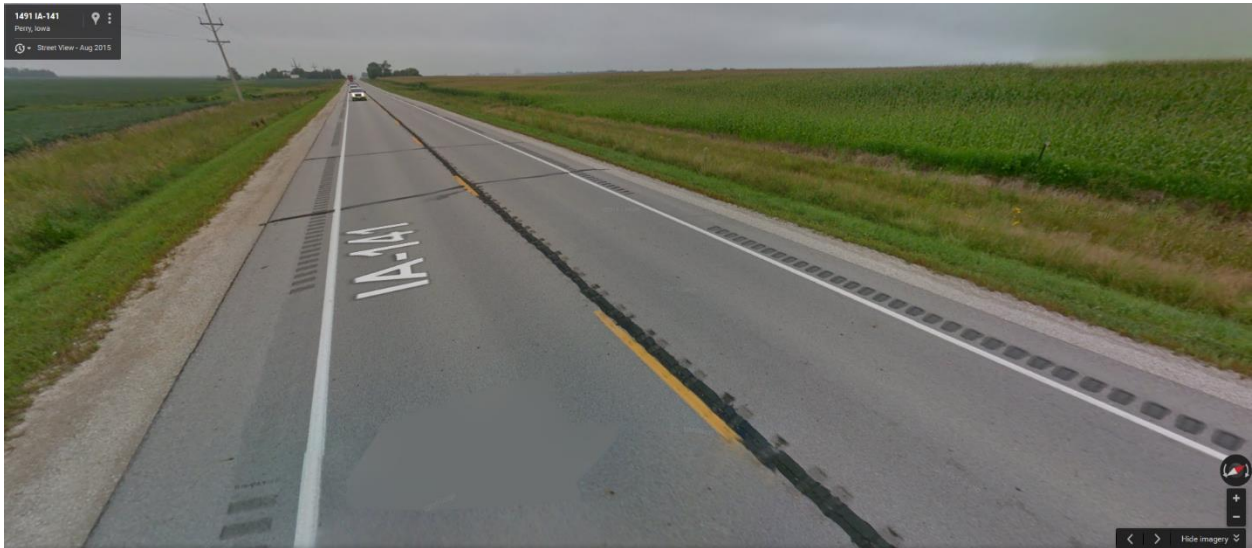
Figure 4. Continuous rumble strip installation with bicycle gaps
