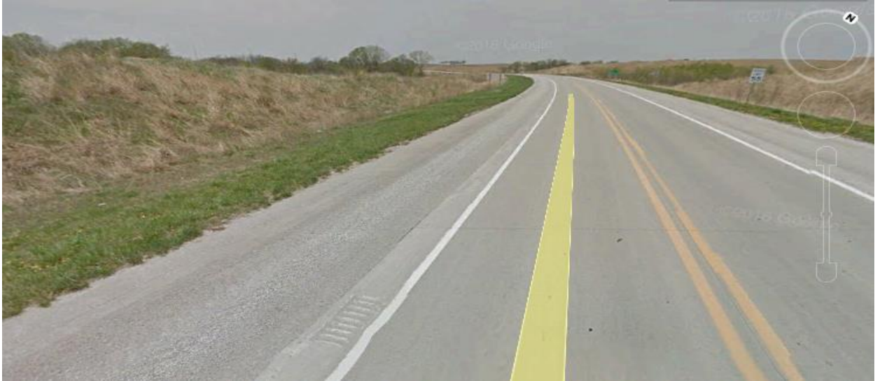
Figure 3. Intermittent rumble strip installation example
