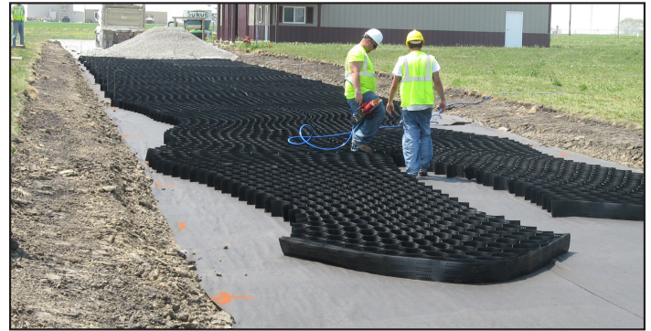
Figure 5. Installation of 6 in. geocell over non-woven geosynthetic layer placed on subgrade
