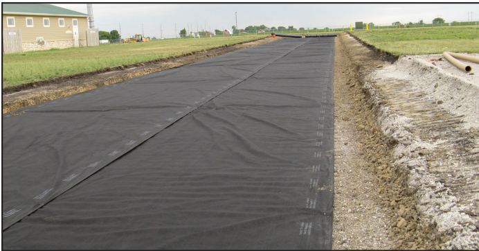
Figure 2. Non-woven geotextile placed on subgrade as a separation layer
