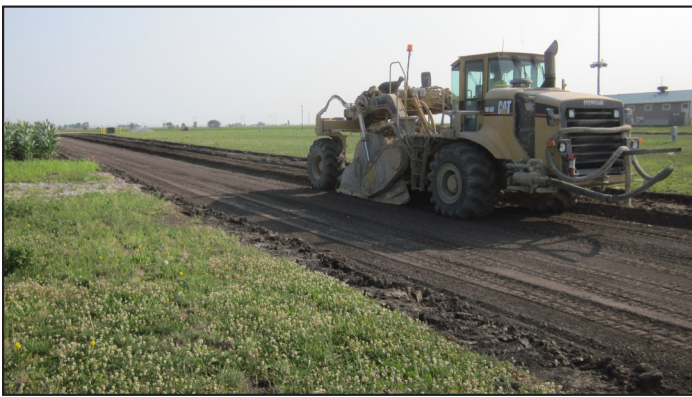
Figure 12. Mechanical stabilization
