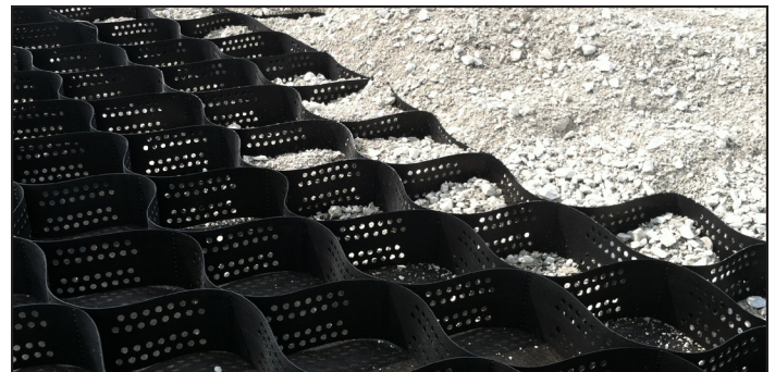
Figure 6. Close-up of 6 in. geocell over non-woven geosynthetic layer placed on subgrade
