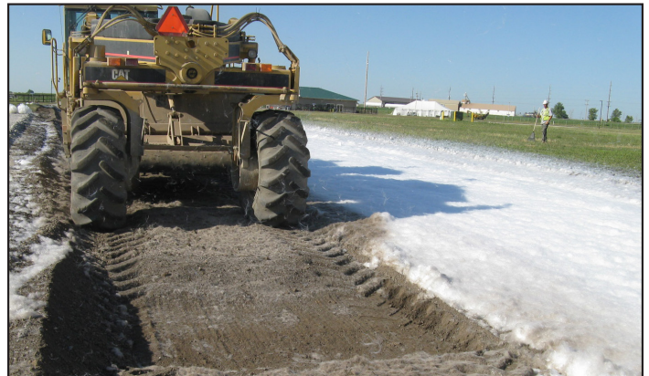
Figure 10. Mixing white MF-PP white fibers into recycled subbase
