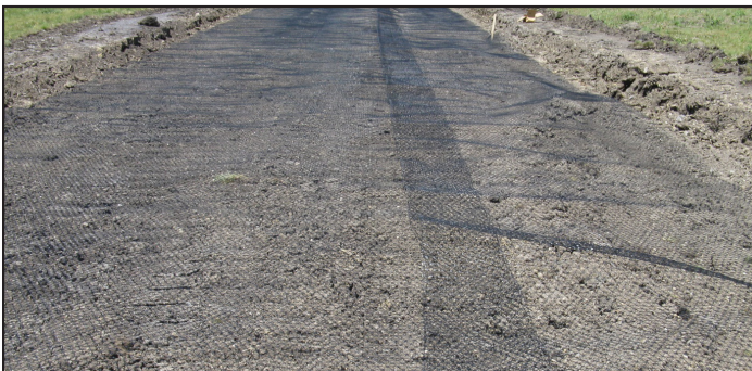
Figure 3. Triaxial geogrid placed at the interface of subgrade and limestone base layers
