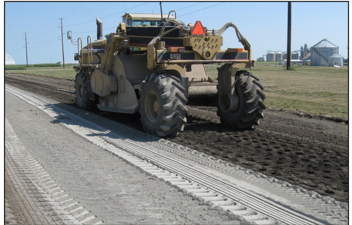
Figure 9. Soil reclaimer mixing PC with recycled subbase material
