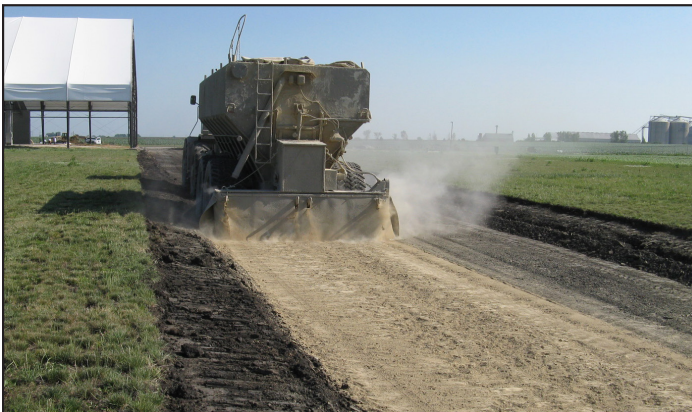
Figure 7. Distribution of FA on subgrade for mixing
