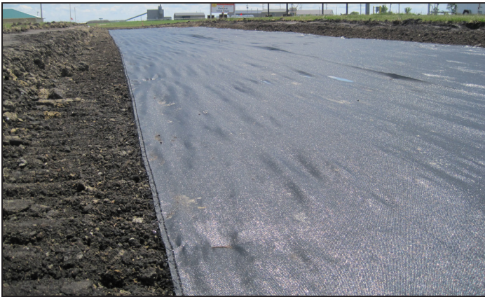
Figure 1. Woven geotextile placed on subgrade as a separation layer
