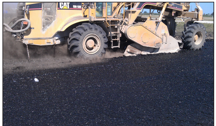
Figure 11. Mixing black PP fibers into recycled subbase
