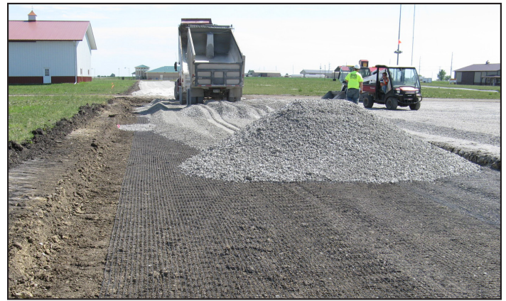
Figure 4. Biaxial geogrid placed at the interface of subgrade and limestone base layers
