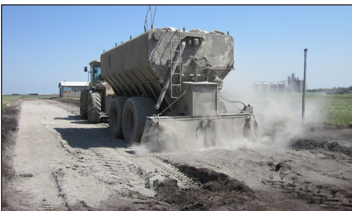
Figure 8. Distribution of PC on subgrade for mixing
