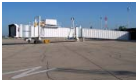
The new jet bridge at the Dubuque Regional Airport.
