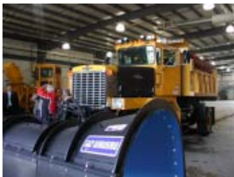
New snow removal equipment storage and maintenance facility at the Sioux Gateway Airport.
