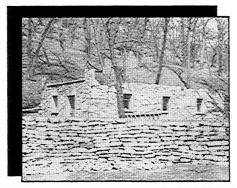
Hatchery building, completed in 1939, of natural rock laid edgewise in concrete to blend with rock surroundings of Big Spring.
