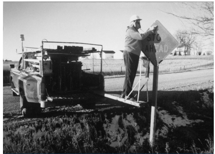
Sign replacement on a rural road in Iowa
