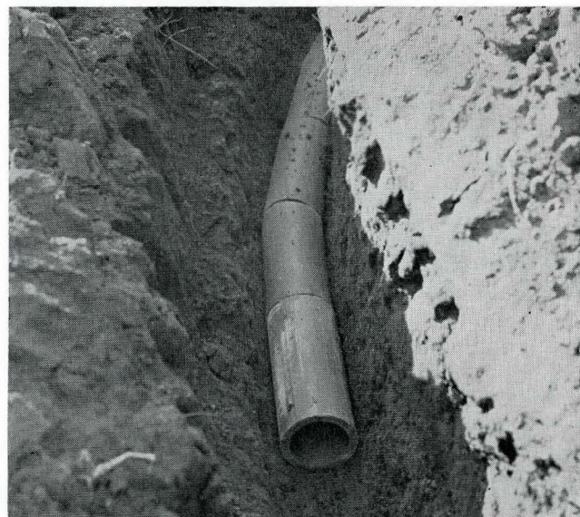
Fig. 15. When soil is too wet for the healthy growth of crops, the excess water can often be removed from the land by the use of tile drains.
