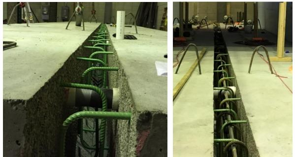
Two box beams placed side-by-side (left); Joint reinforcement with longitudinal bars and stirrups (right)
