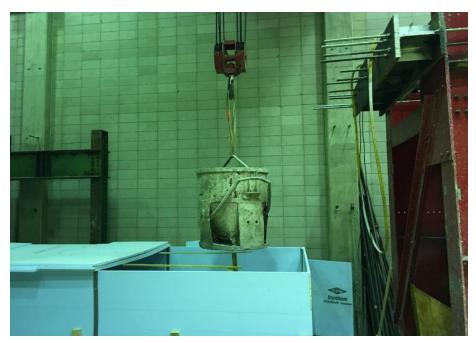
**Figure 30. Pouring joint concrete**
