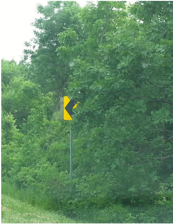
Figure 14. Chevron obstructed by tree branches
