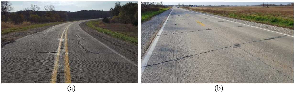
Figure 76. Joint deterioration on Dallas County F-31 at sections (a) west of Minburn and (b) west of Granger (November 2016)
