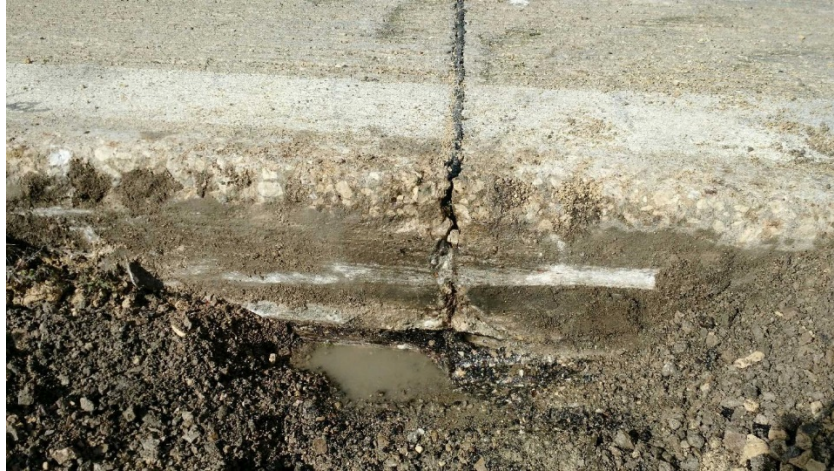
Figure A.37. Activated transverse joint in slab adjacent to blow-up on Linn County North 10th Street
