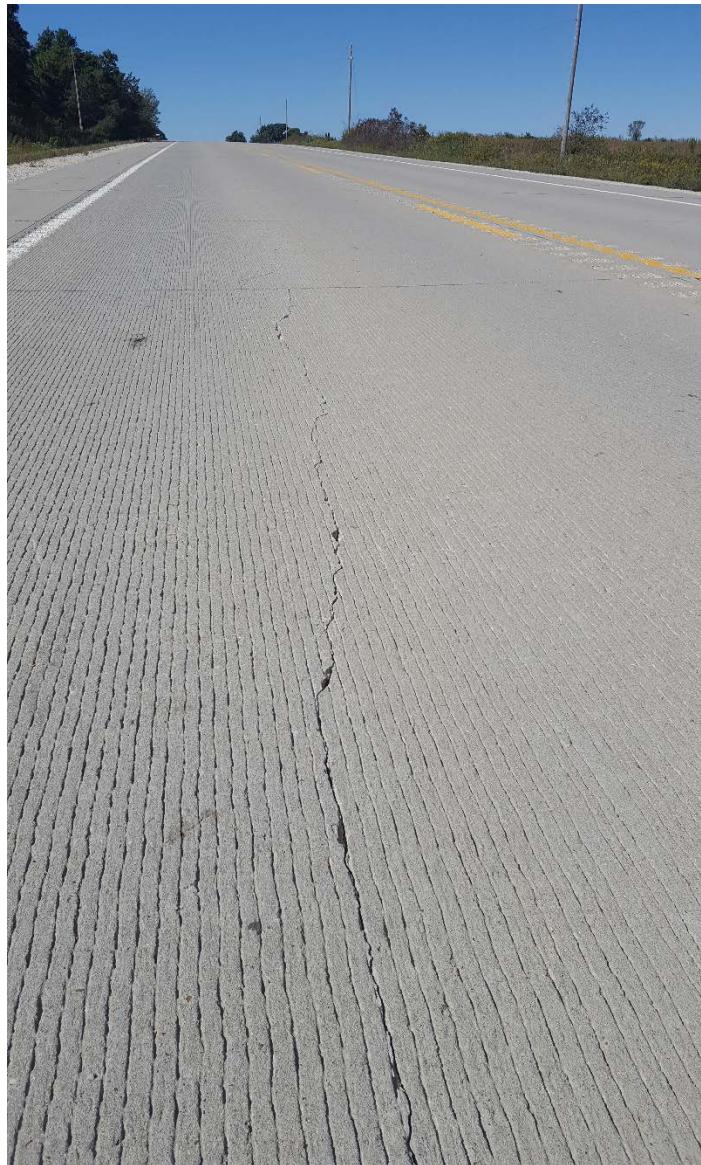
Figure A.2. Longitudinal cracking in Buchanan County D-22, September 2016
