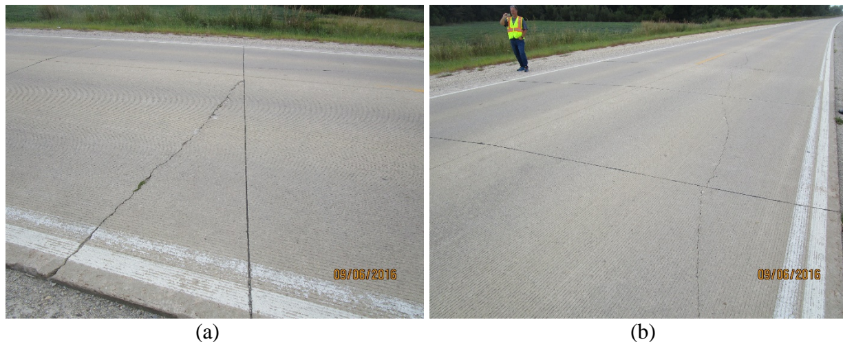
Figure 79. (a) Longitudinal and (b) corner cracking on Blairs Ferry Road (September 2016)
