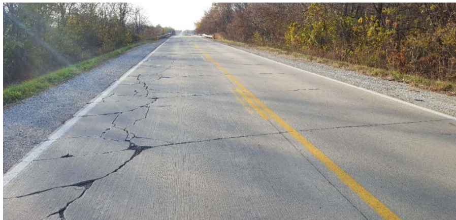
Figure A.19. Cracking at slab edge approaching creek crossing on Dallas County F-31 west of Granger, November 2016
