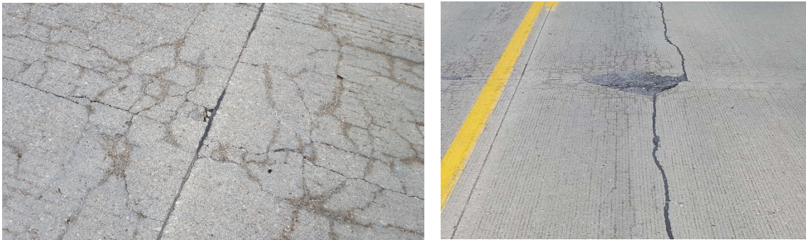
Figure A.48. Materials-related distresses on Pottawattamie County L-66, November 2016
