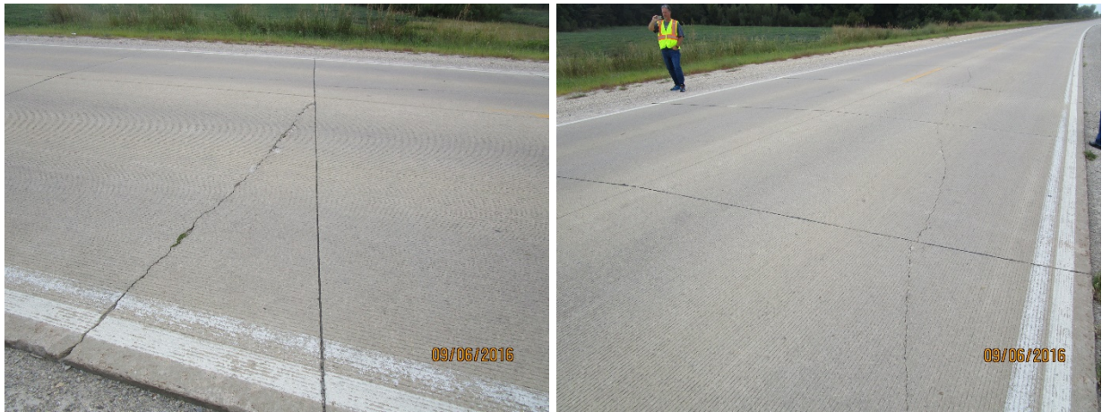
Figure A.32. Longitudinal and corner cracking on Linn County Blairs Ferry Road, September 2016
