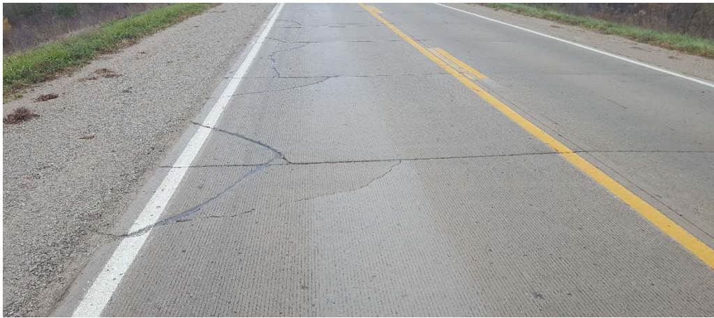
Figure 80. Cracking on Dallas County F-90 (November 2016)
