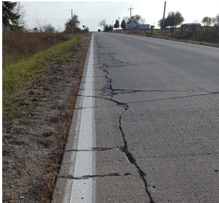
Figure A.30. Loss of support along pavement edge on Dallas County R-22, November 2016
