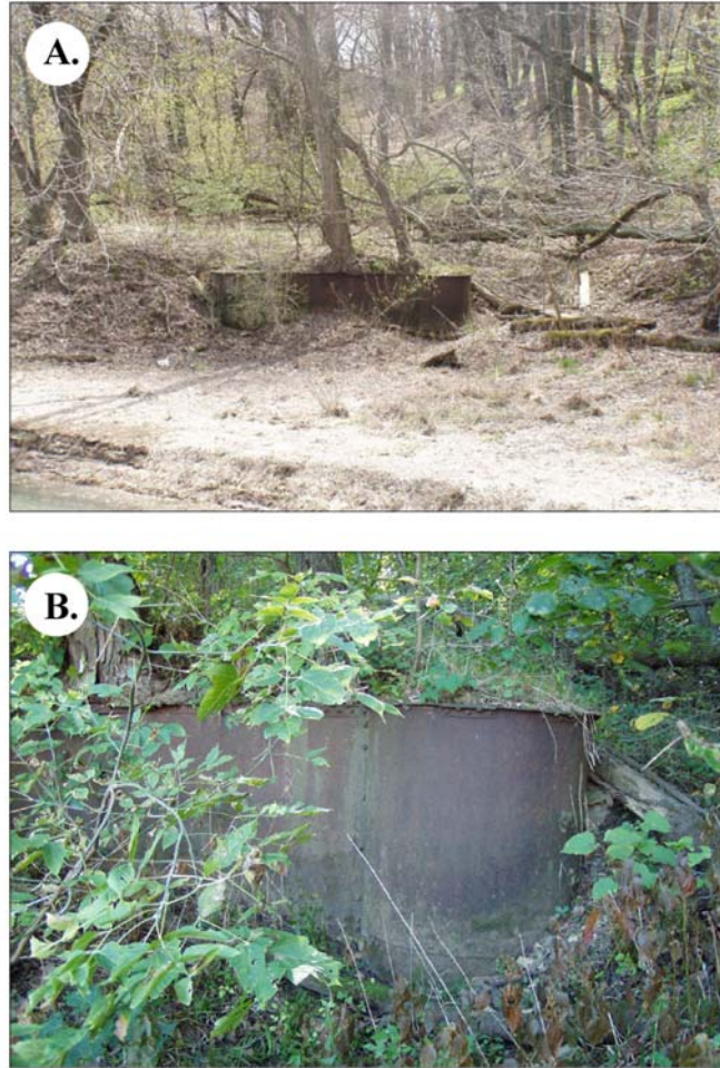
Figure 18. Photographs of the cast-iron bridge footings located at the north end of site 13JK267. A.) Photo showing bridge footings from the north Mill Creek bank, facing south. B.) Photo showing close-up of the cement-filled, riveted, cast-iron bridge footings along the south bank of Mill Creek.
