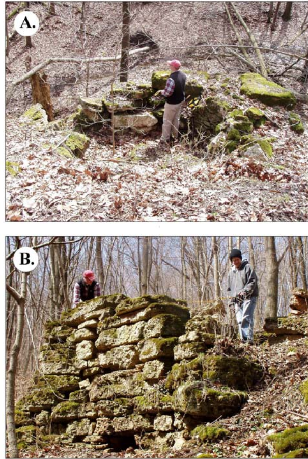
Figure 14. Photograph of site 13JK604. A.) Looking down on the lime kiln showing crew member for scale facing south, B.) View looking up at kiln showing crew members for scale, the partial north wall collapse, and the stoking door facing west south-west.
