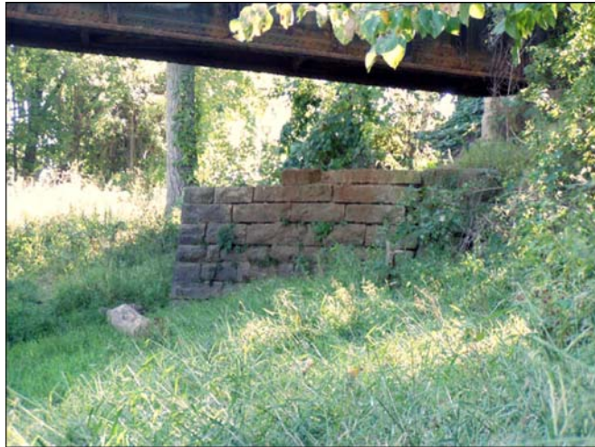
Figure 20. Photographs railroad bridge footings left from the 1896 flood beneath extant bridge.
