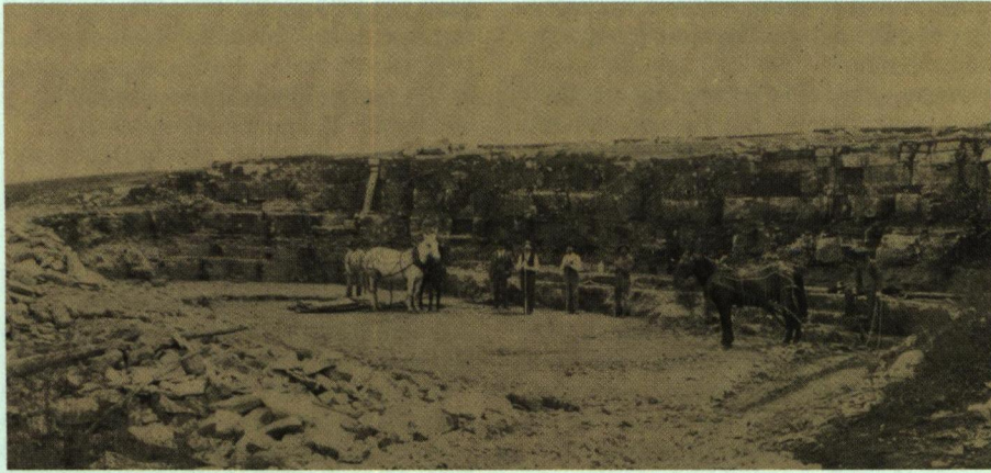
Above: Men with pry bars and horse-drawn skids for hauling stone work the layers of lithographic limestone at Quarry No. 1 in Lithograph City near the Floyd-Mitchell county line about 1914. Below: Rough slabs of quarried lithographic stone sit outside the cutting plant where they are to be shaped and sanded before shipment for use in lithograph printing. (From Webster, 1915)
