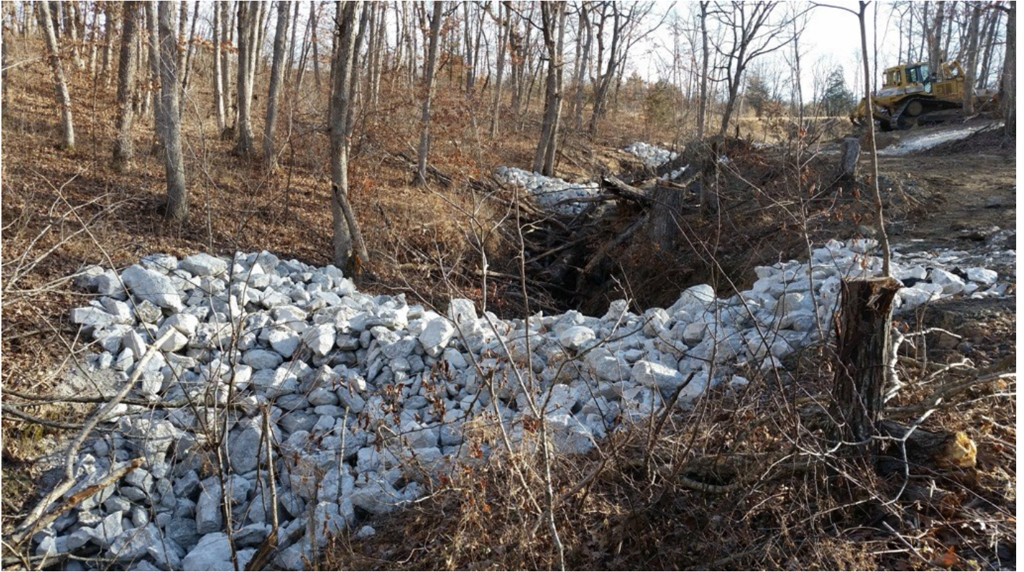
Rock check dams installed on State Owned Land as part of Lake Miami Watershed Project 1325-012
