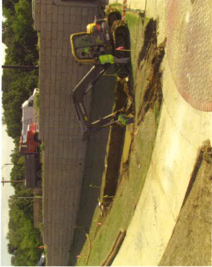
Excavation of one of the two southern biocells after proper stabilization of the surrounding area.
